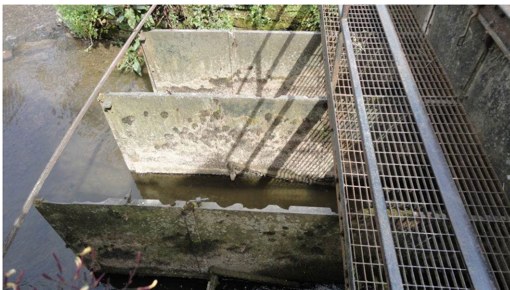
Photo 5: The eel trap divider plates, looking N
