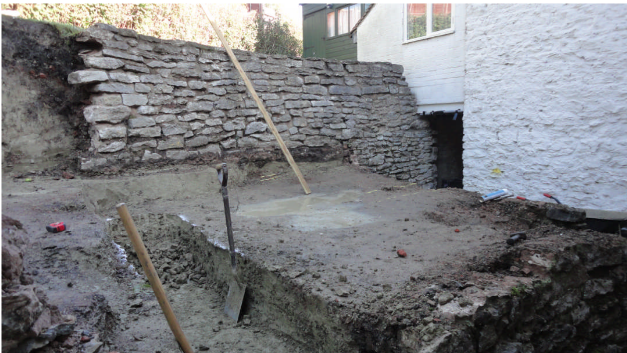
Photo 2: The development site; looking NE
