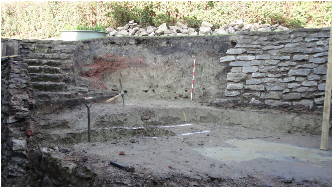
Photo 1: The development site showing the deposits behind the patio terrace wall; looking NW; scale bar 1m
