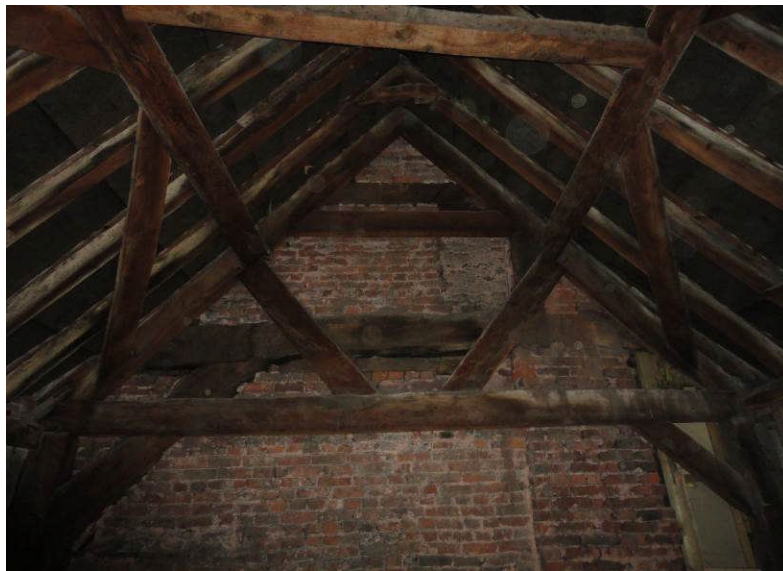
Photo 13: The truss in the S end wall above bedroom 5, looking S
