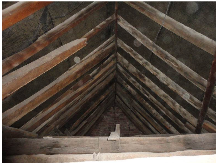
Photo 10: The roof-space above bedroom 1, looking N
