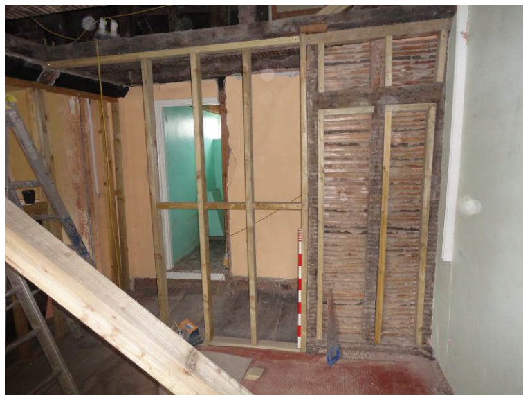
Photo 11: The location of the new stairwell in bedroom 4, looking SW
