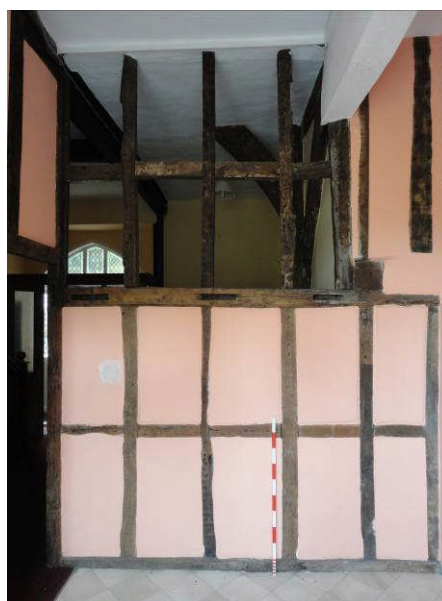
Photo 3: The hall partition looking E; scale bar 1m
