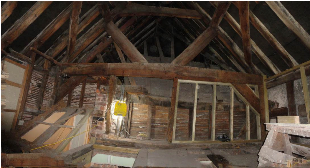
Photo 12: The roof-space above bedrooms 4 & 5, looking N
