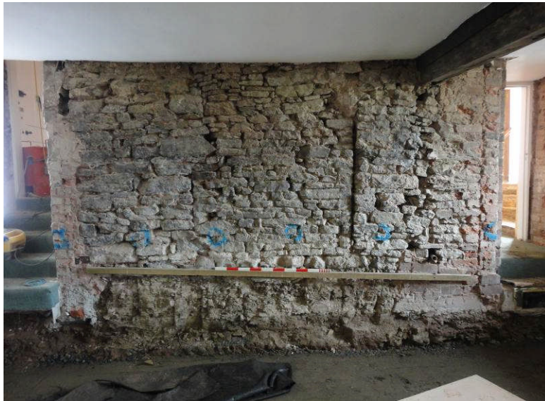
Photo 5: The chimney base in the undercroft, looking S; scale bar 1m
