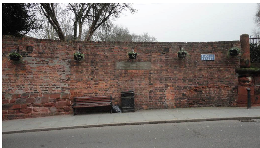
Photo 10: The location of the entrance to the 20 th century air raid shelter (site 12) on Castle Gates, looking E
