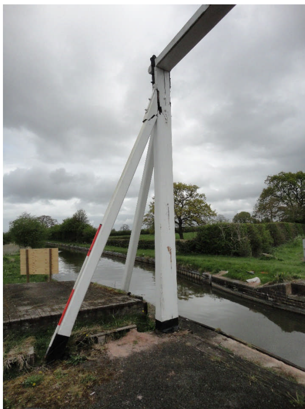
Photo 8: Portal frame, showing crack on N frame looking NE, scale bar 2m
