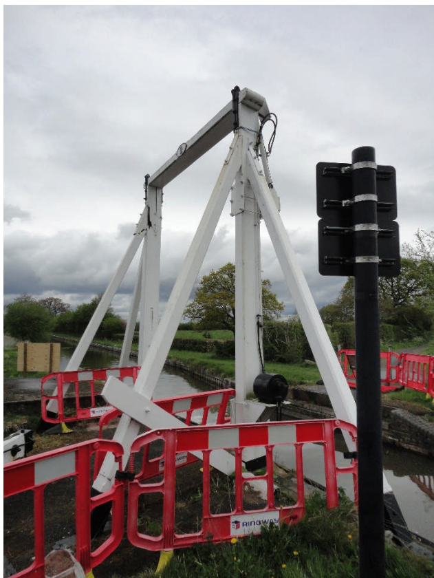
Photo 7: Portal frame, showing lifting gear, looking NE
