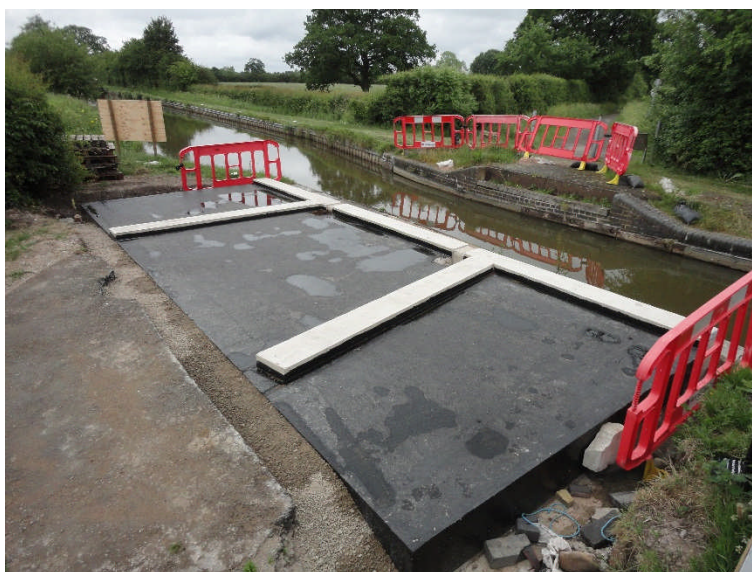
Photo 12: The new portal frame base, looking NE
