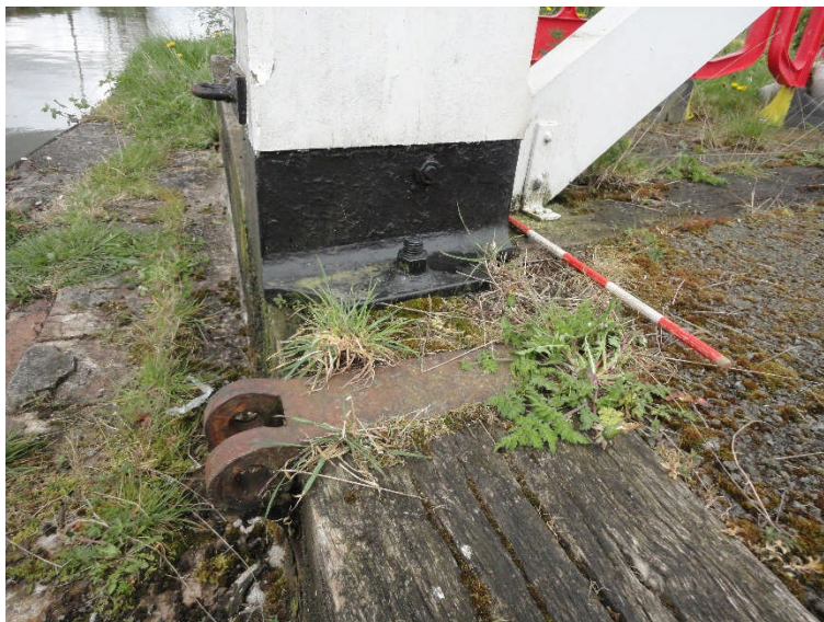
Photo 10: The portal frame base plate (S) and deck hinge, looking S, scale bar 0.5m
