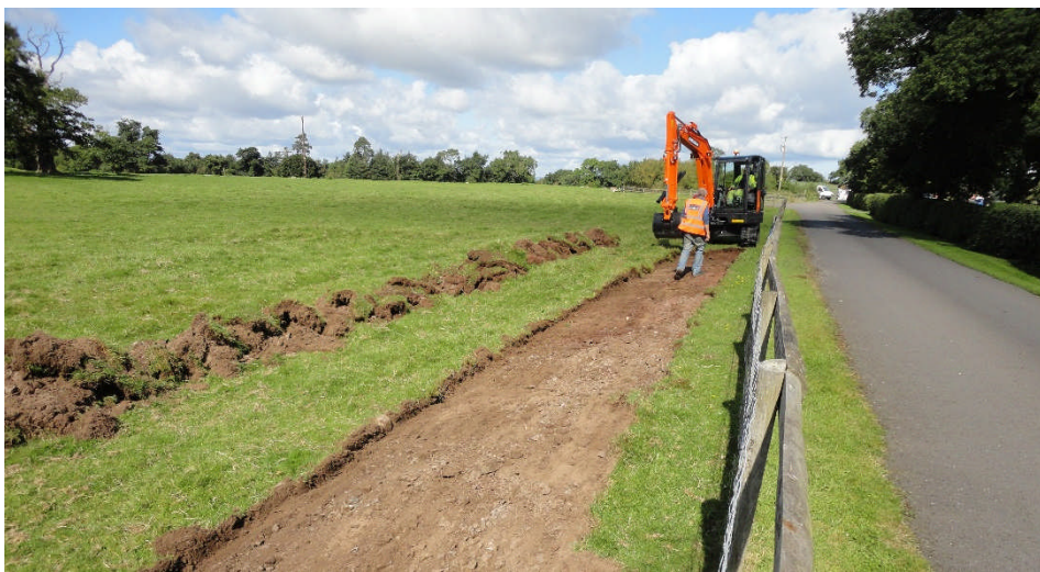
Photo 2: The topsoil strip, looking NW
