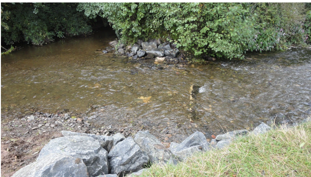
Photo 3: The completed work, looking NW
