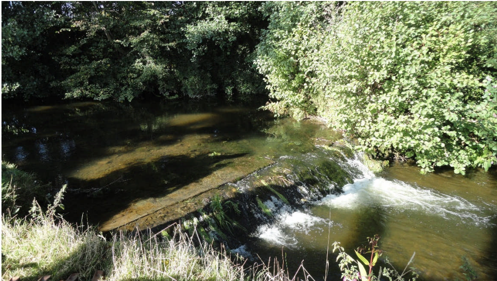
Photo 1: The weir, immediately before the work, looking W
