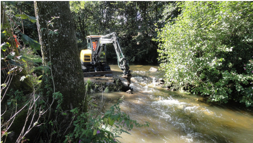
Photo 2: The weir reduction underway, looking SW
