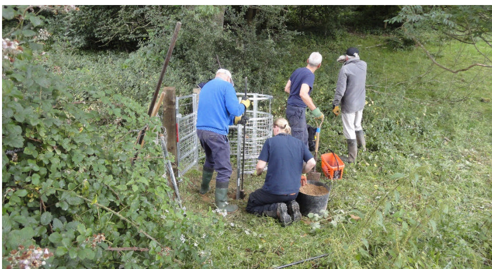
Photo 3: The new gate installed, looking S
