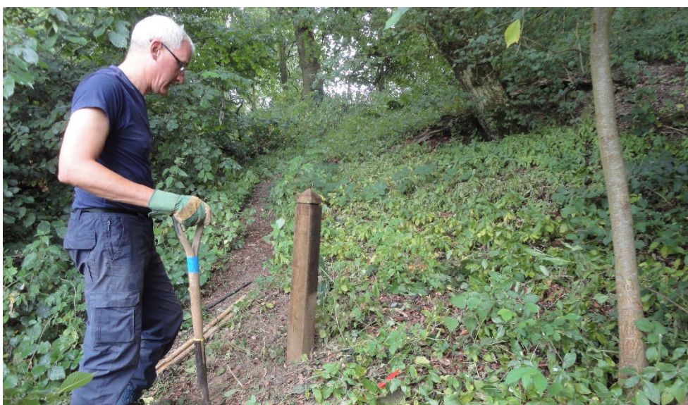
Photo 6: The new waymark post, looking S
