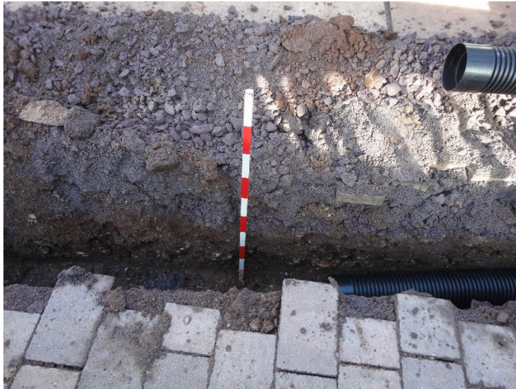
Photo 2: The pit (6) looking SW; scale bar 1m
