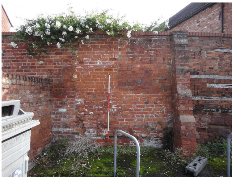
Photo 4: The east wall, N section, looking E; scale bar 2m
