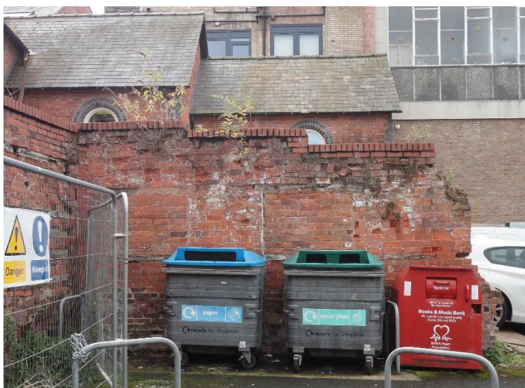
Photo 5: The south wall, looking S
