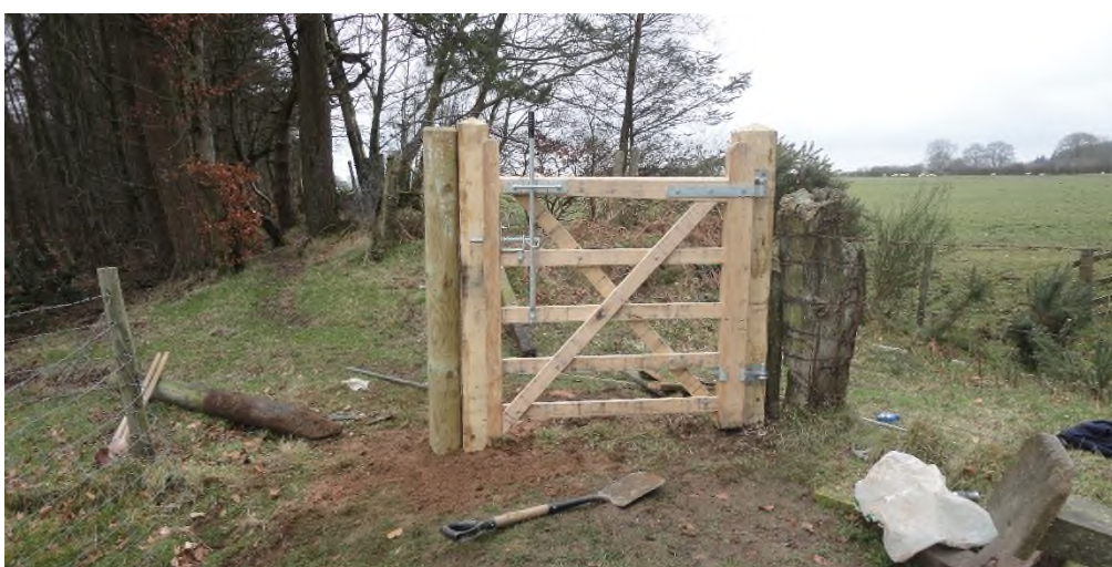
Photo 12: The new gate at Selattyn Lodge A, looking S
