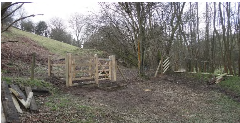
Photo 3: The completed gate at Lower Mount C, looking SW
