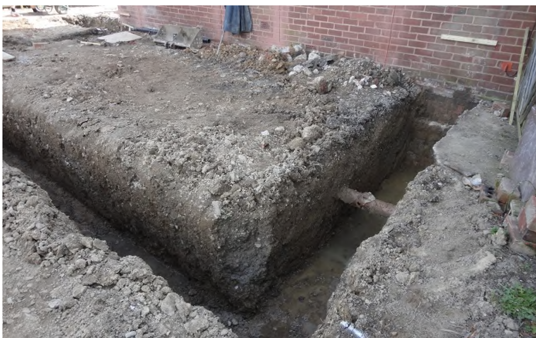
Photo 3: The foundation trenches, looking SE
