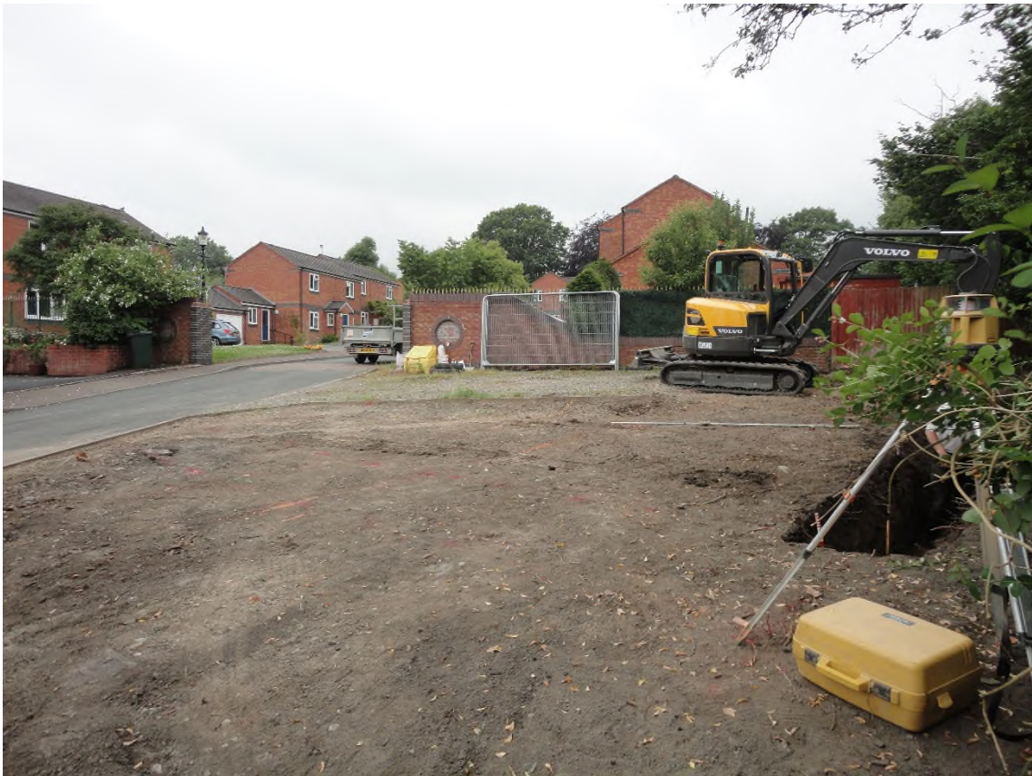
Photo 1: The development site, looking W
