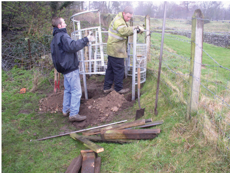
Photo 2: Gate B, looking E
