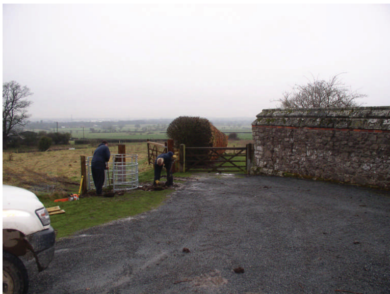
Photo 3: Gate D, looking NW
