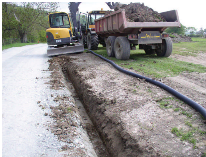
Photo 4: Excavating the french drain alongside the new track
