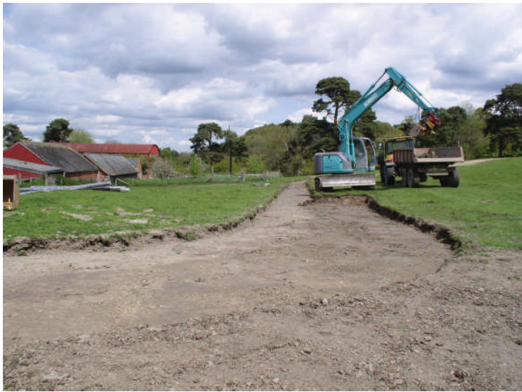
Photo 1: The excavation for the new track, looking east
