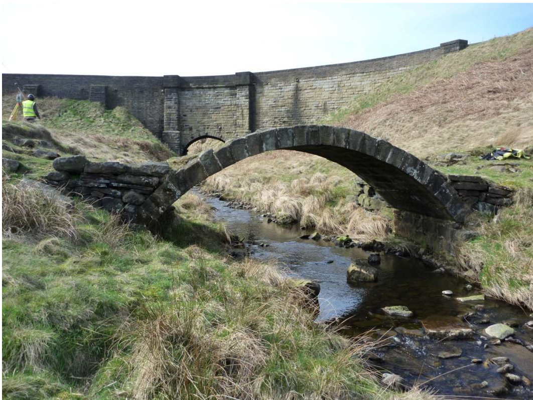
Plate 2: View of the bridge, looking southwest
