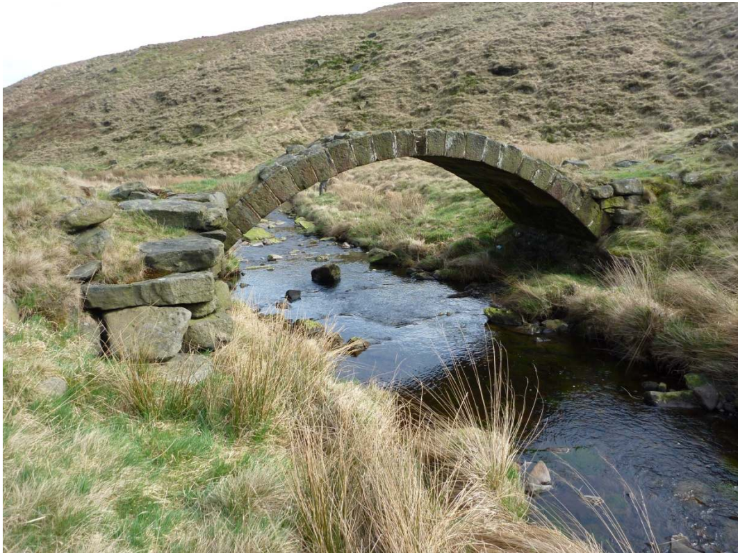
Plate 1: View of the bridge, looking northeast
