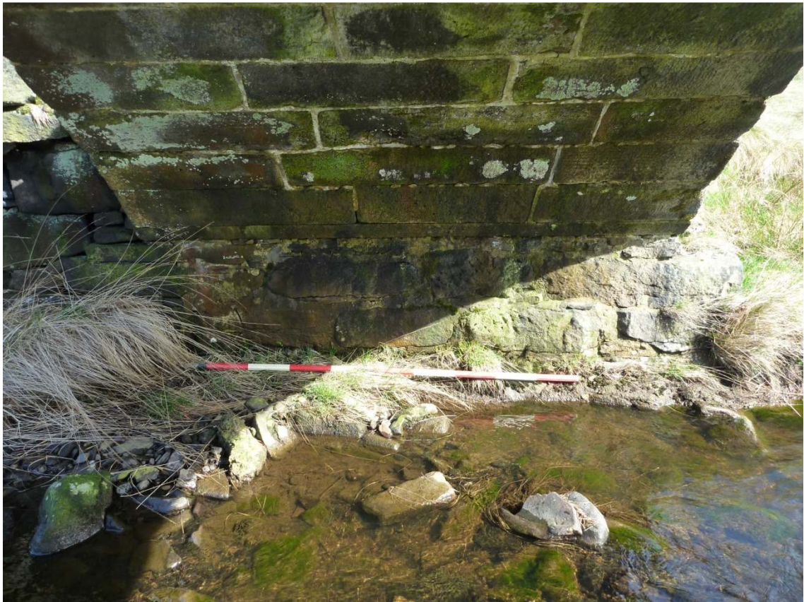
Plate 5: Inner face of north side abutment, looking north
