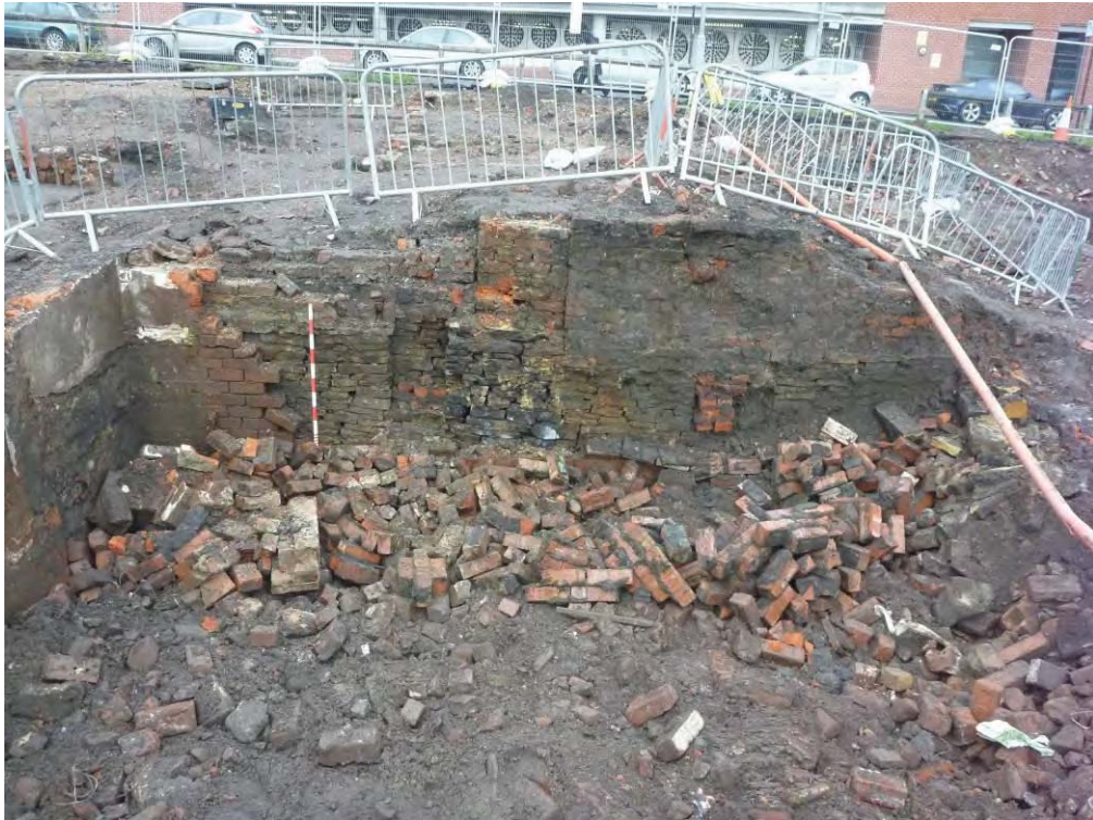
Plate 14: Cellar D, after removal of wall 1092, viewed from the south-west
