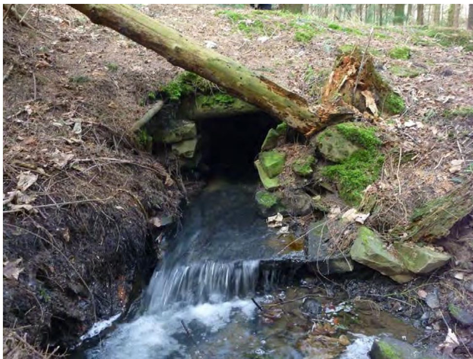
Plate 17: Unmortared sandstone culvert with stone flag base
