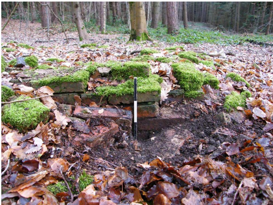
Plate 53: Detail of brick structure (Survey Feature 45)
