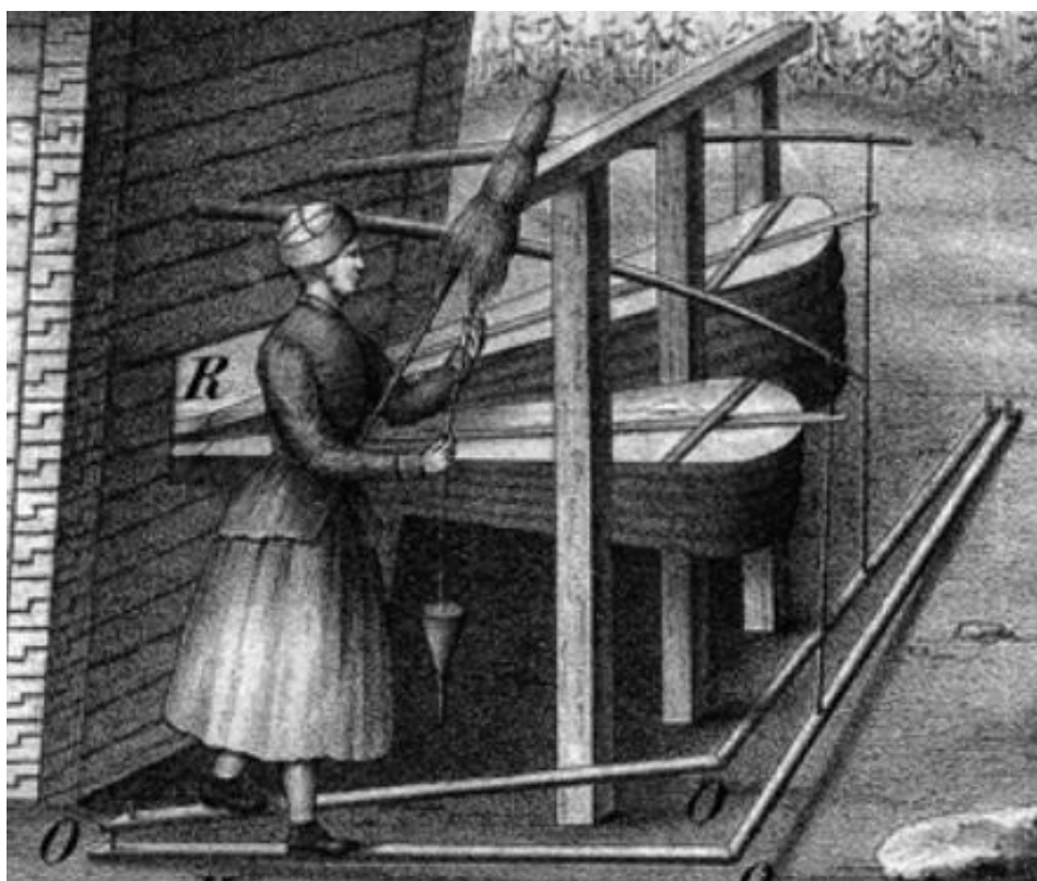
Plate 6: Foot-operated bloomery bellows
