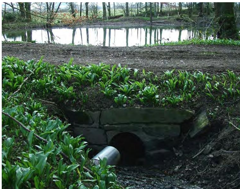
Plate 11: Stream culverted beneath present-day track
