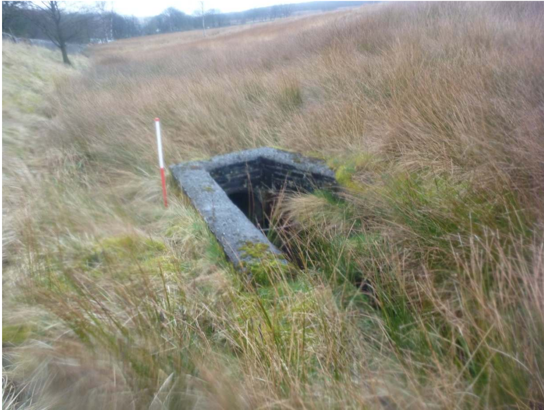
Plate 5: Brick and concrete culvert 68511, viewed facing north
