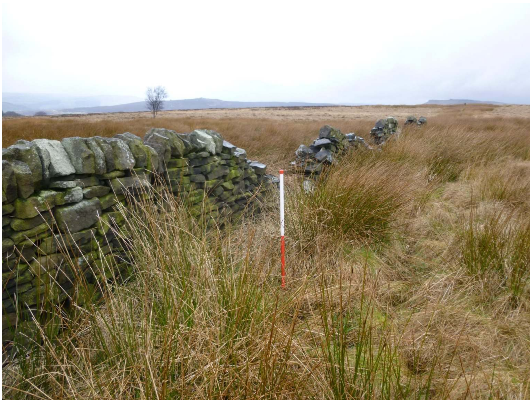
Plate 6: Field boundary wall 68527, viewed facing west
