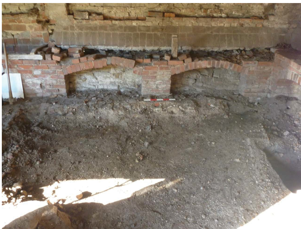
Plate 4: Area 2 following excavation. Viewed facing north, 50cm scale
