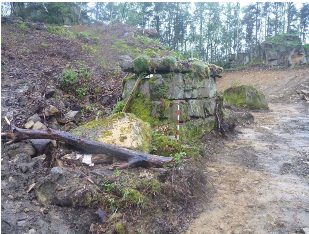
Plate 3: South and east faces of structure WS12, viewed facing north
