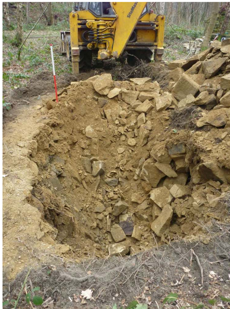
Plate 6: Sondage through fractured sandstone blocks 104, viewed facing southeast
