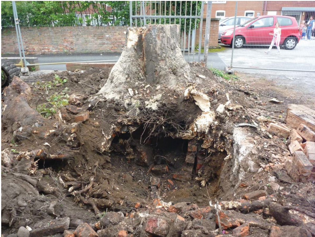
Plate 1: Working shot of tree root and manhole during removal
