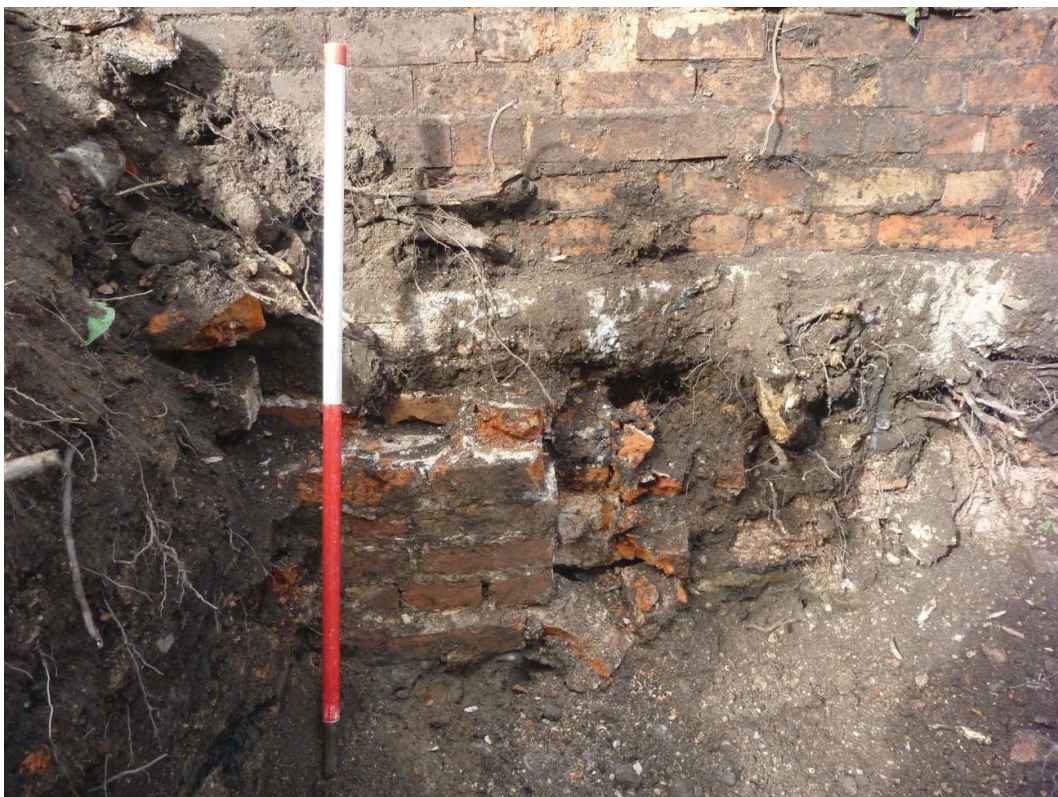
Plate 2: Structure [1003] below modern structure [1001]. Viewed facing west, 1m scale.
