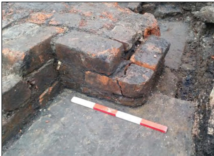
Plate 12. Detail of additional outer skin 117, added to wall 107. Scale 0.40m. Looking north-east
