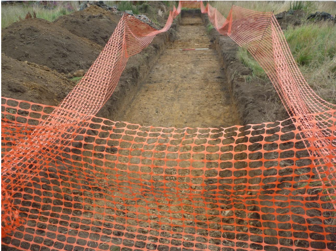
Plate 5: Trench 3, looking north-east. Scale 1m.
