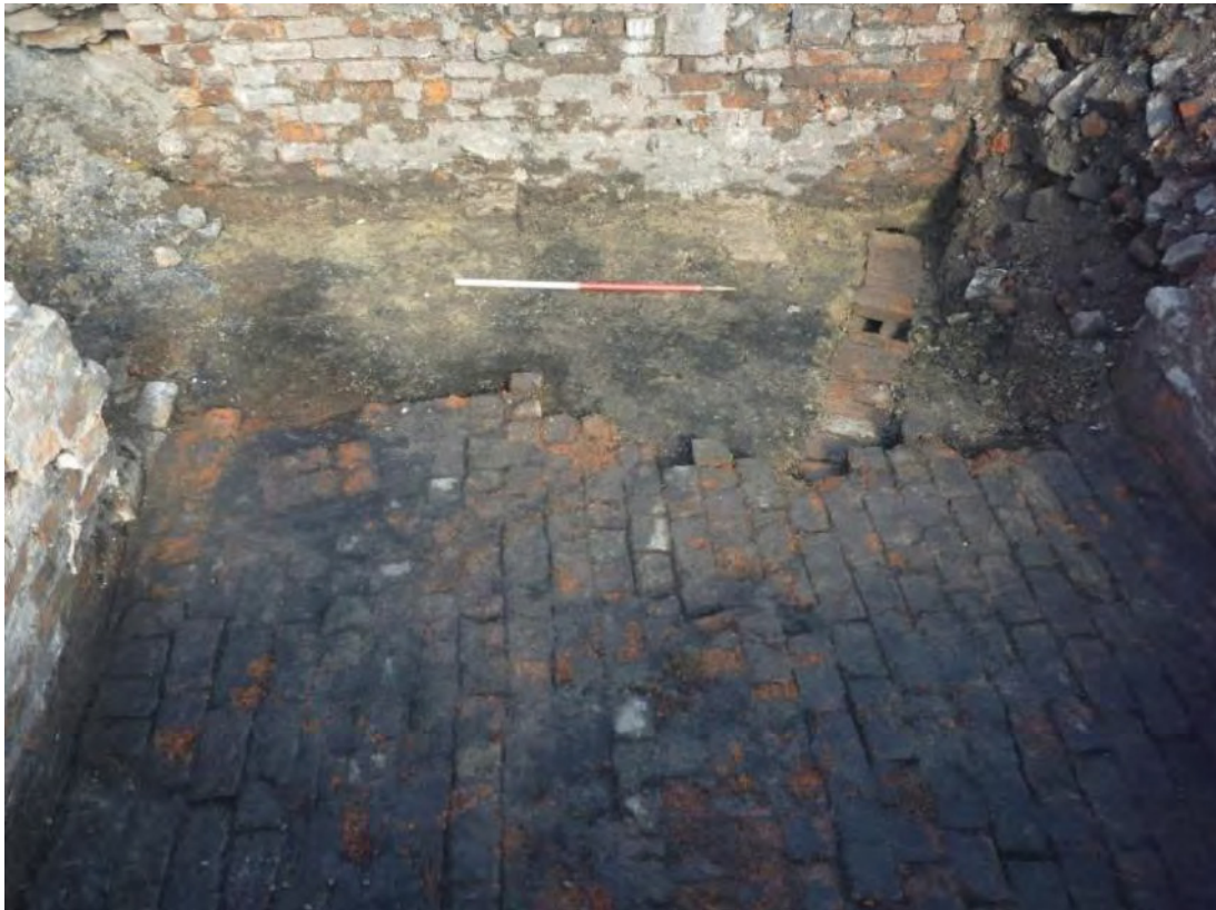
Plate 11: Truncation in Cellar 2, showing damage to the brick floor (162) and walls (103, 108, 119 and 192). Drain (163) and possible fireplace (164 and 165) can also be observed. Looking north-west. Scale 1m.
