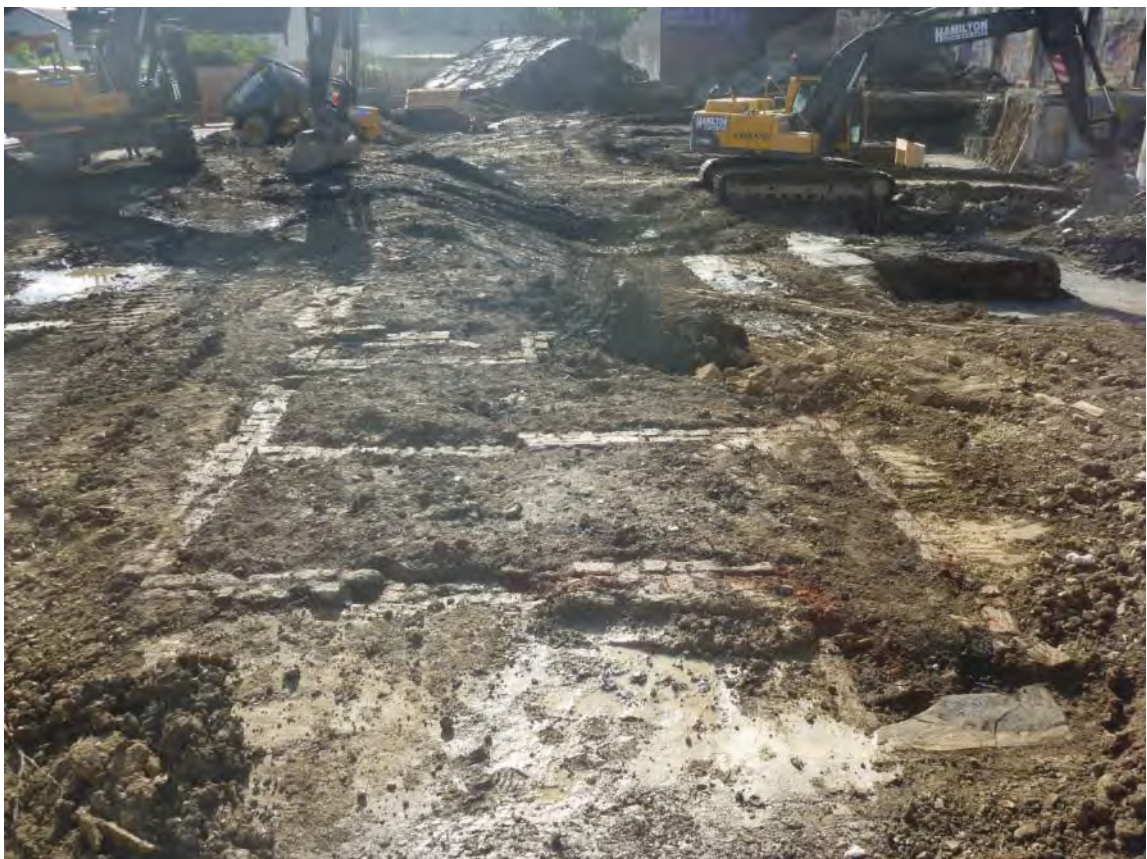
Plate 34: Cellars 7 and 8, looking south-east.
