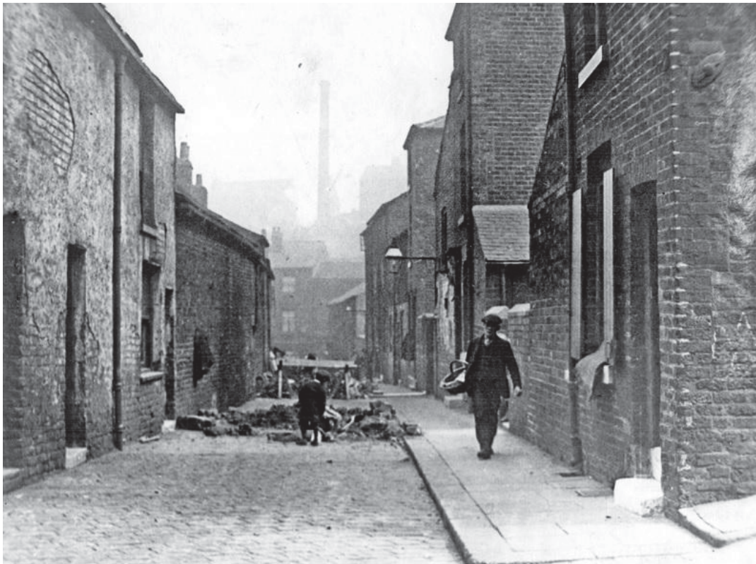
Plate 1: Road works in Daisy Walk, taken from the entrance to Court No. 9 (right) looking towards Upper Allen Street. ©Sheffield City Council. Picture Sheffield Reference s14815
