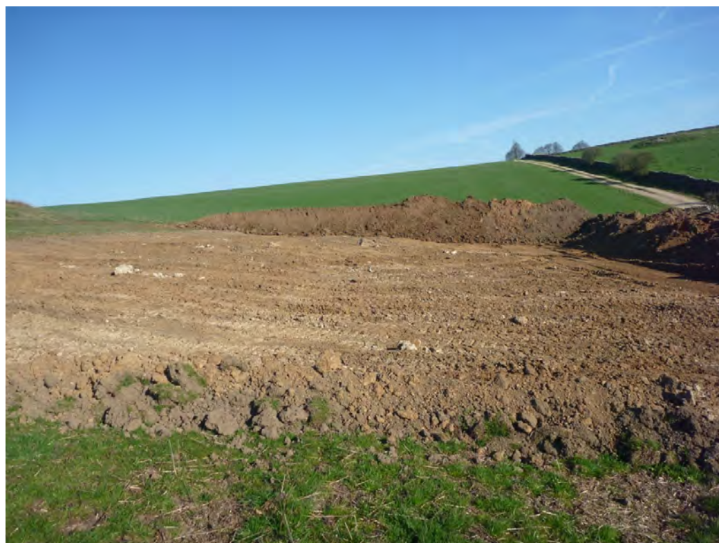
Plate 2: Soil strip at the location of Turbine 1. Facing north-west.
