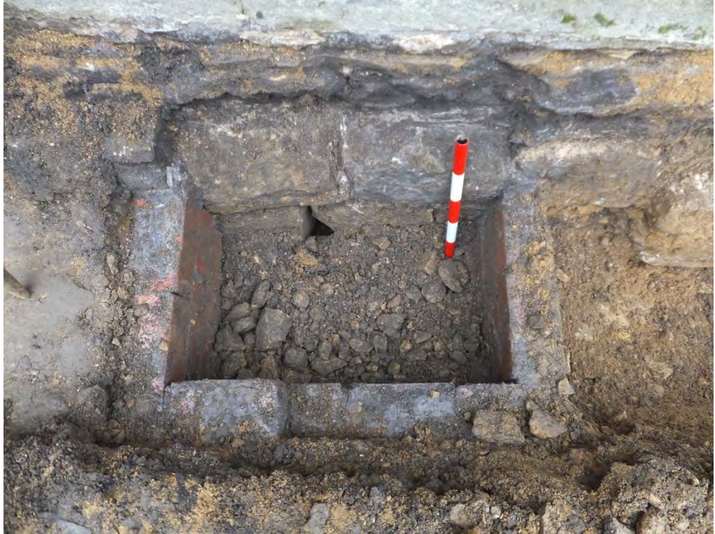
Plate 1: Duct 1003 & 1009 on the eastern side of the trench. Looking west, scale 0.5m.
