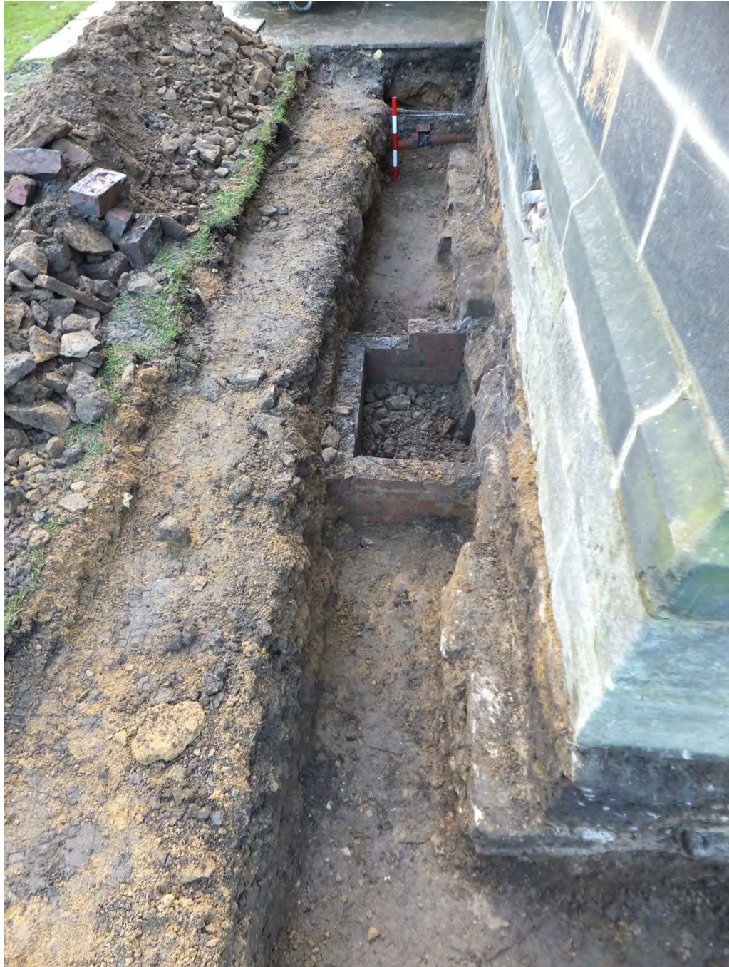
Plate 3: East side of the trench, looking south, showing duct 1003 & 1009. Scale 0.5m.
