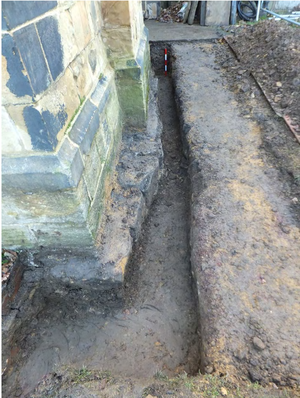
Plate 2: West side of the trench, looking south. Scale 0.5m.
