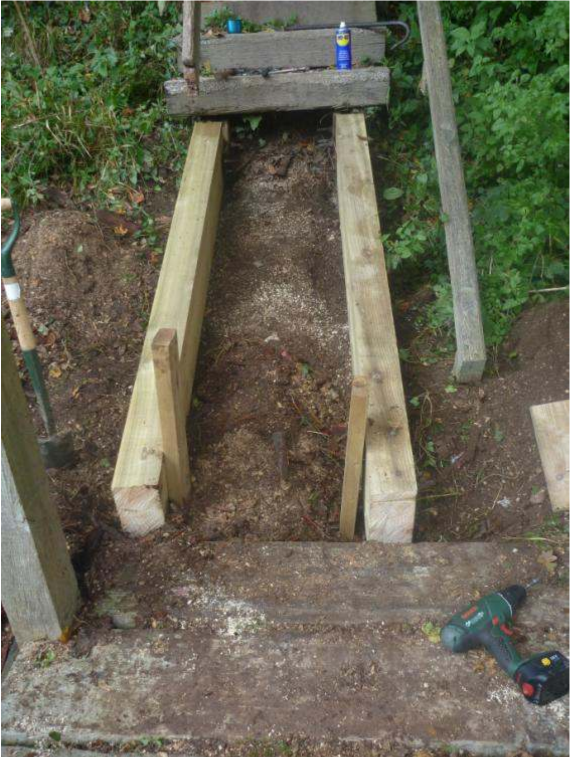
Plate 2: Replacement beams in place, facing north
