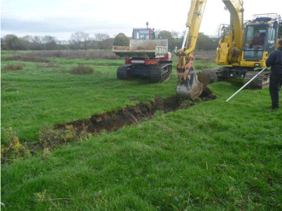
Plate 7: Working shot of the initial excavation of the connector ditch.
