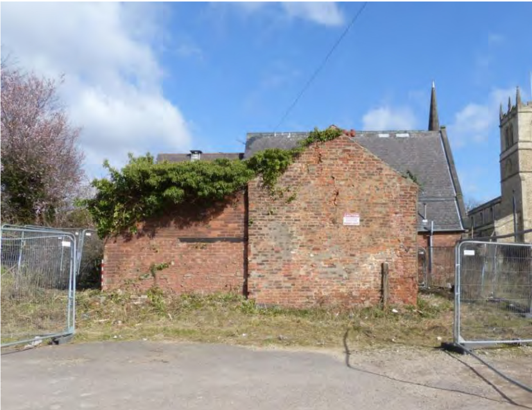
Plate 1: Western elevation of the building, with the earliest phase (southern half) on the left, and the more recent phase (northern half) on the right. Scale 1m.
