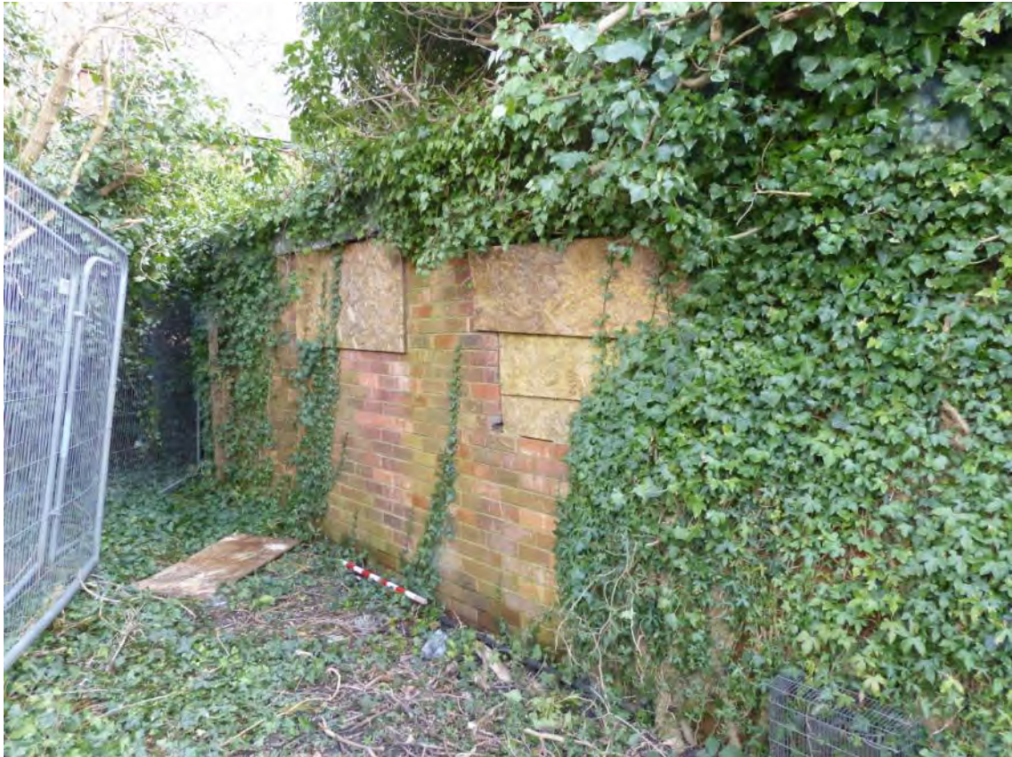
Plate 5: Northern elevation of the building. Scale 1m.
