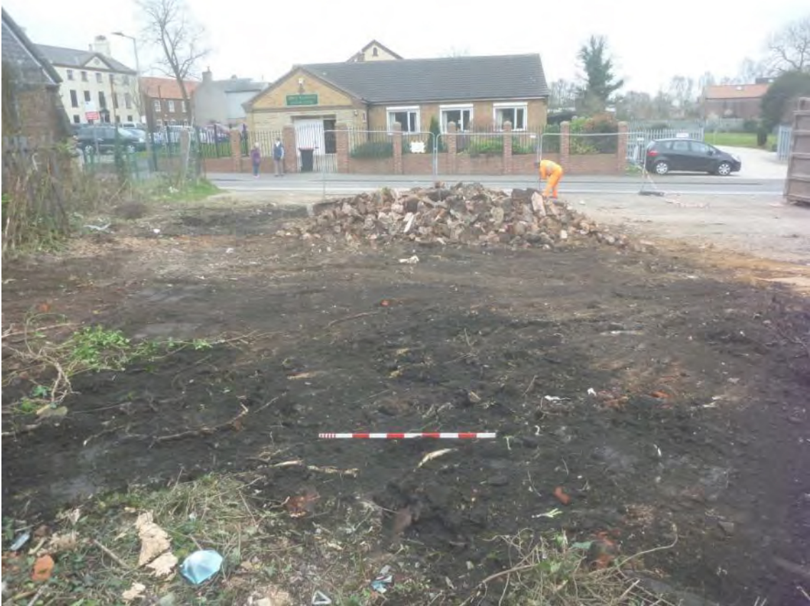
Plate 17: Demolition complete. Looking south-east, scale 1m.
