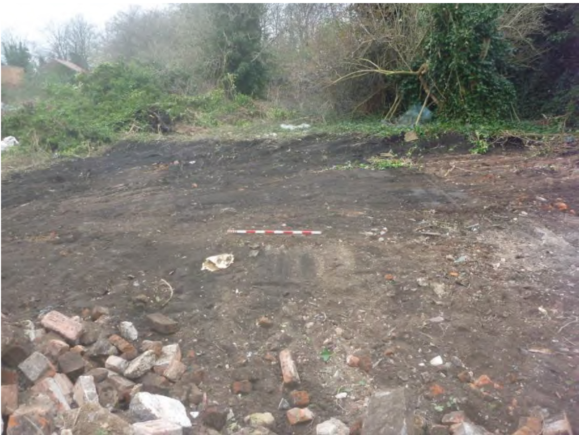
Plate 18: Demolition complete. Looking north-west, scale 1m.
