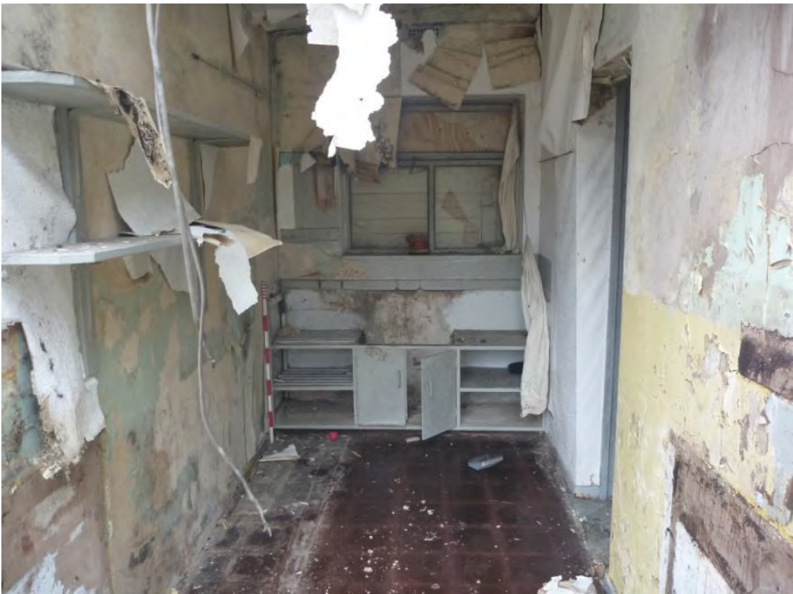
Plate 14: Kitchen (Room 3) in the northern half of the building. Looking north-east. Scale 1m.
