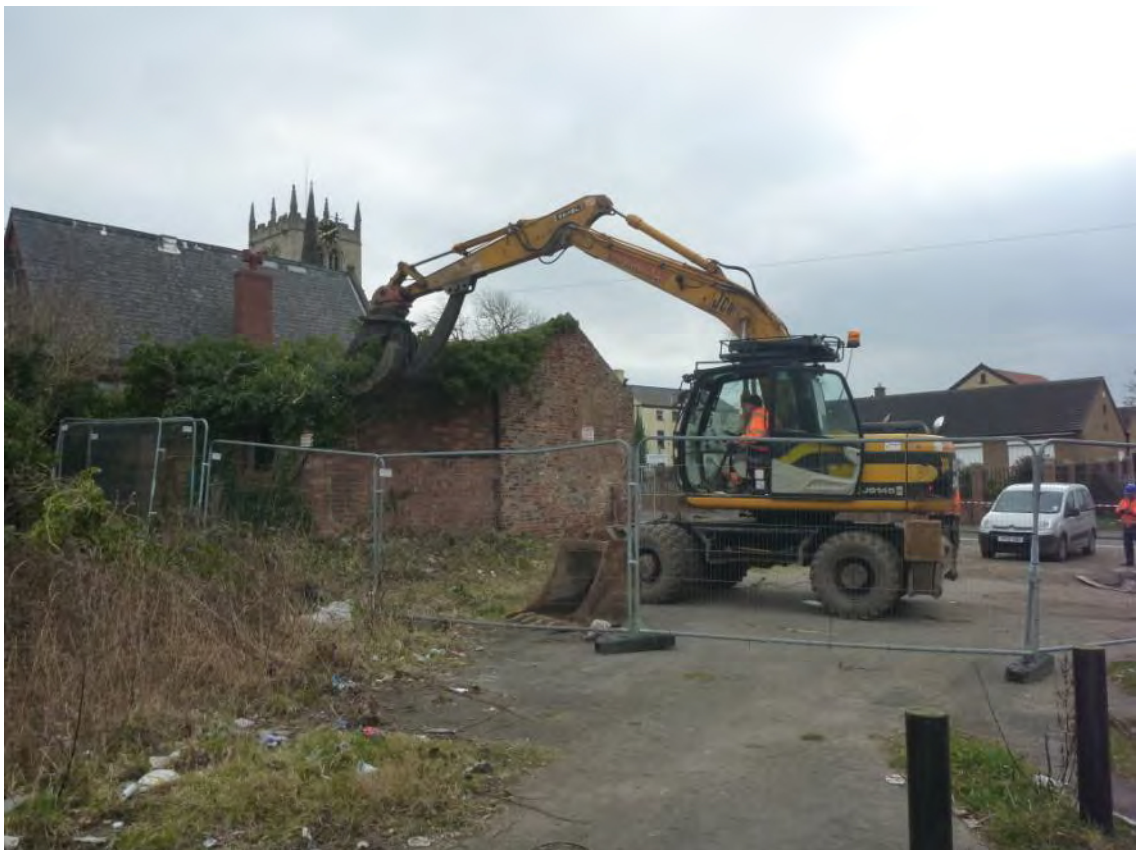
Plate 6: Working shot of demolition of the building. Looking south-east
