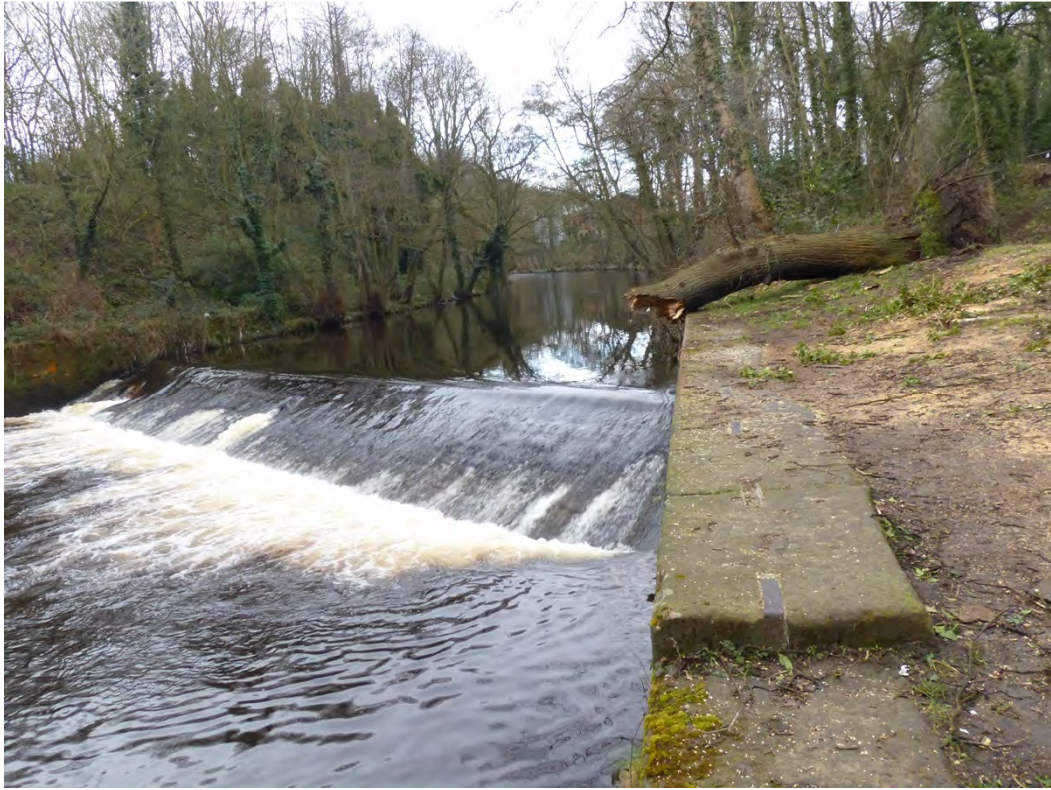
Plate 13: East bank revetment wall constructed from large blocks
