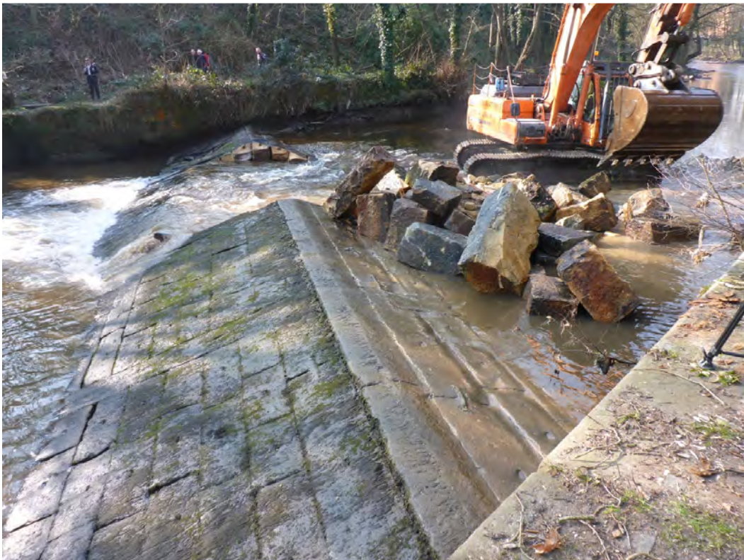
Plate 2: Cutting through the weir
