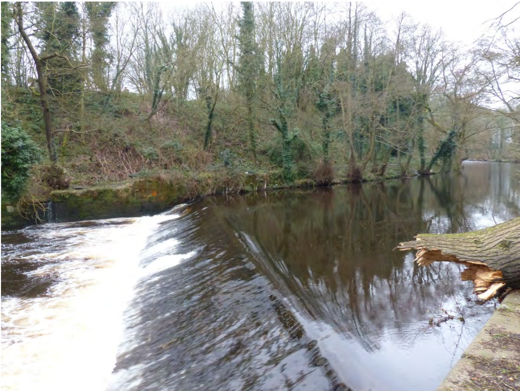
Plate 6 View of weir prior to works showing former river levels
