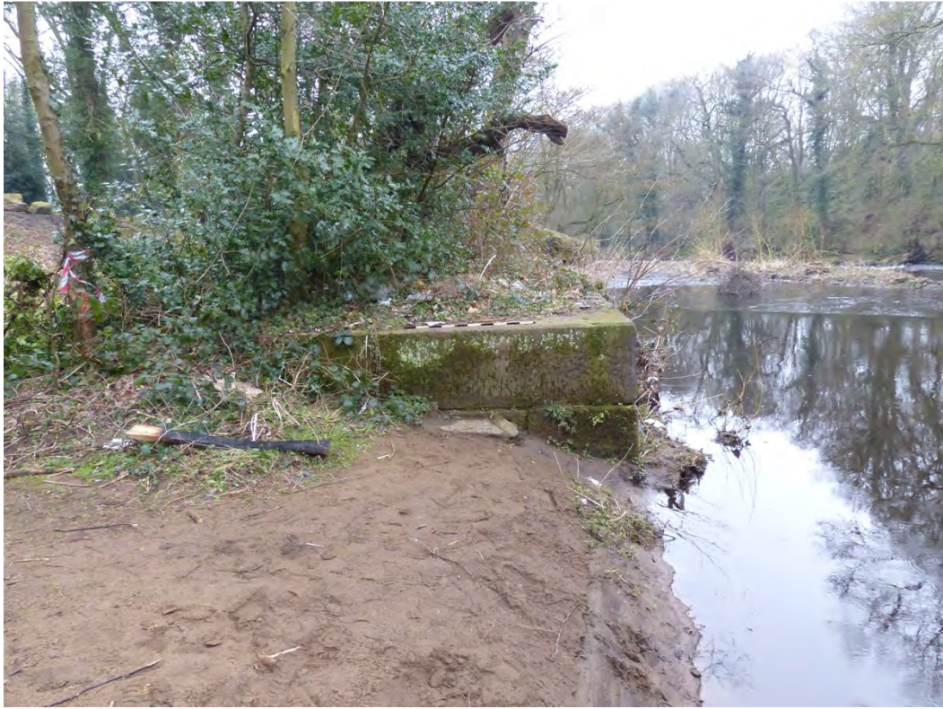
Plate 15: North end of east bank wall viewed from the goit
