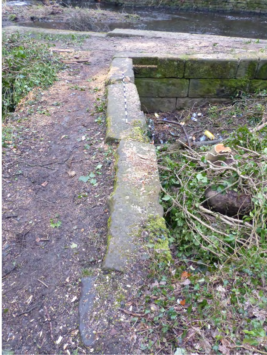
Plate 19: View across bridge to the river (scale 2m)
