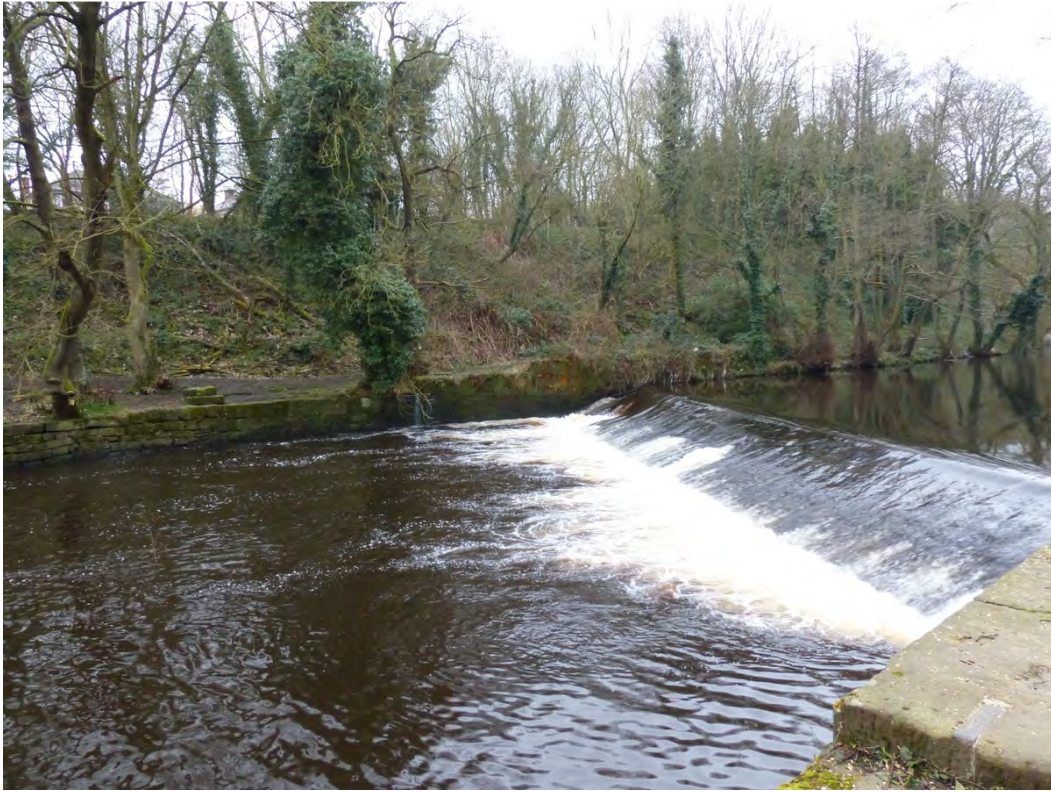
Plate 1: Beeley Wood Weir pre works, viewed facing west
