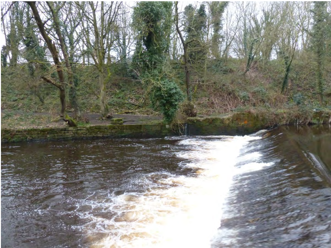
Plate 12: West bank revetment wall showing construction changes
