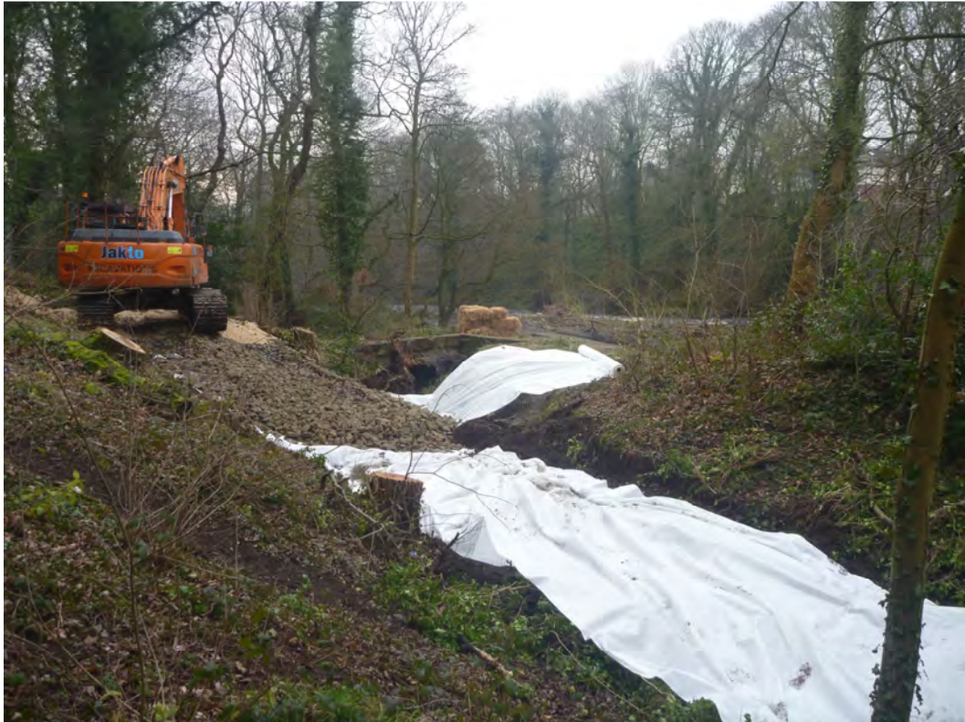
Plate 3: Construction of access along the goit
