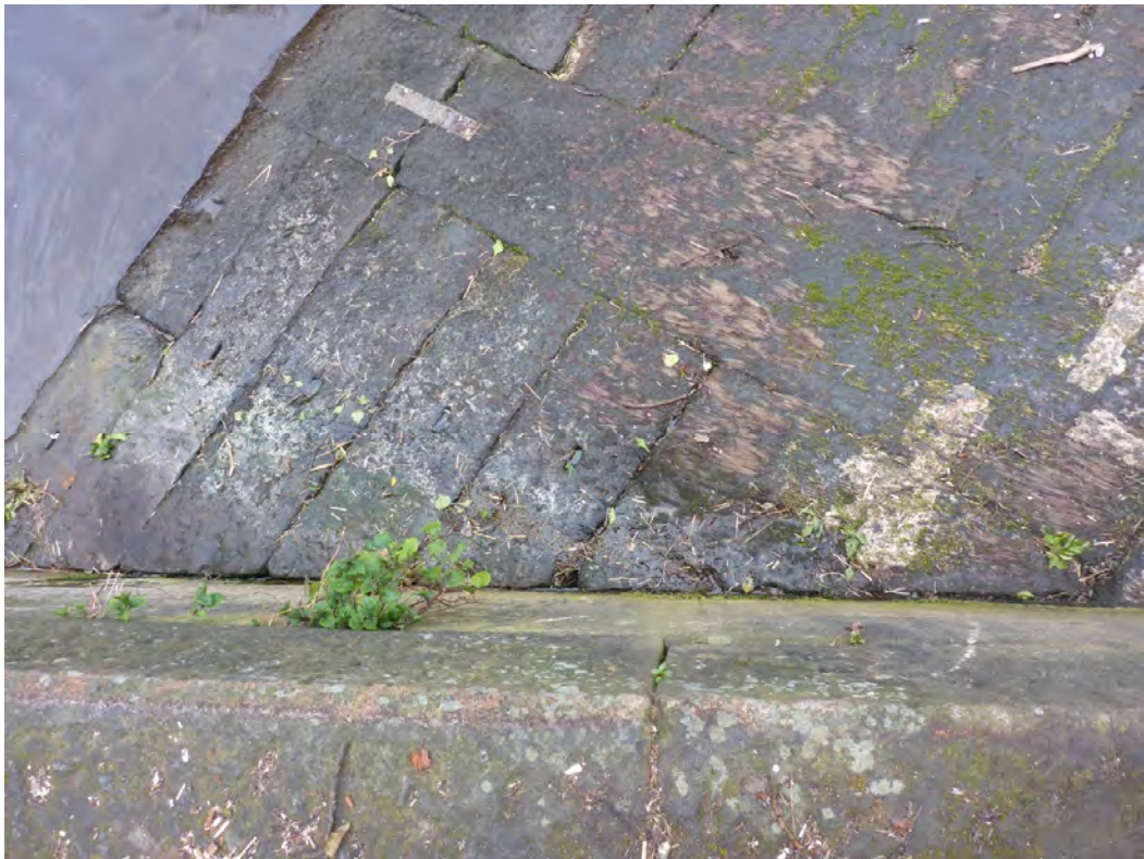
Plate 14: Weir abutting wall on east river bank
