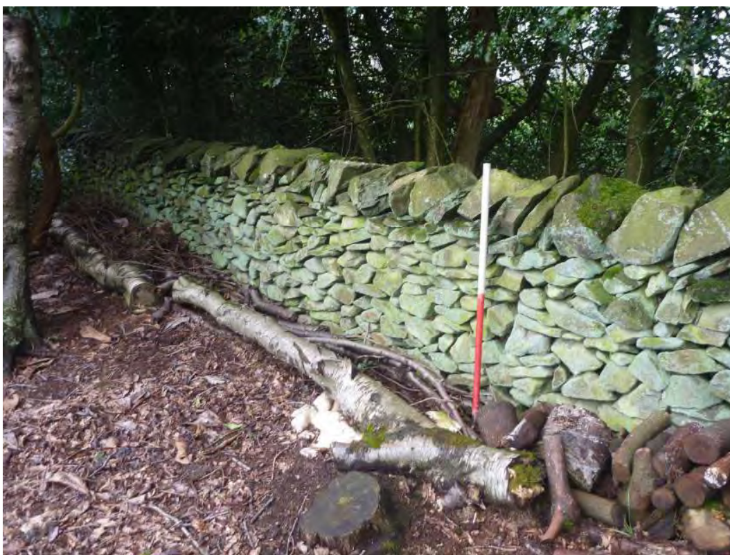
Plate 4: Boundary wall 209 at the northern side of Stoneywell Cottage grounds
