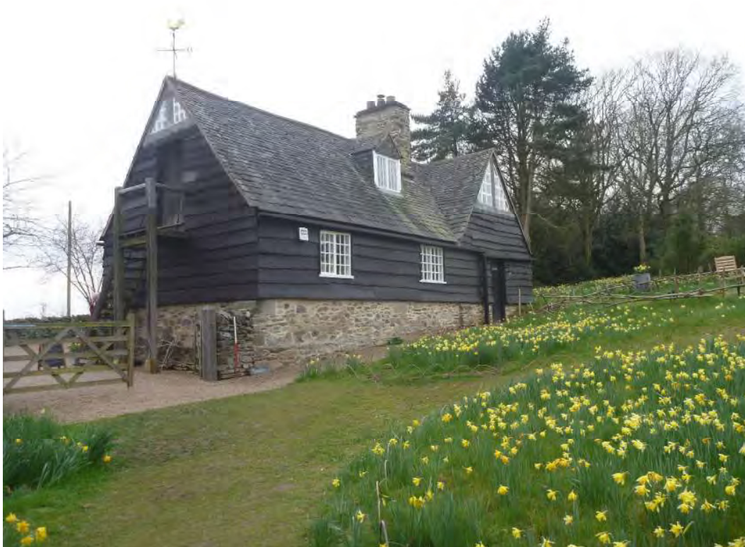
Plate 10: Northeast elevation of coach house (feature 125), viewed facing west
