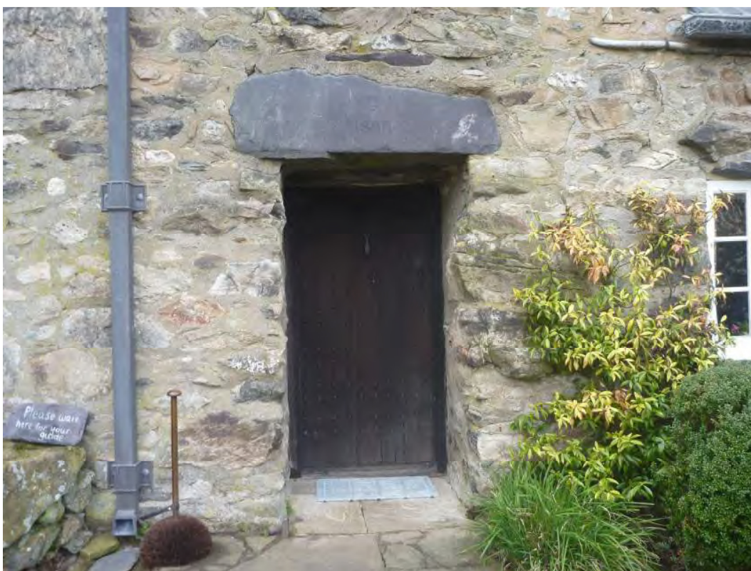
Plate 6: Main doorway to Stoneywell Cottage, showing datestone, viewed facing west
