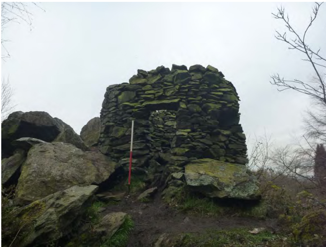
Plate 11: 'Tower' fort, feature 117, viewed facing east
