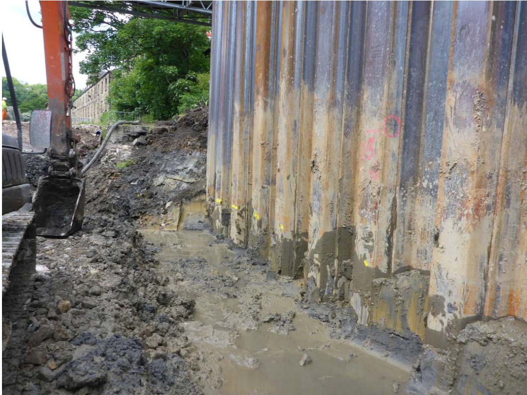
Plate 3: Grey clay under the northern bridge footings, with brown clay canal lining in section, viewed facing northwest
