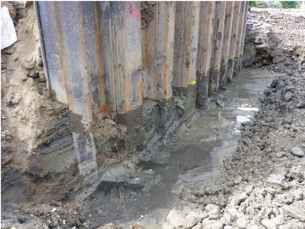
Plate 2: Grey clay underlying the southern bridge foundations, viewed facing southwest
