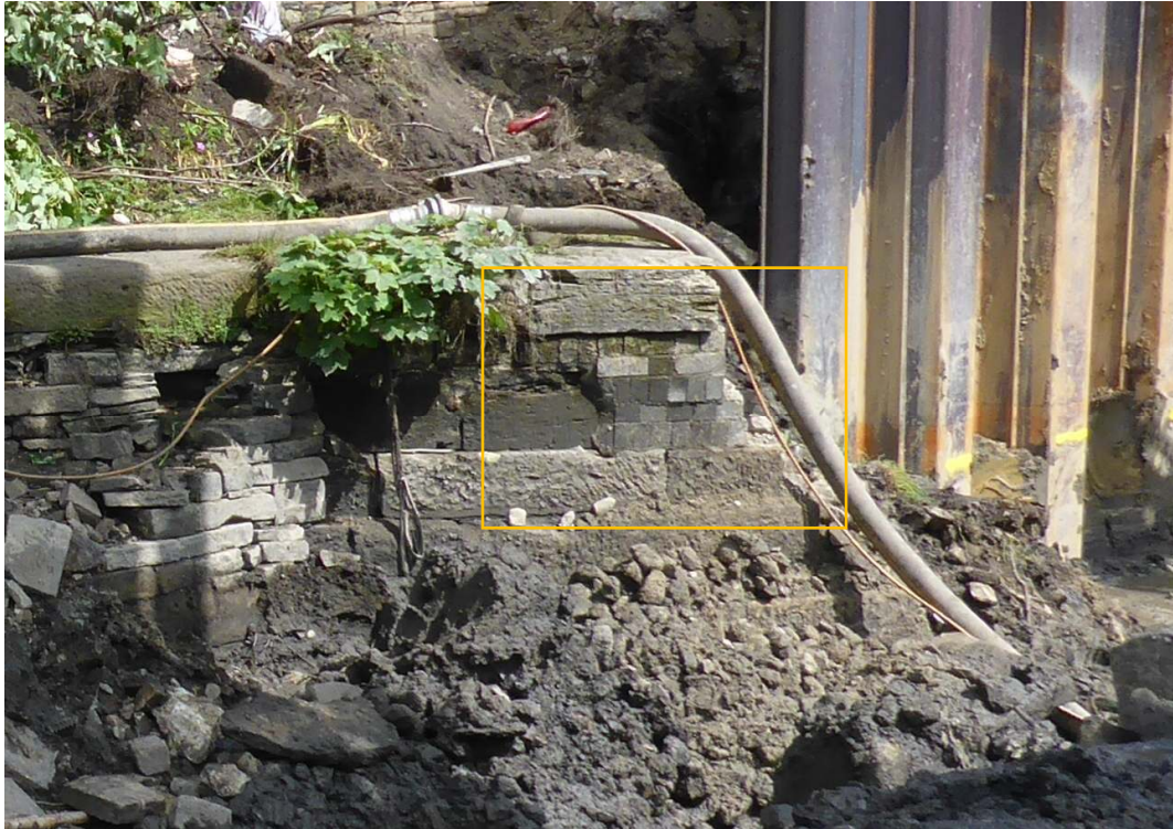
Plate 5: Detail of area of repair to bridge buttress, viewed facing north
