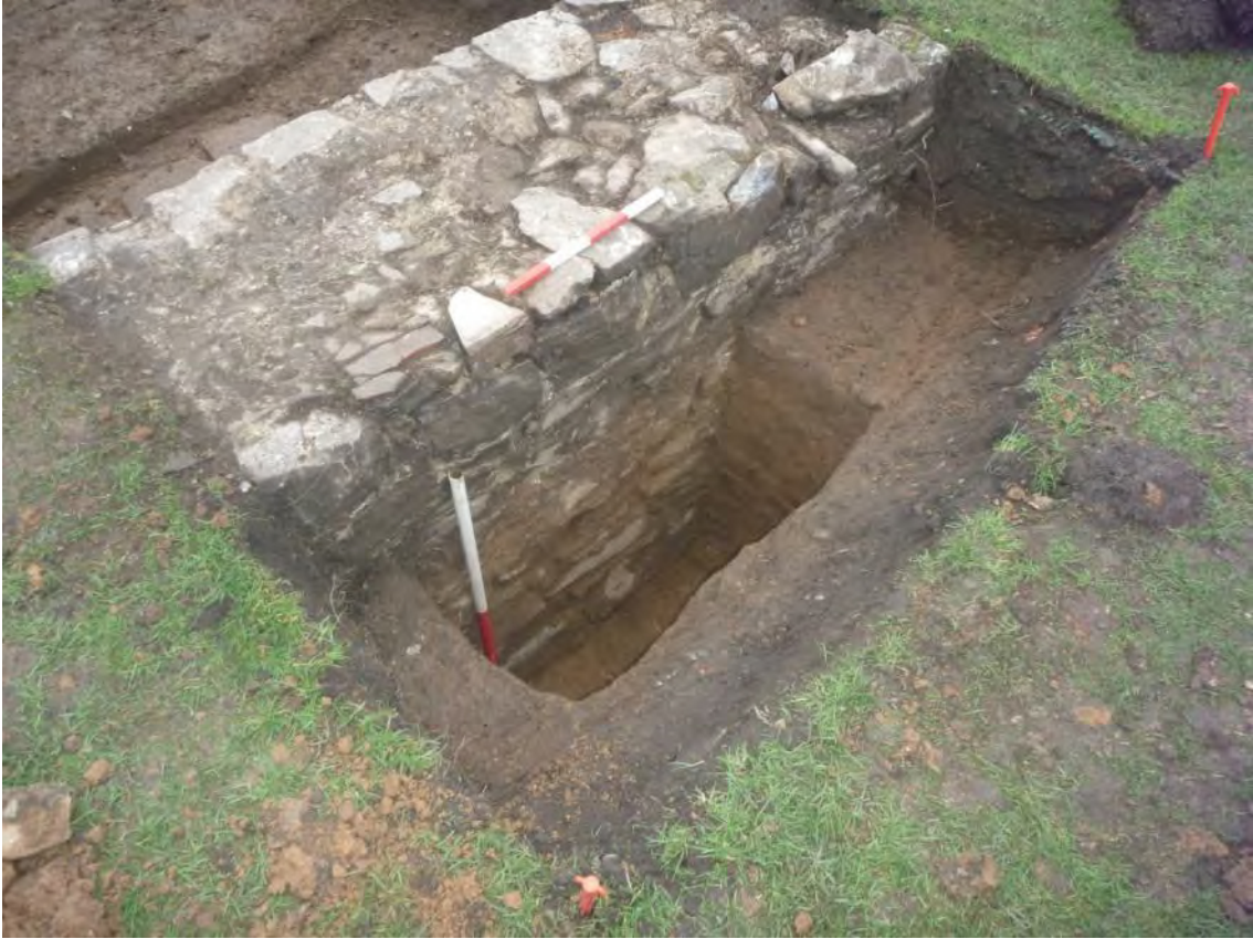
Plate 11: Wall (306), Trench 3, showing depth of foundations. Looking south, scales 1m and 0.40m.
