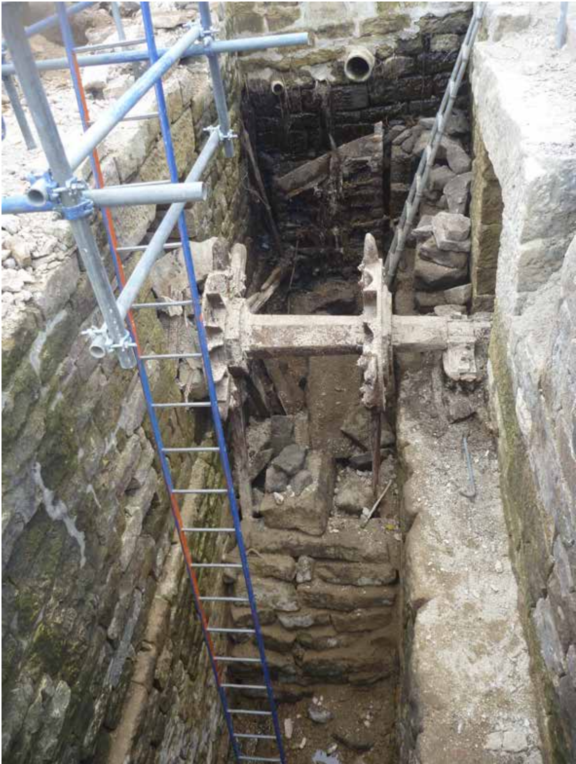
Plate 1: Exposed wheel pit, looking west
