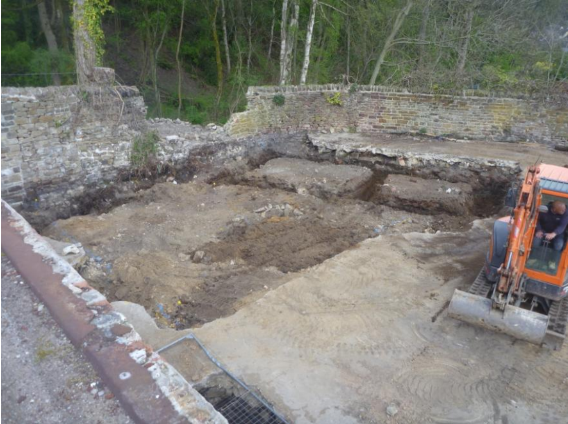
Plate 16: Working shot of the excavation of the footings within Area F. Looking north-east
