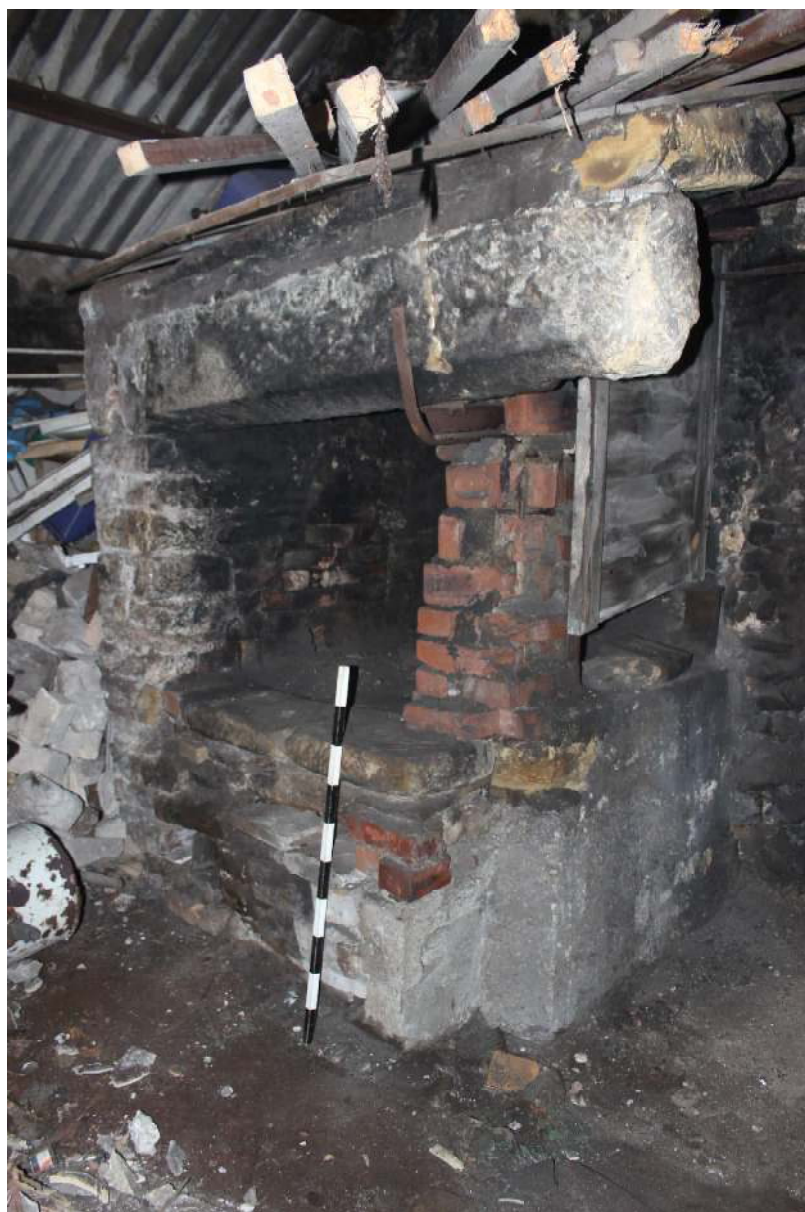
Plate 15: Hearth, showing reused stone lintel and support brickwork
