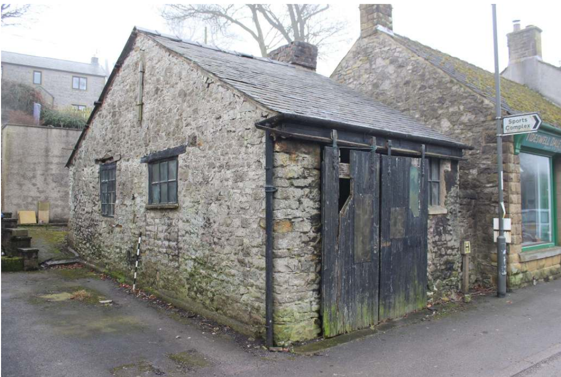
Plate 6: View of the former smithy, looking south
