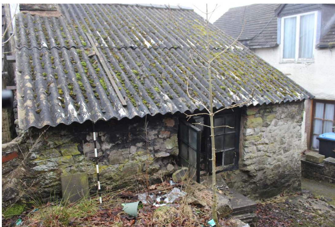
Plate 9: South side with external raised platform in foreground
