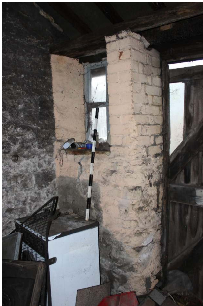
Plate 12: Internal walling by main entrance
