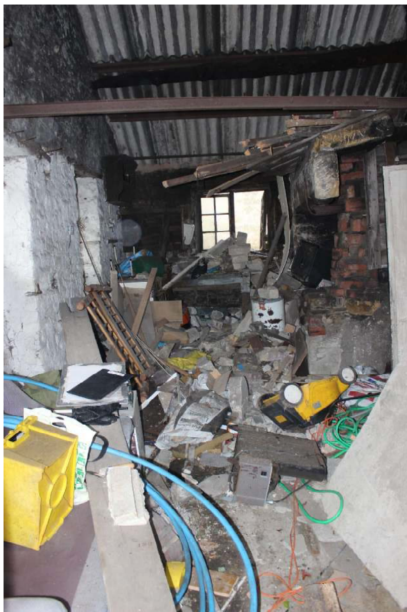
Plate 11: The debris-filled interior of the former smithy, as found in February 2017
