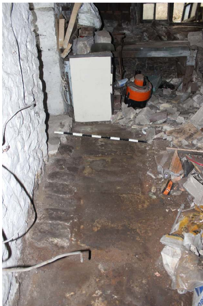
Plate 20: Line of hard stones set against east wall, probably the base for a water trough
