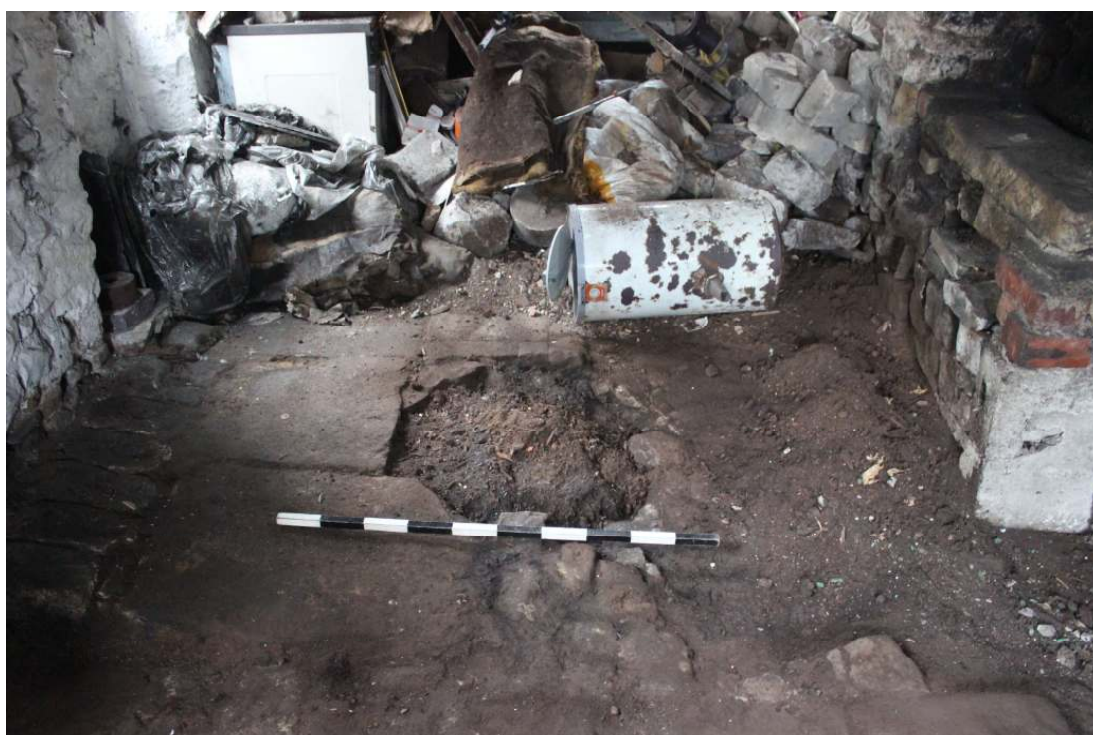
Plate 19: Worn away part of the slab flooring near the hearth (to right) where the support block for the anvil had been set
