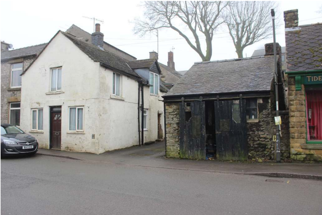
Plate 5: Frontage of the former smithy and the owner's cottage on Commercial Road
