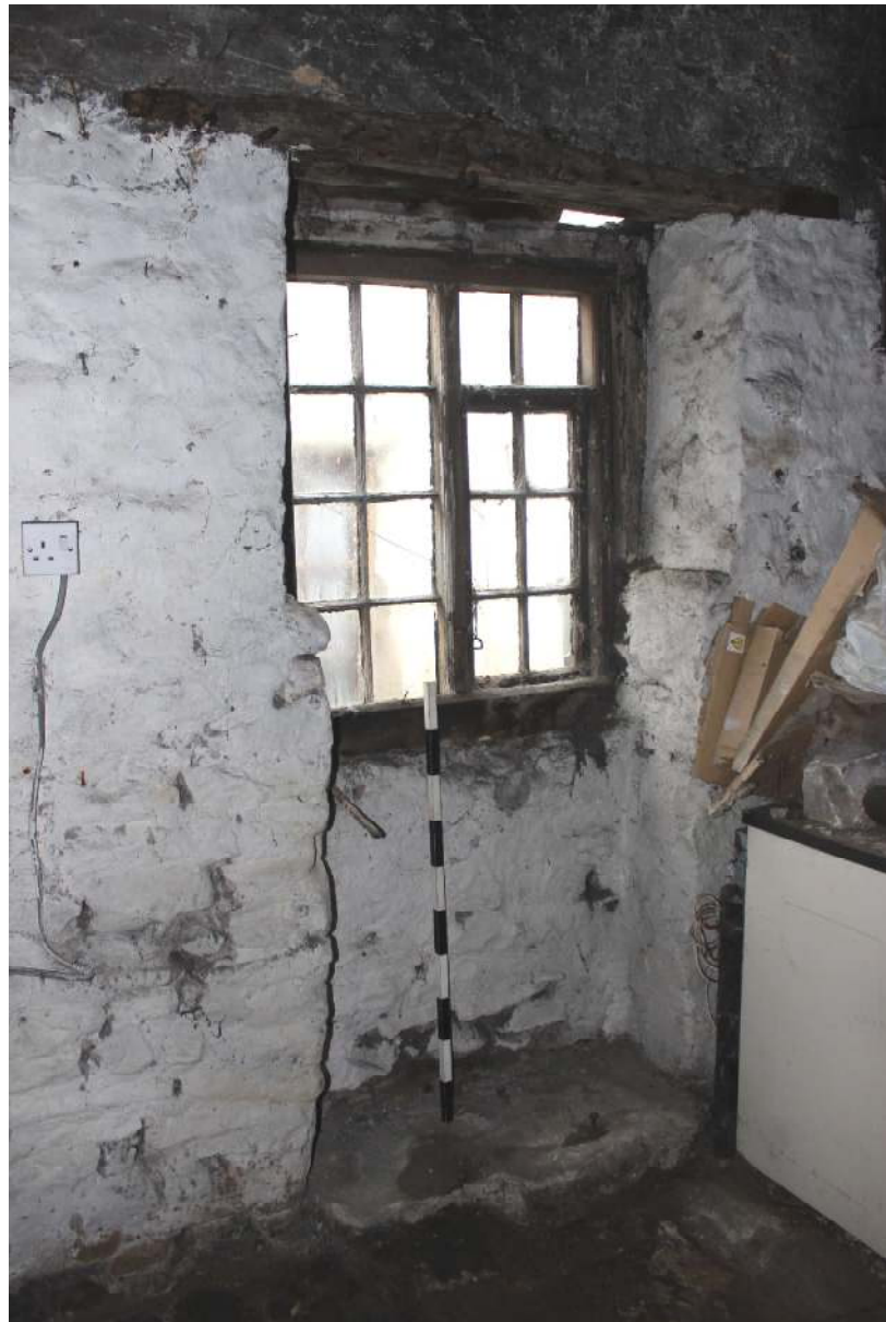
Plate 13: Recessed window opening with shoulders for former high window
