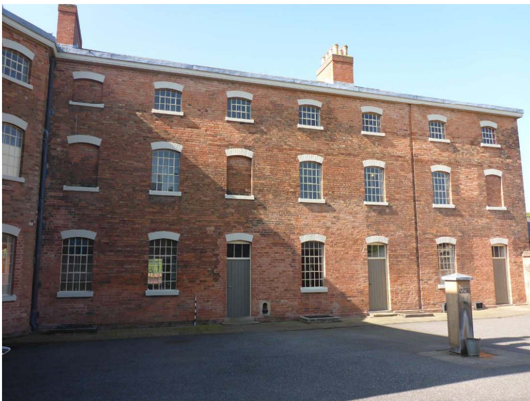
Plate 3: North elevation of women's accommodation wing, viewed facing southwest
