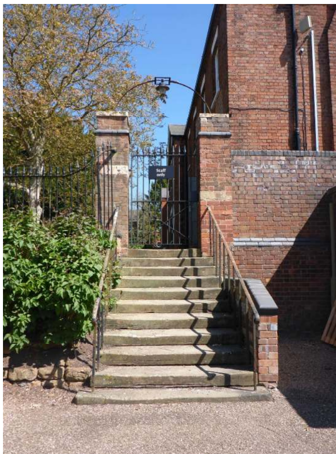
Plate 22: Steps and railings to Firbeck House (asset 114)
