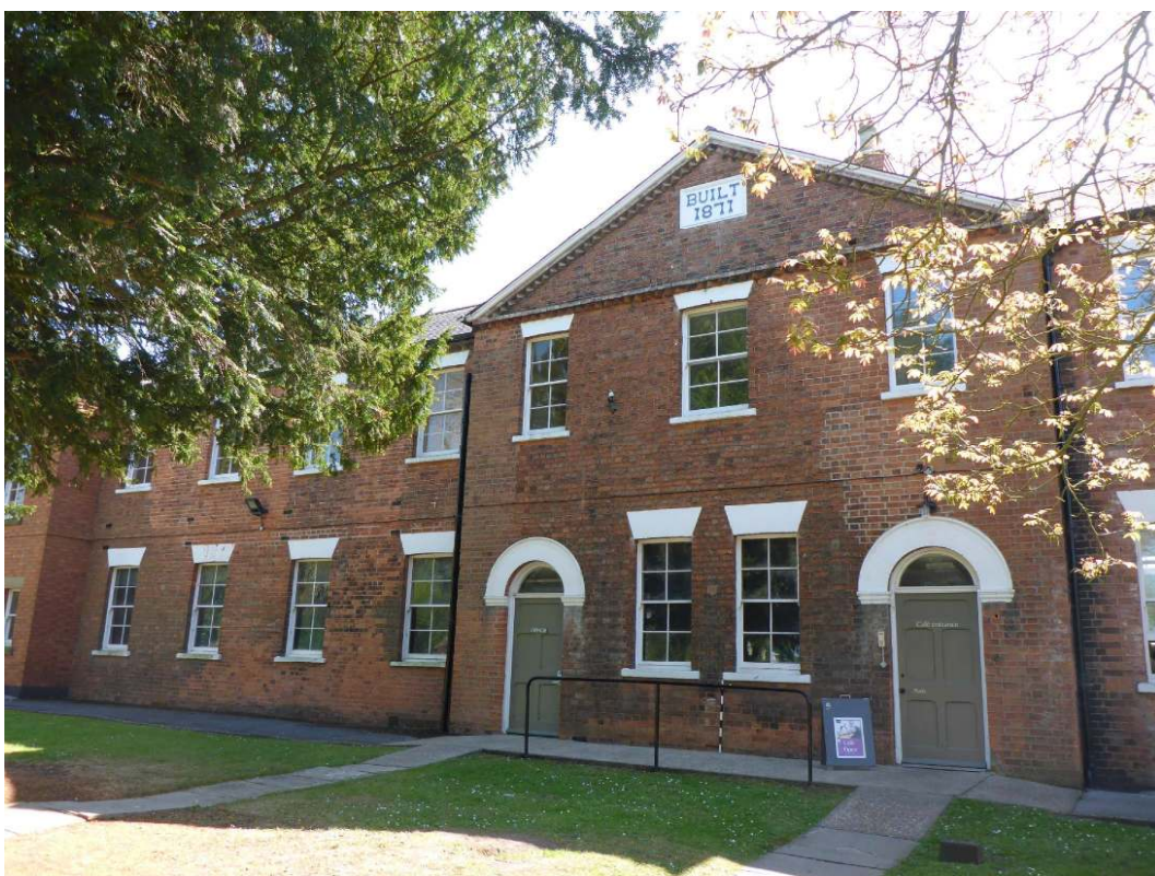
Plate 23: Central entrance gable and north wing of Firbeck House (asset 113), facing east
