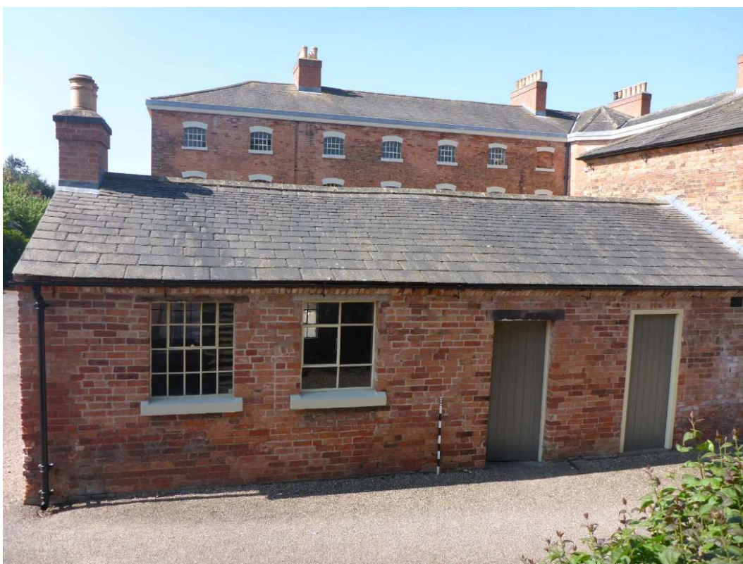
Plate 17: North elevation of former cow house (asset 102), viewed facing south
