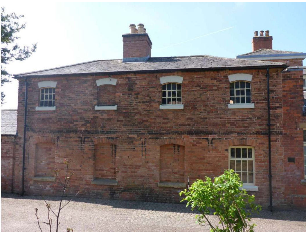
Plate 15: North face of laundry/infirmary (asset 102), showing staining possibly from former coal bins, and stone setts (asset 117)
