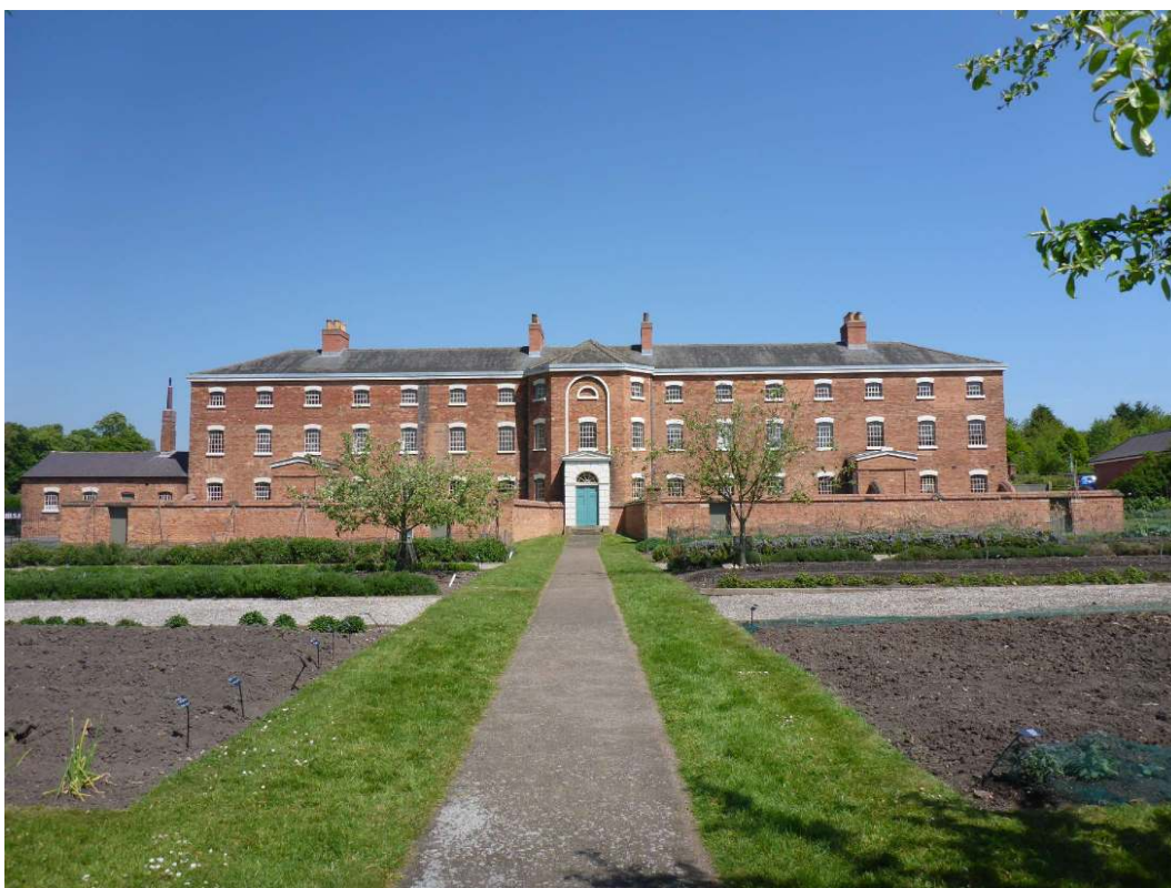
Plate 1: South front of The Workhouse (asset 101), looking towards the formal entrance
