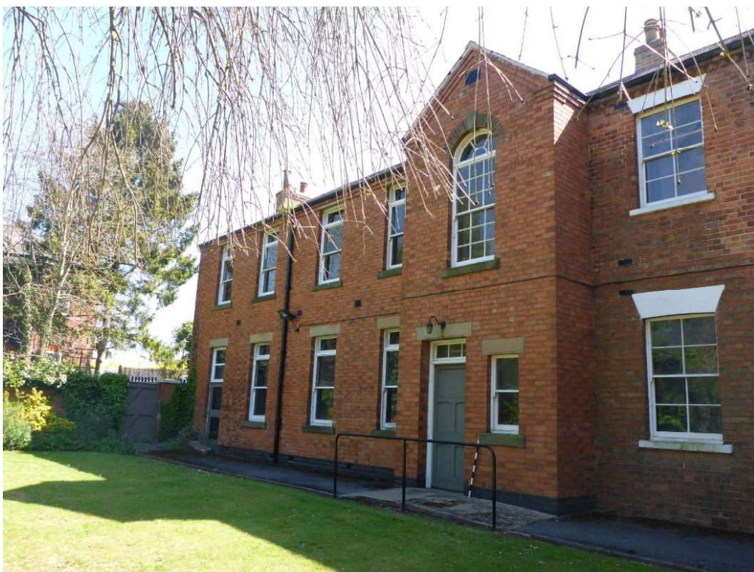
Plate 24: Northern extension of Firbeck House (asset 113), viewed facing northeast
