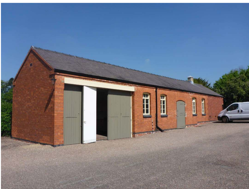
Plate 20: East elevation of garage/stable (asset 112), viewed facing north
