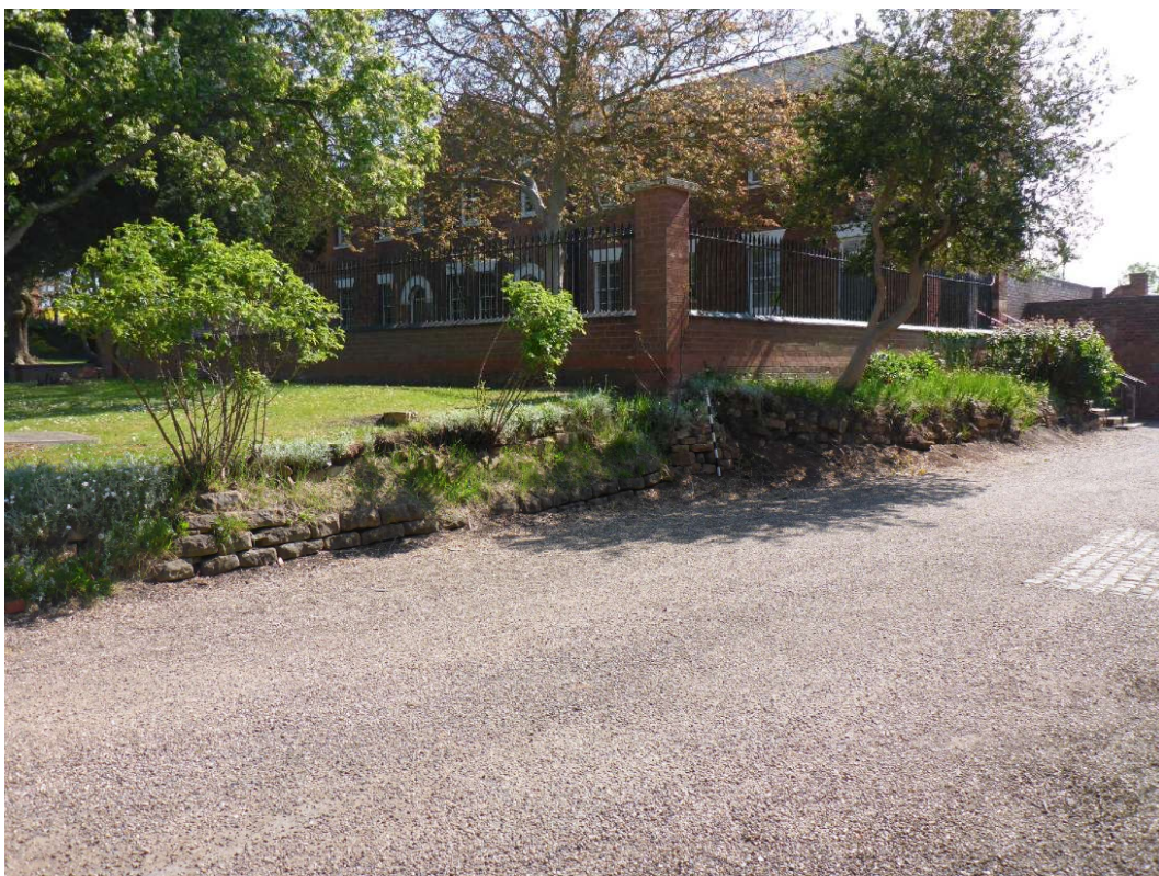
Plate 25: Stone revetment wall (asset 116), viewed facing northeast
