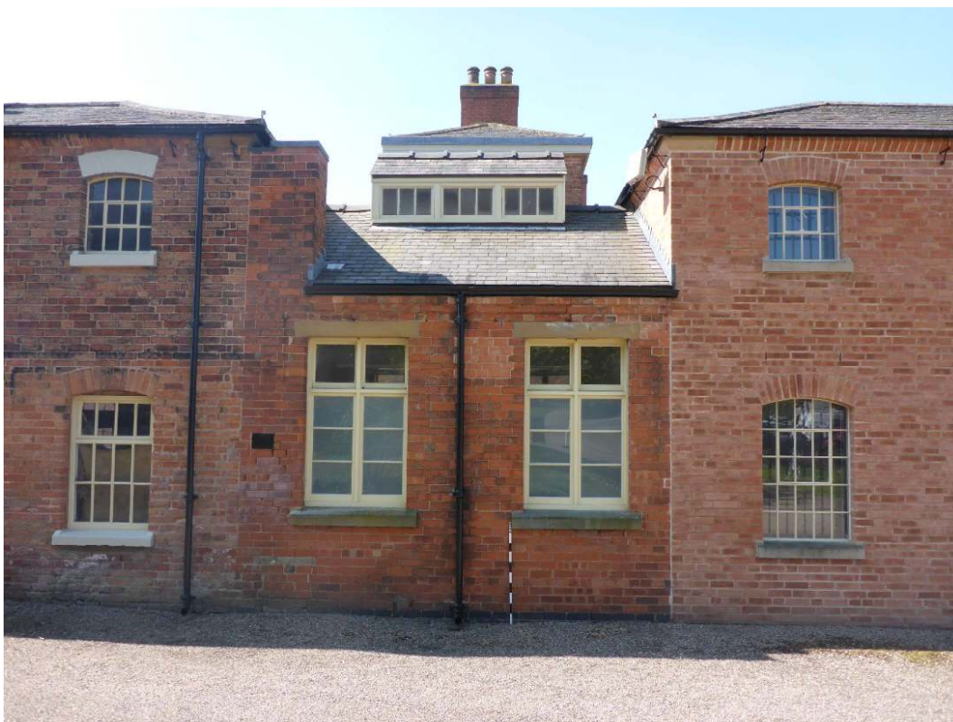
Plate 13: North elevation of drying room (asset 102), viewed facing southwest
