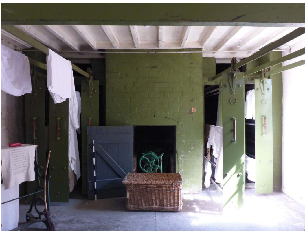
Plate 14: Interior of laundry/infirmary building (asset 102), showing drying racks
