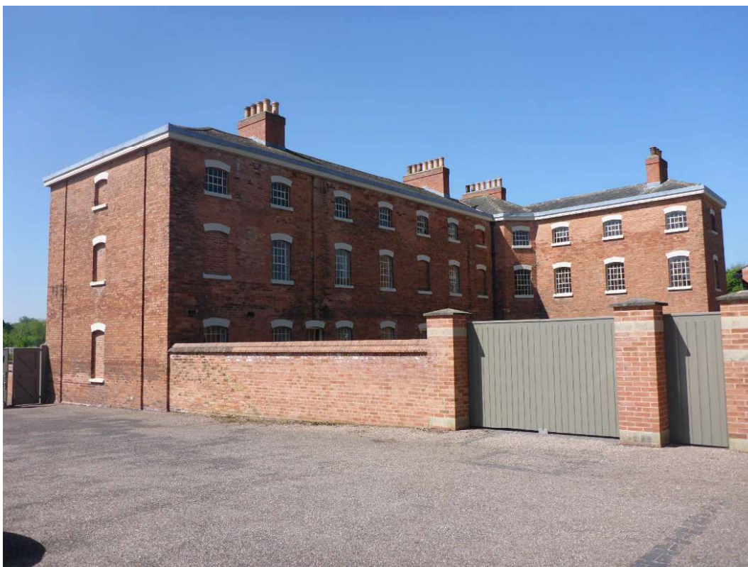
Plate 5: East gable of accommodation block and restored work yard wall, facing southwest
