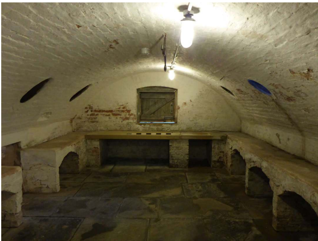
Plate 9: Basement room in main accommodation block, viewed facing west
