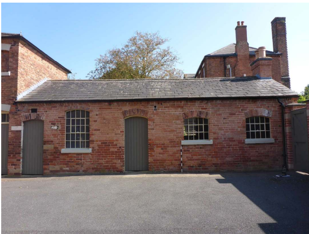
Plate 16: South elevation of former cow house (asset 102), viewed facing north
