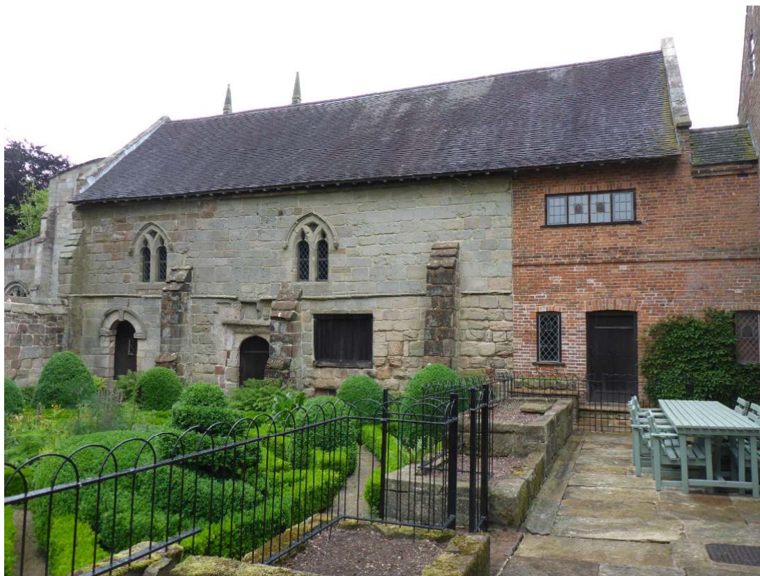
Plate 5: West elevation of the medieval wing of Norbury Manor (asset 101), viewed facing east
