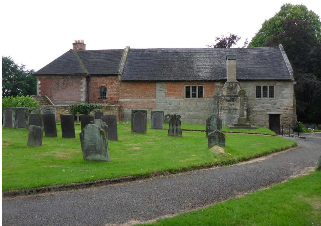
Plate 7: East elevation of Norbury Old Manor (101 & 102), viewed facing west
