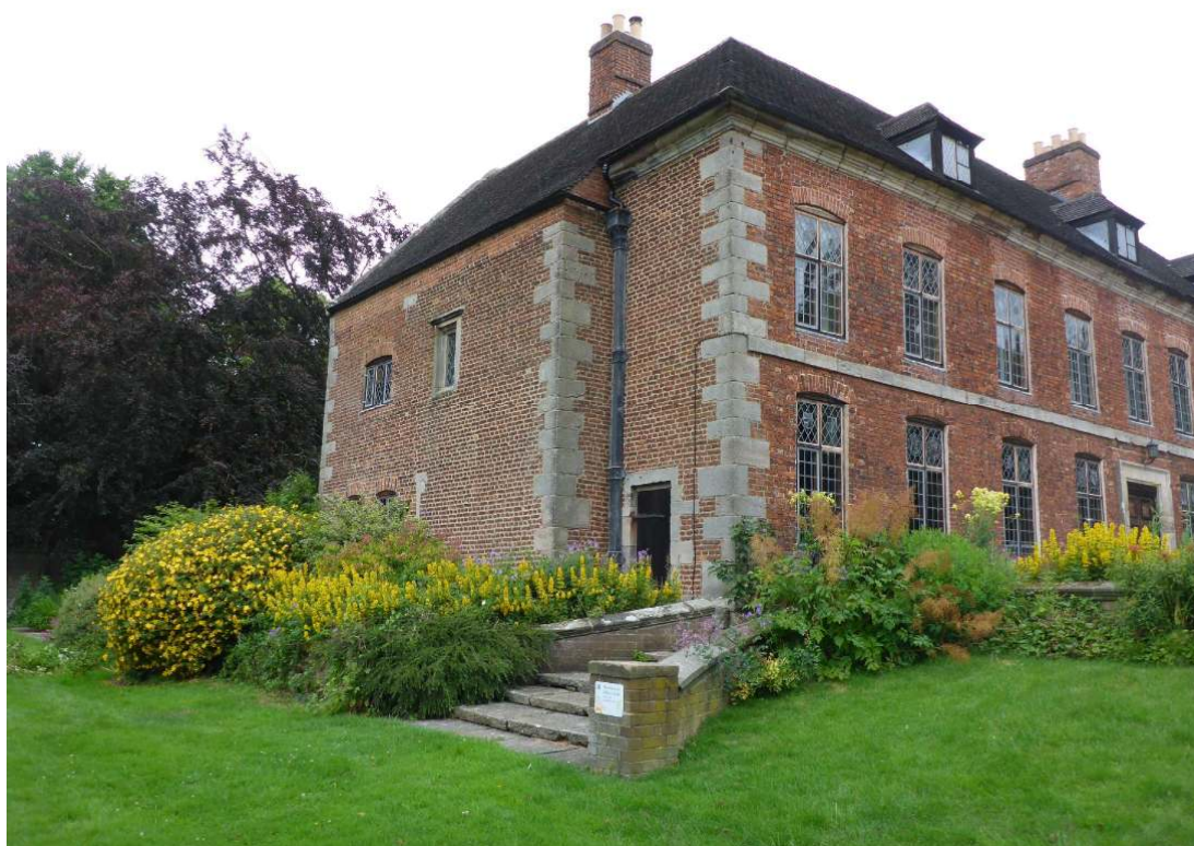
Plate 9: West elevation of the 17 th -century building (102), viewed facing northeast
