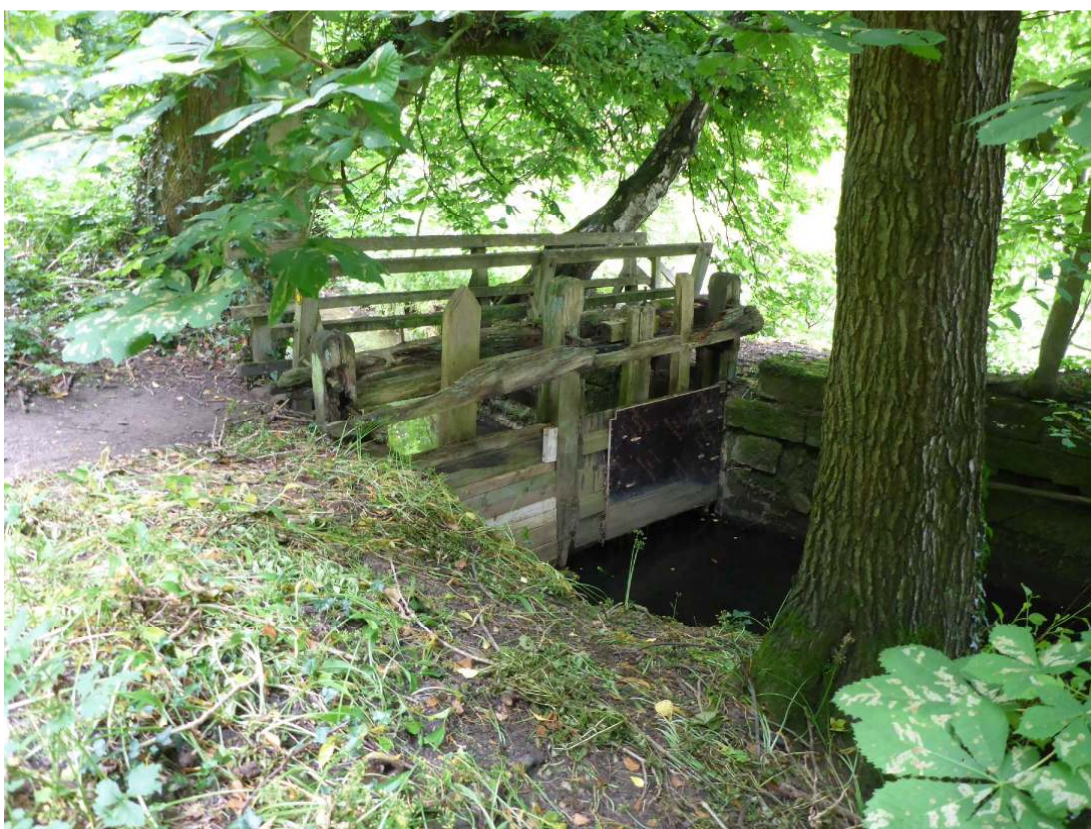
Plate 28: Wooden sluice gate (140) and mill race revetment, viewed facing west
