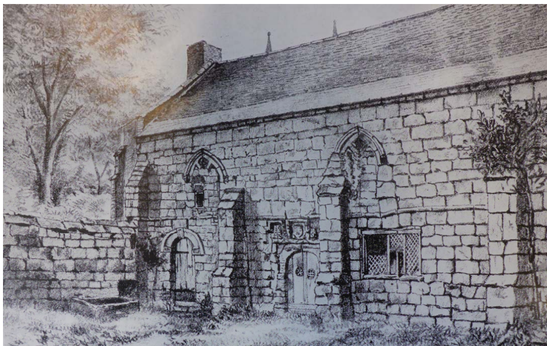
Plate 1: West front of the medieval wing (asset 101) c.1885, viewed facing northeast
