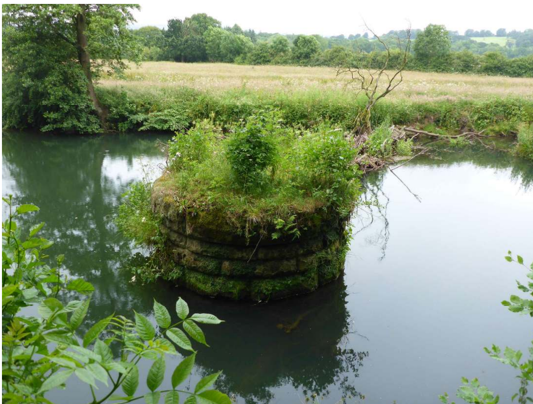
Plate 27: Circular pier for railway bridge (asset 135), viewed facing northwest
