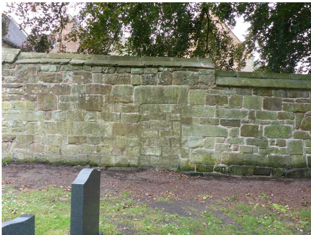
Plate 11: North elevation of courtyard wall (asset 103), showing blocked gate
