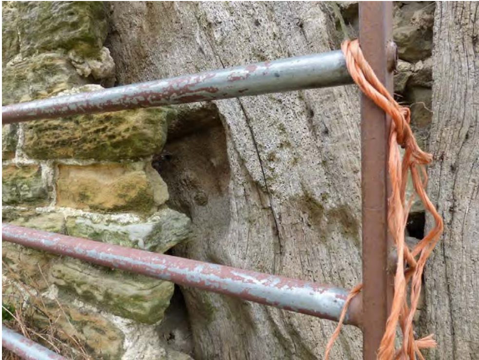
Plate 13: Cruck 1 base looking south-east and showing empty dovetail joint behind gate
