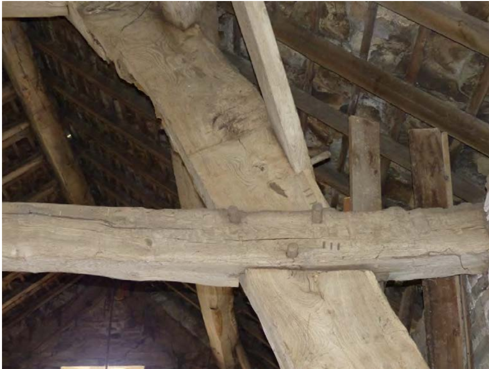
Plate 7: Detail of Cruck 2 looking north, showing assembly marks 'III'
