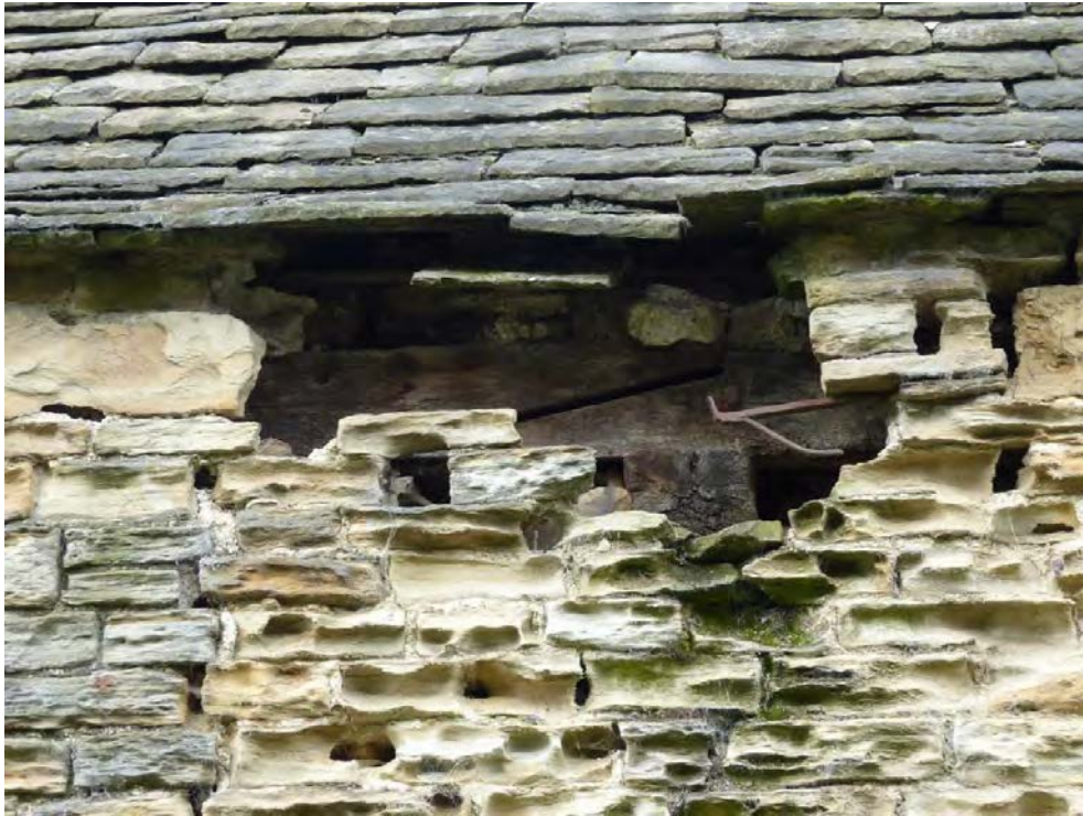
Plate 11: Detail of wall plate and tie beam looking west (Cruck 5)
