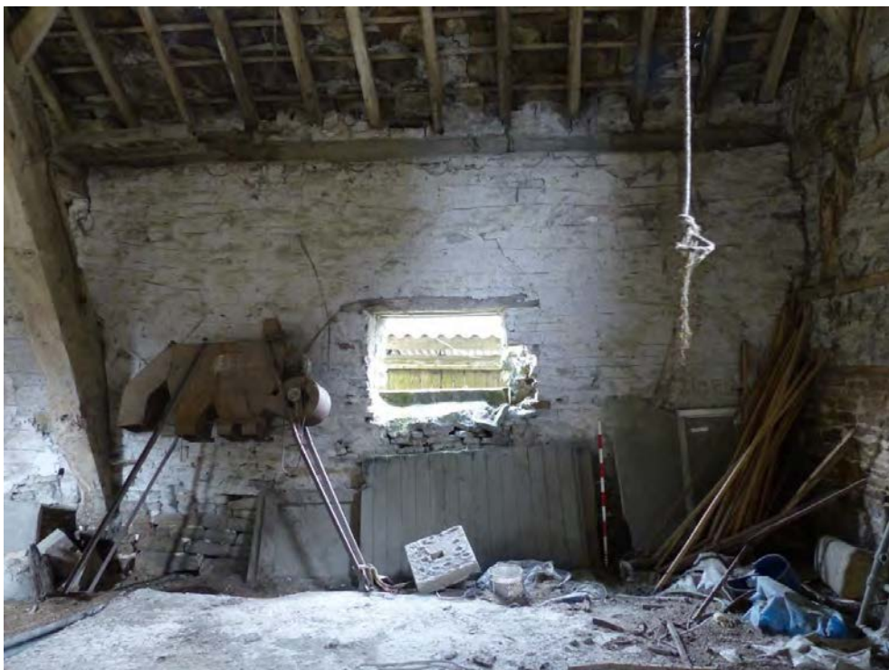
Plate 22: Bay 1 looking west showing square window
