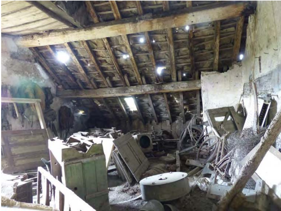
Plate 43: Area F (Bay 5) looking west
