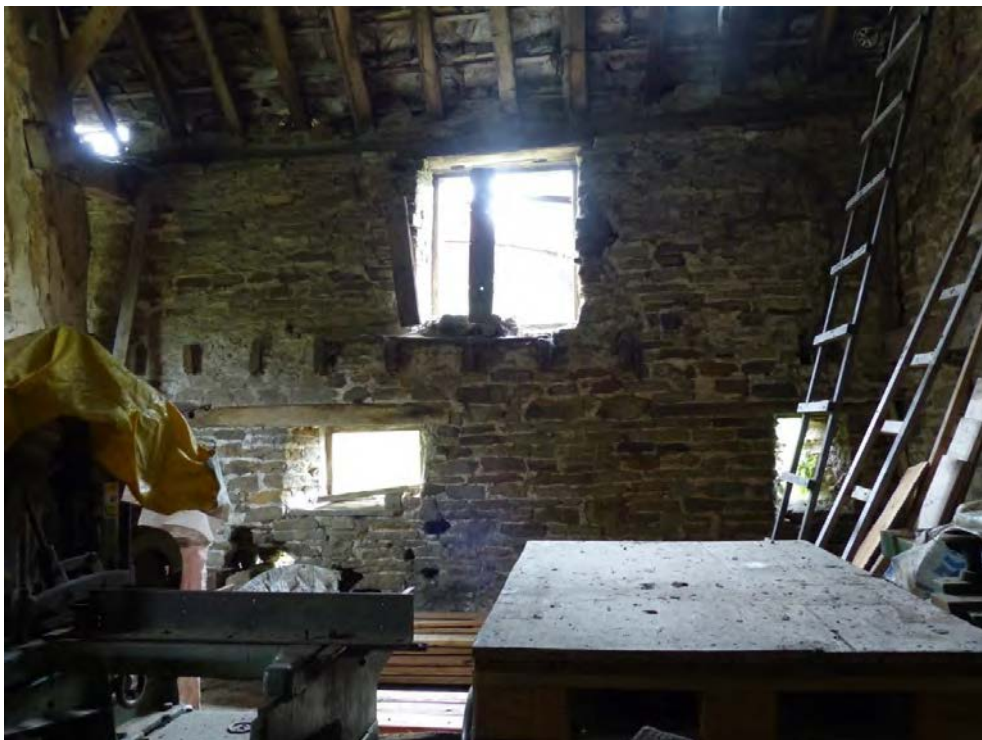
Plate 26: Bay 4 looking east showing windows
