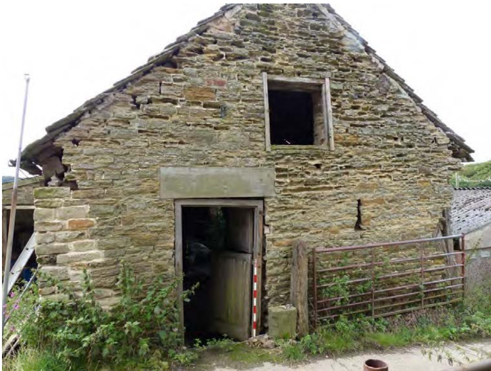
Plate 20: north gable (Cruck 1) looking south
