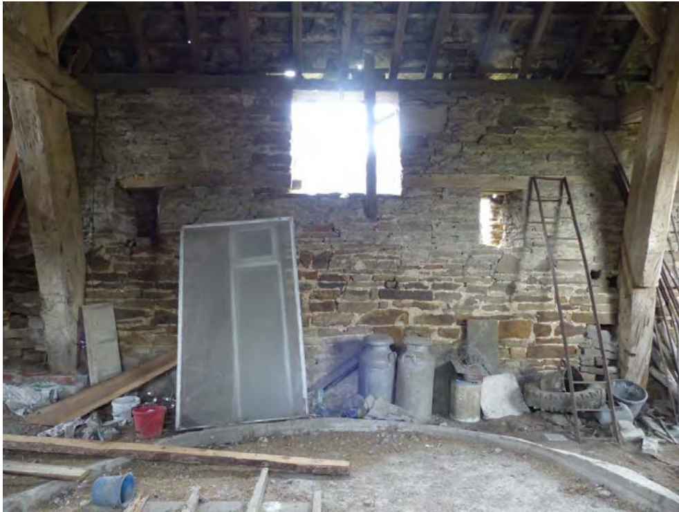
Plate 25: Bay 2 looking east and showing windows
