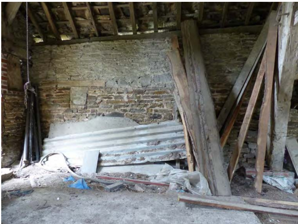
Plate 24: Bay 1 looking east showing blocked-up slit window in the interior
