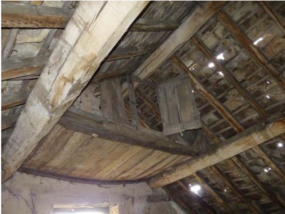
Plate 47: Area F looking south
