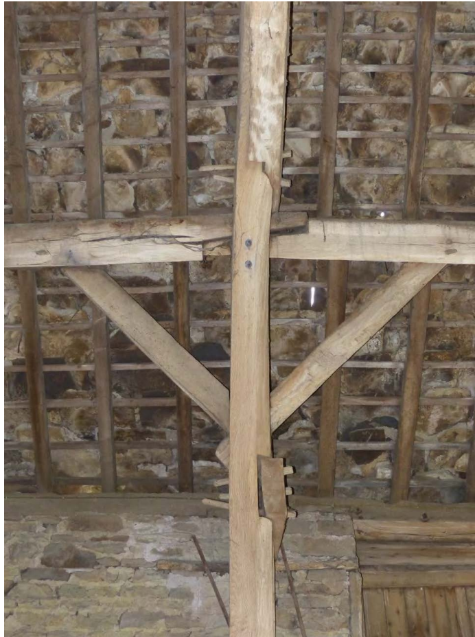
Plate 9: Cruck 4 looking west, detail of purlin and wind braces
