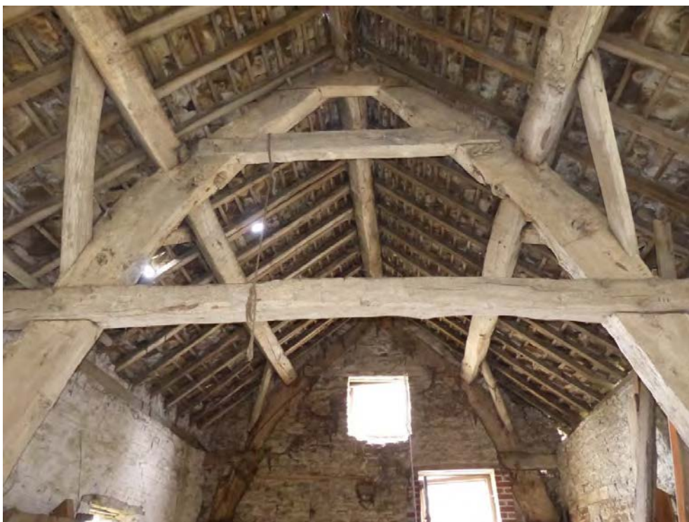
Plate 4: Cruck 2, looking north, detail of timber components
