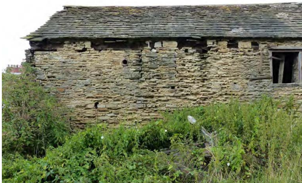
Plate 10: Bay 5 looking west. Wall plate exposed behind stonework
