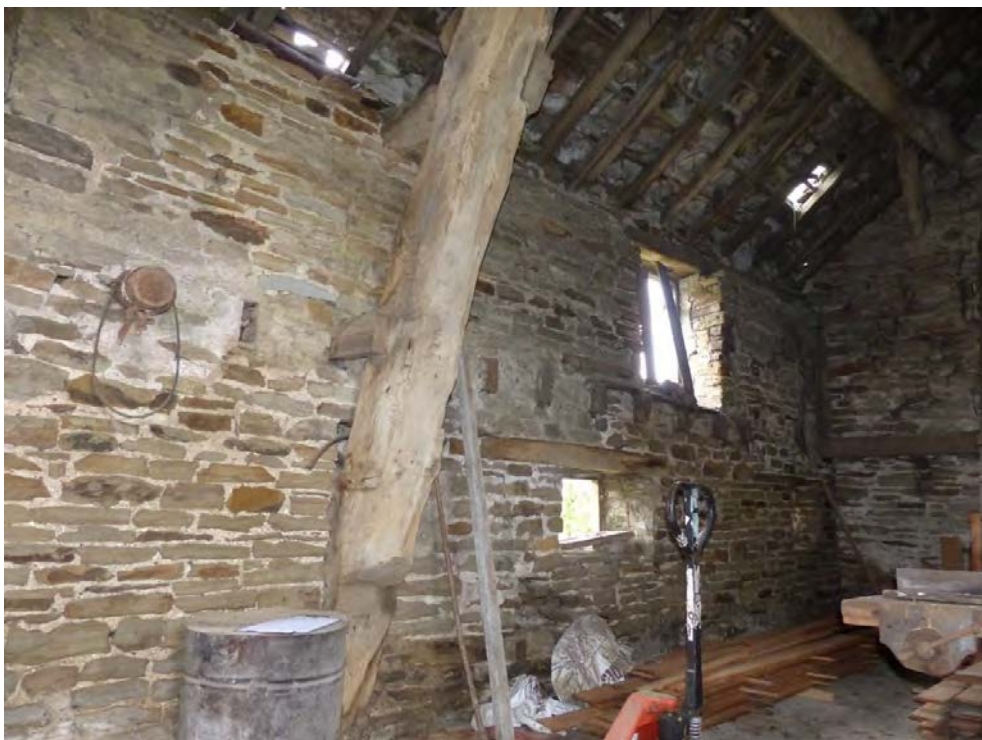
Plate 32: Bay 4 looking south-east showing remains of floor joists in east wall
