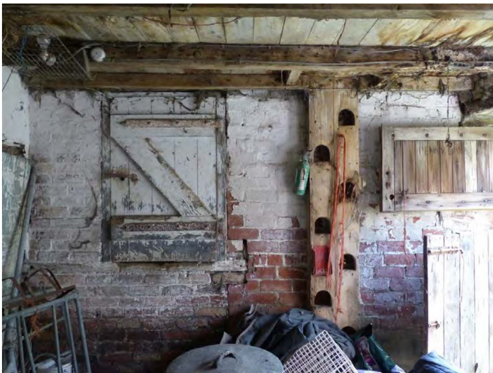
Plate 38: Area D looking south and showing brick internal wall
