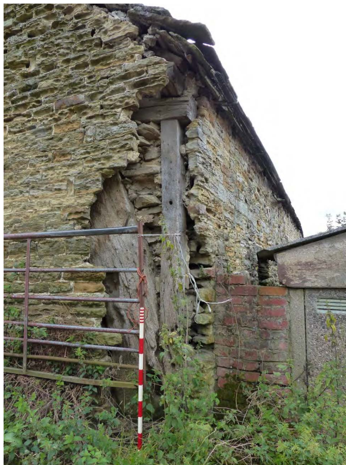
Plate 6: Cruck 1 looking south-east showing base of cruck blade and wall post
