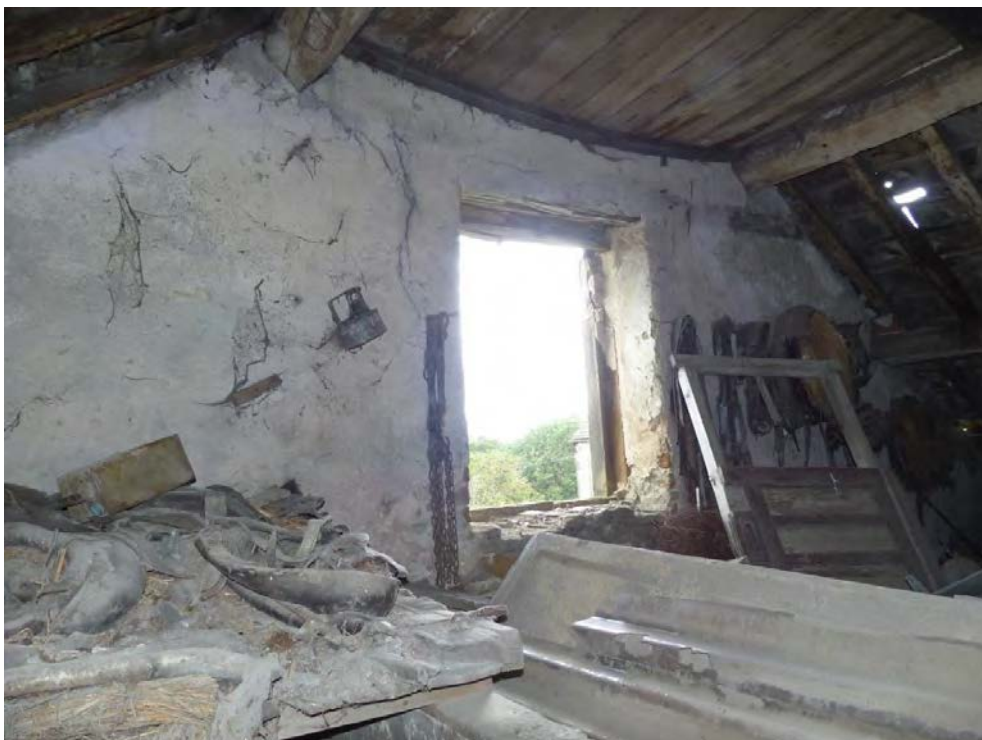
Plate 42: Area F (Bay 5) looking south-west
