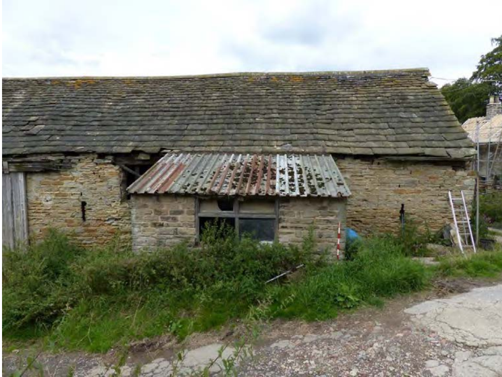
Plate 23: Bays 1 and 2 looking west and showing slit windows
