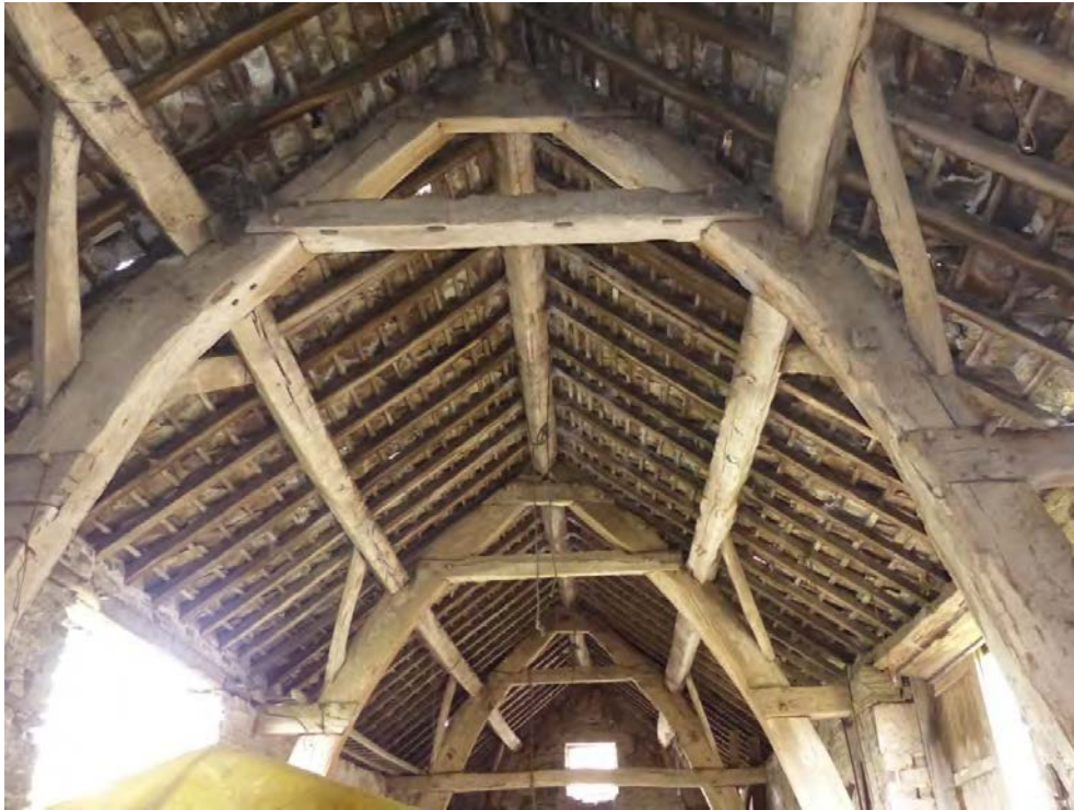
Plate 5: Crucks 3 and 4 looking north with central section of tiebeams removed
