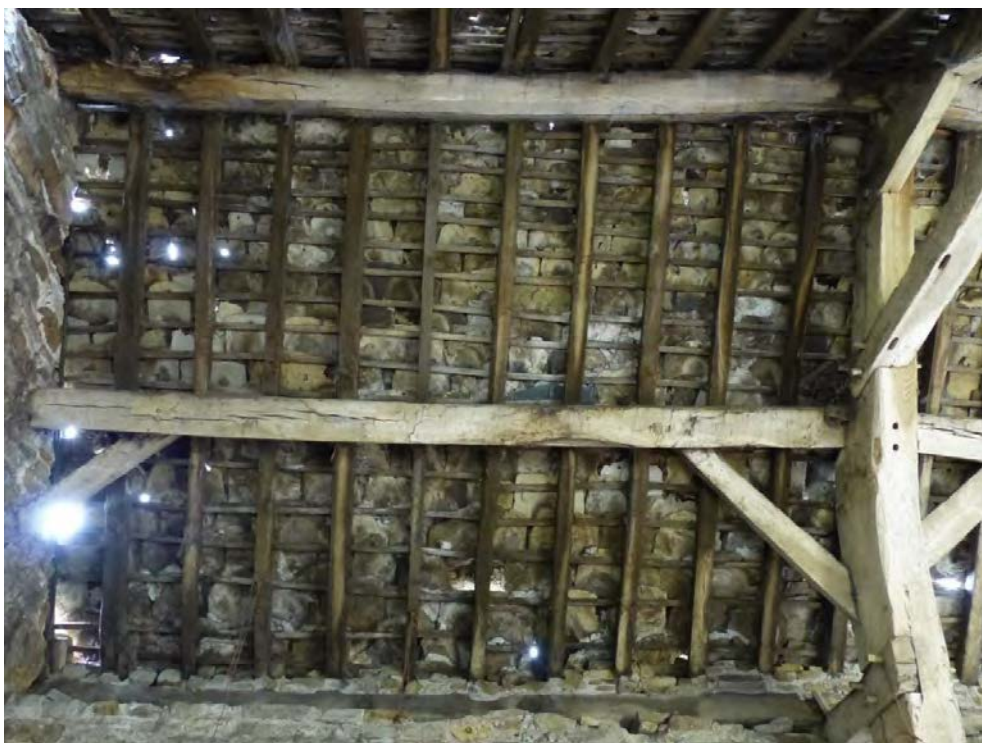
Plate 8: Detail of purlin in Bay 4, looking west
