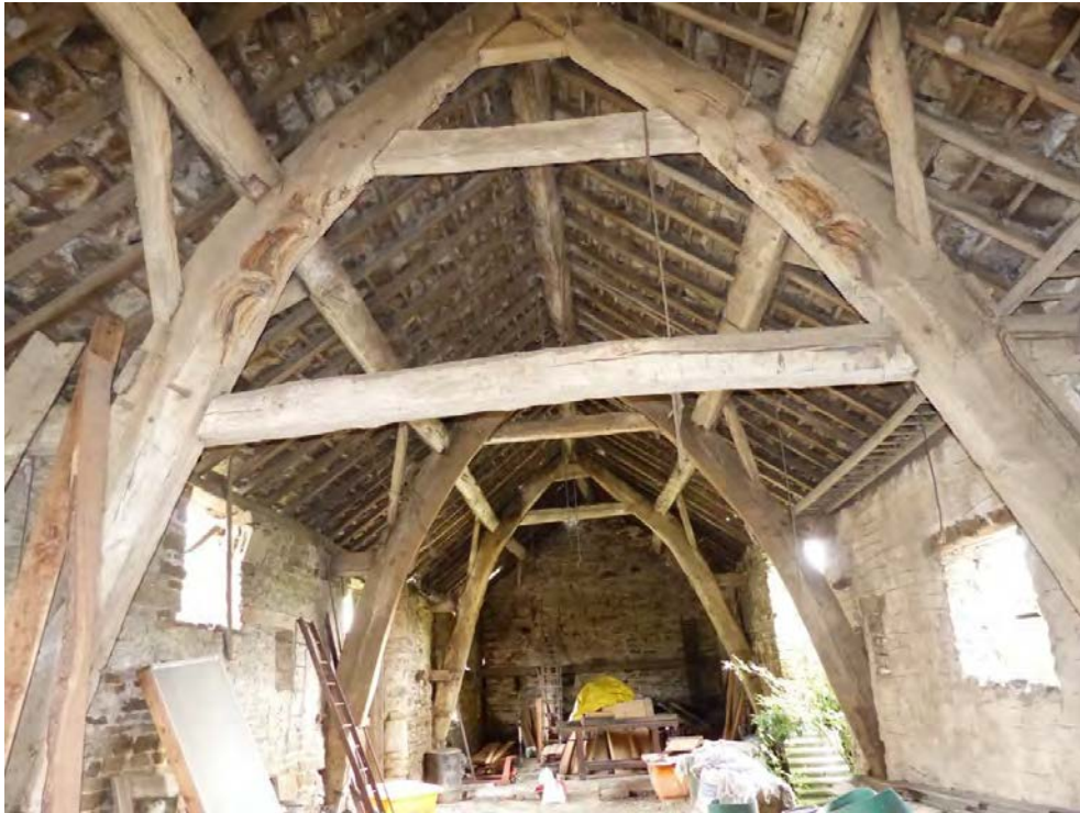
Plate 1: Crucks 2, 3 and 4 looking south
