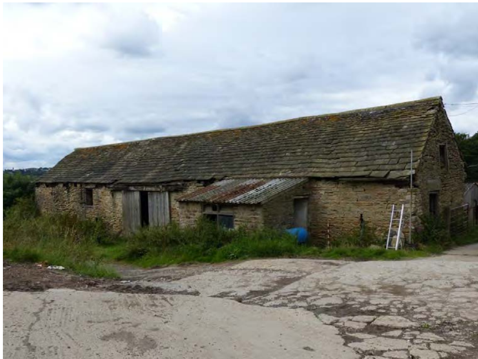
Plate 18: The Cruck Barn, looking south-west
