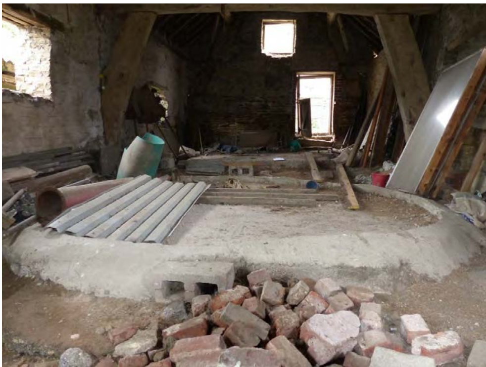
Plate 48: Area A Bays 1 and 2 showing concrete bases for grain silos
