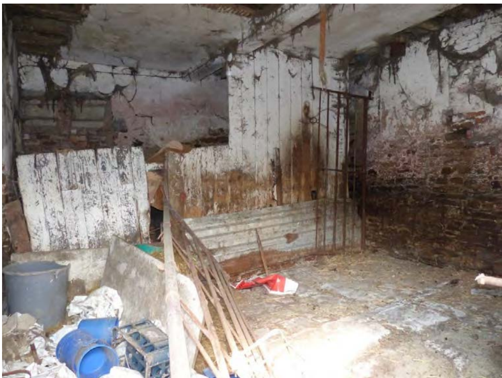
Plate 34: Area B (Bay 5) looking north-east
