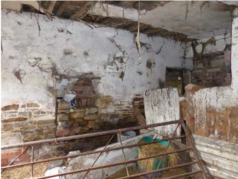
Plate 35: Area B (Bay 5) looking north-west
