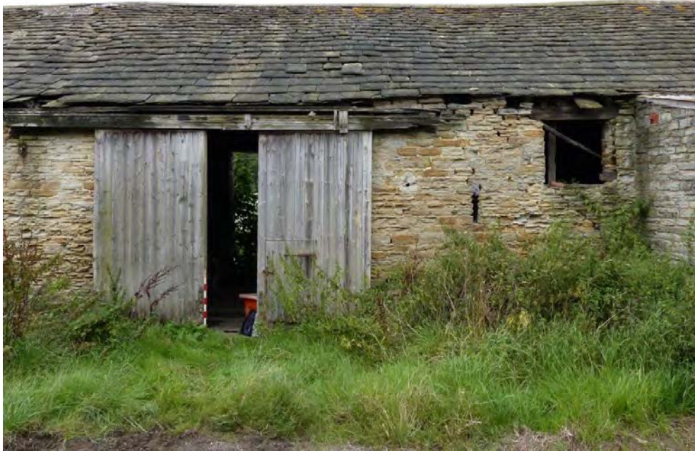
Plate 49: Bay 3 replacement sliding doors
