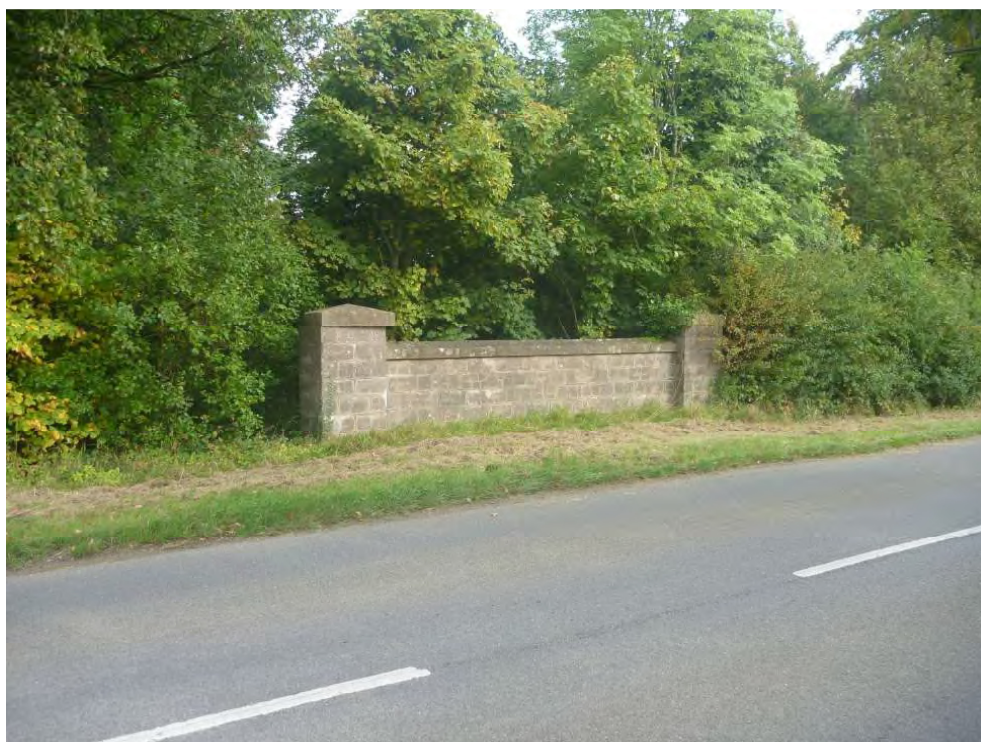
Plate 17: 1950s road bridge 305 over former mineral railway cutting
