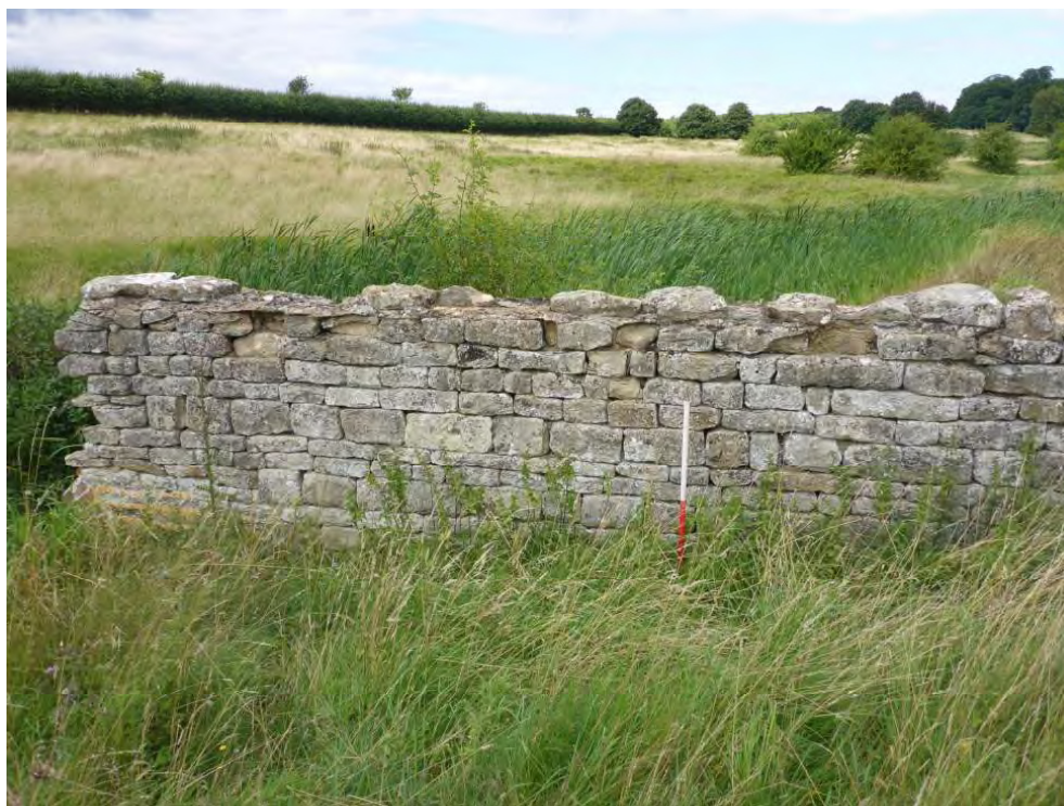
Plate 14: Ruined park boundary wall 292 south of Horn DMV, viewed facing north
