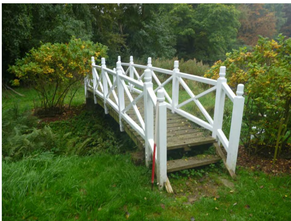
Plate 15: Modern wooden footbridge 310, crossing leat between ponds 307 and 229
