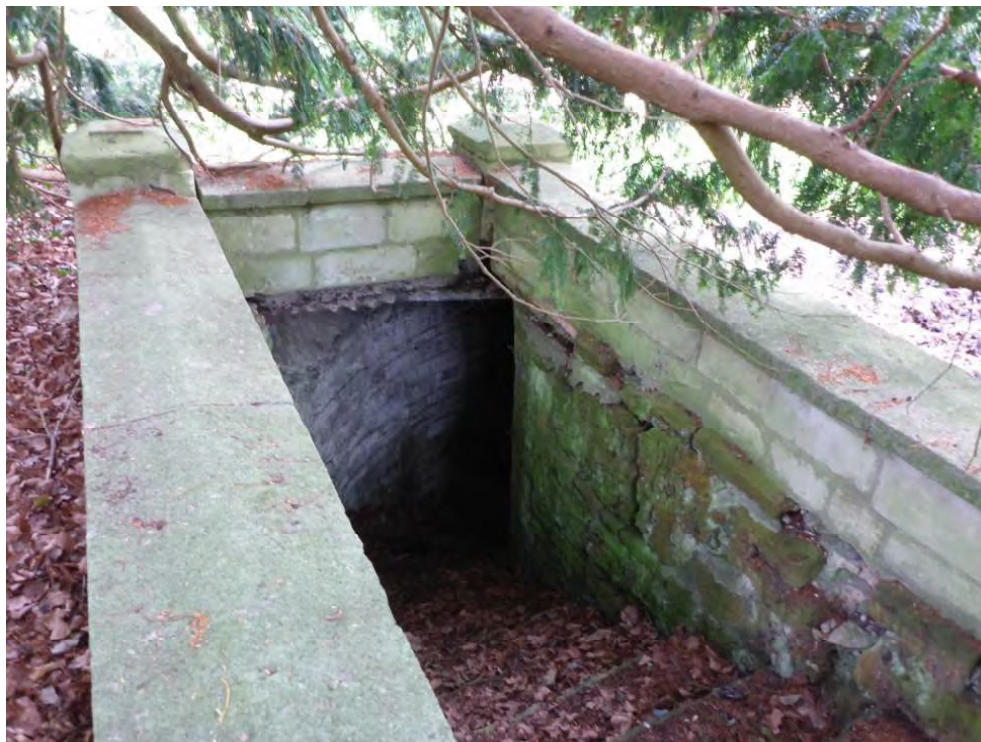
Plate 12: Stone staircase 303, viewed facing northeast
