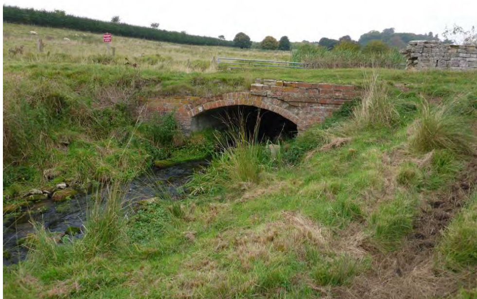
Plate 16: Brick footbridge 116 over North Brook, south of wall 292
