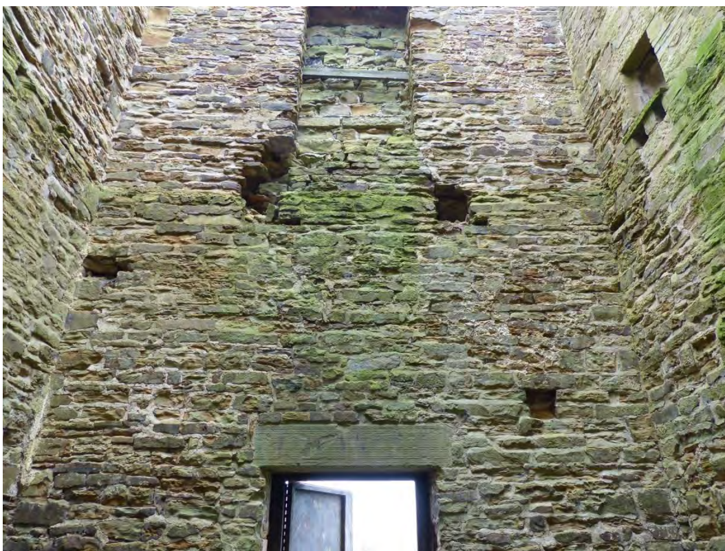
Plate 24: South interior wall, looking south
