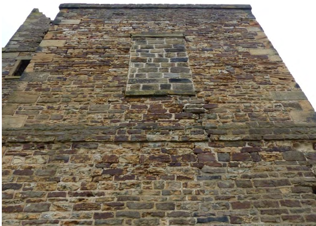
Plate 7: Detail of window to south elevation, looking north
