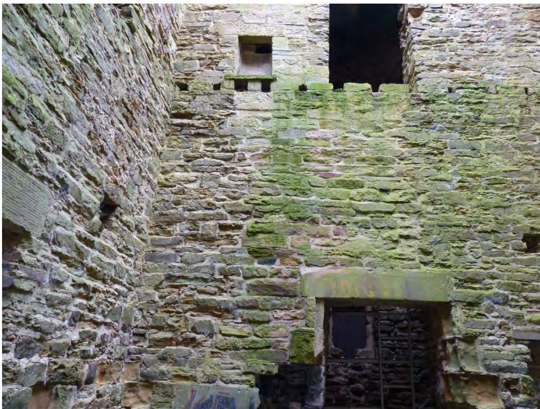
Plate 33: Middle portion of the west interior wall, looking west
