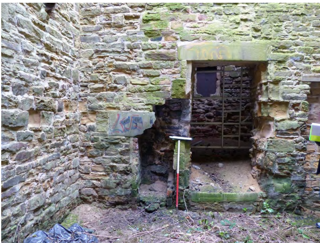
Plate 32: Lower portion of the west interior wall, looking west
