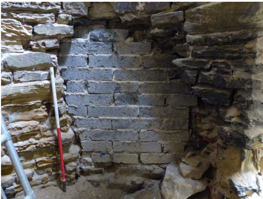
Plate 35: Blocked opening to the north of the stairwell, looking north
