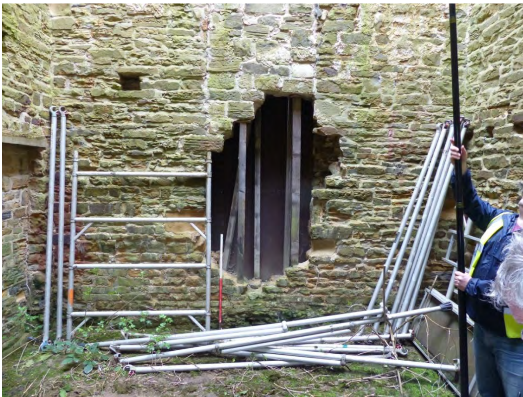
Plate 29: Lower portion of north wall interior, looking north
