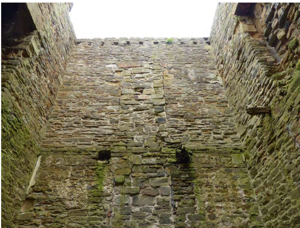
Plate 30: Upper portion of north wall interior, looking north
