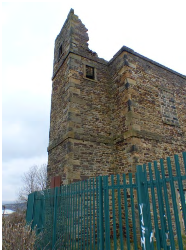
Plate 11: View of stair turret, looking north-east
