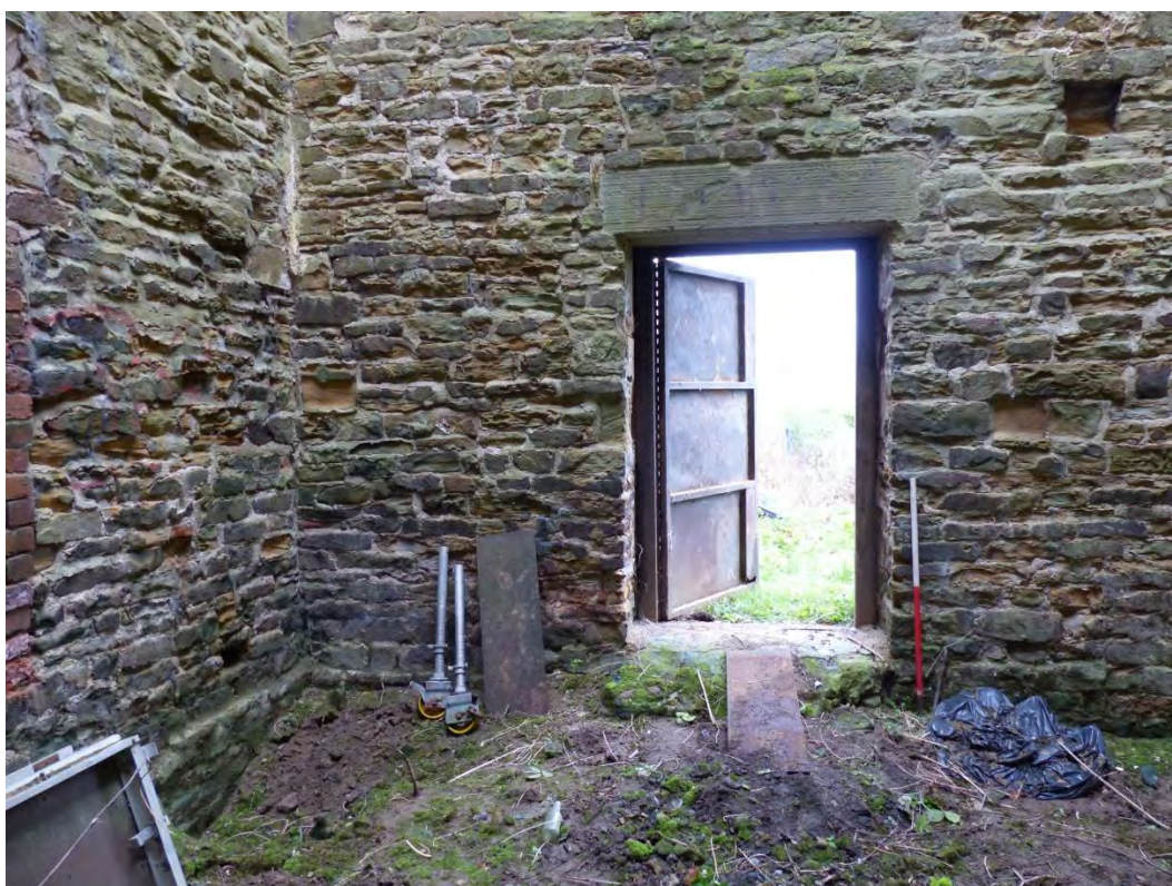
Plate 22: Door opening south interior wall, looking south
