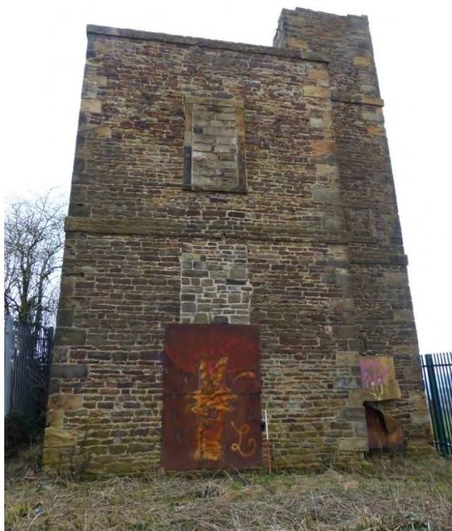
Plate 12: View of north elevation, looking south
