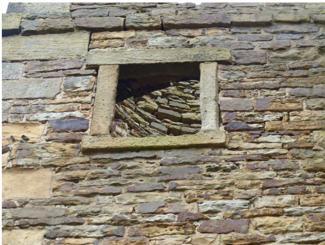
Plate 10: Detail of window to south elevation of stair turret, looking north
