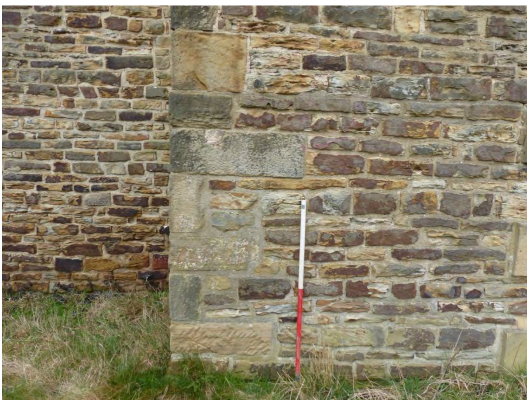
Plate 8: Detail view of quoins to south elevation, looking north
