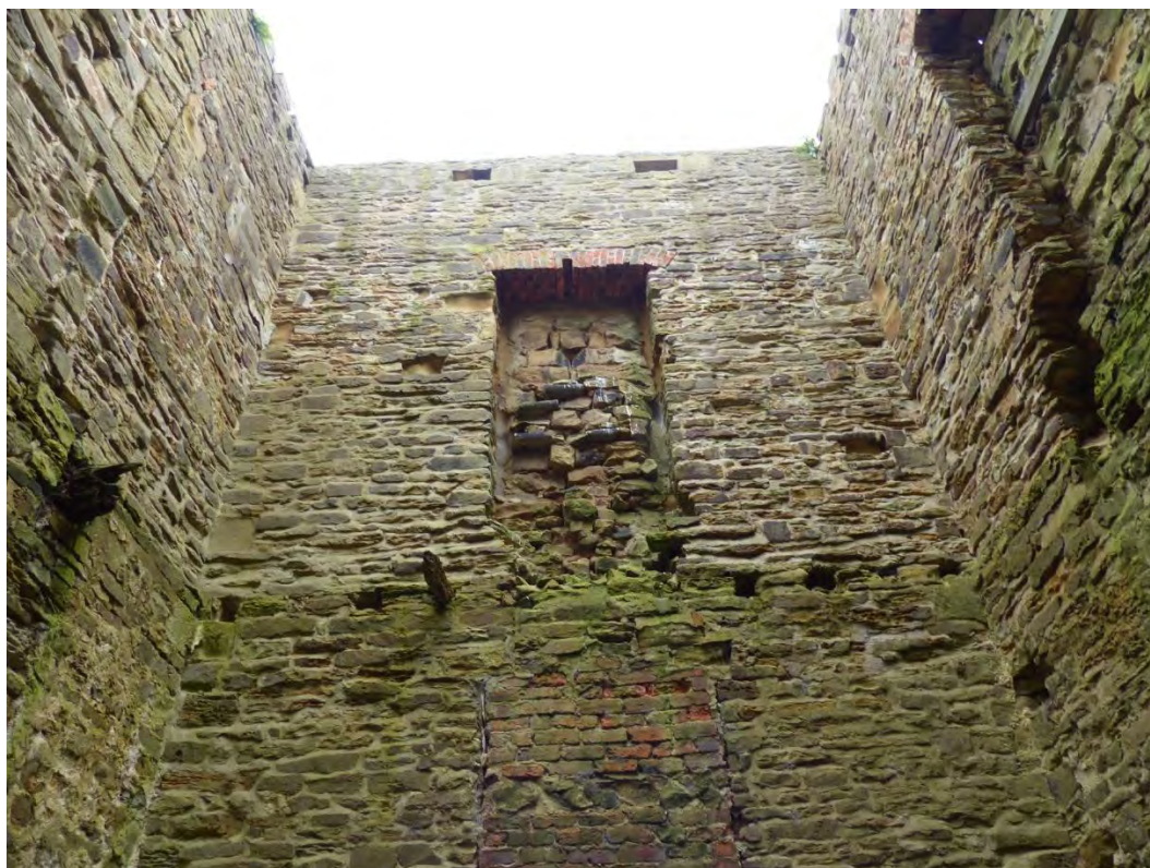
Plate 28: Upper portion of east wall interior, looking east
