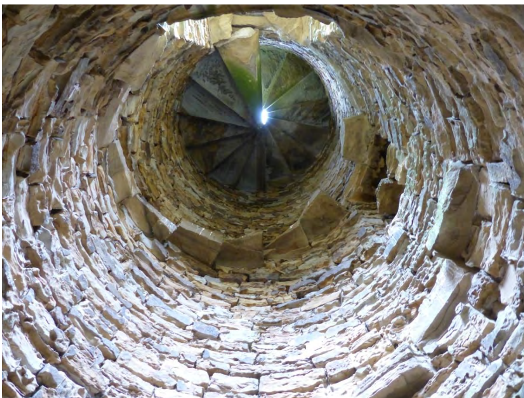
Plate 36: View up the stair tower showing support stones
