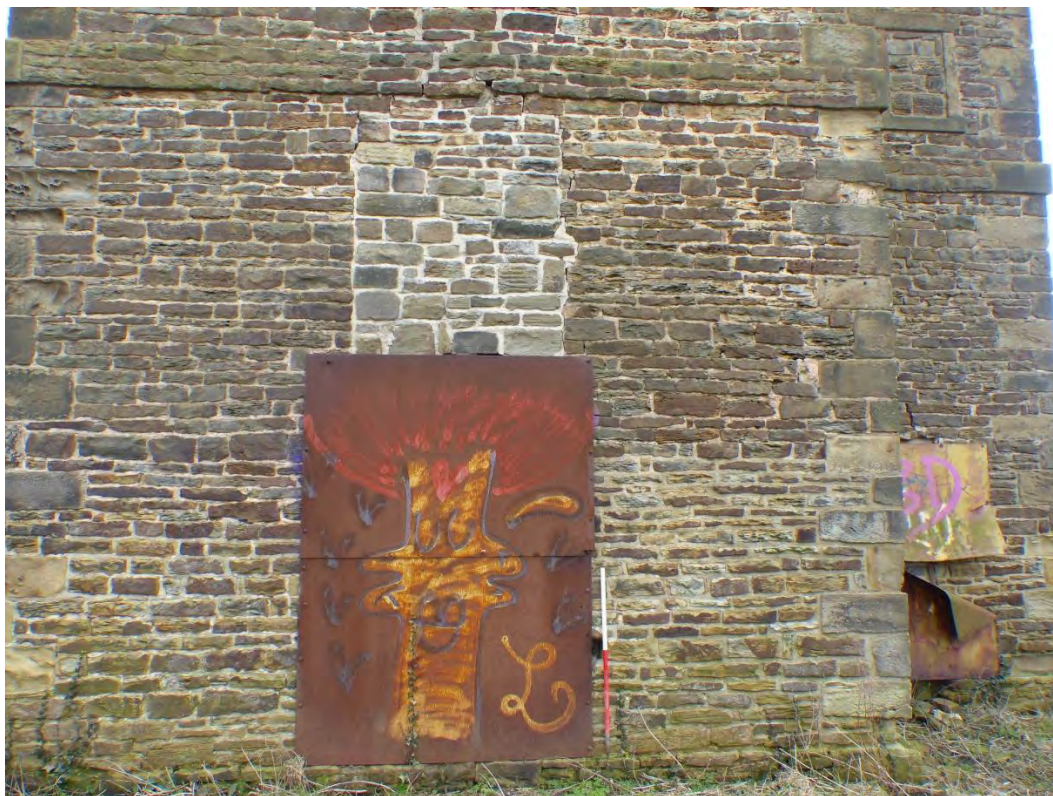
Plate 15: Detail view of blocked openings to north elevation, looking south
