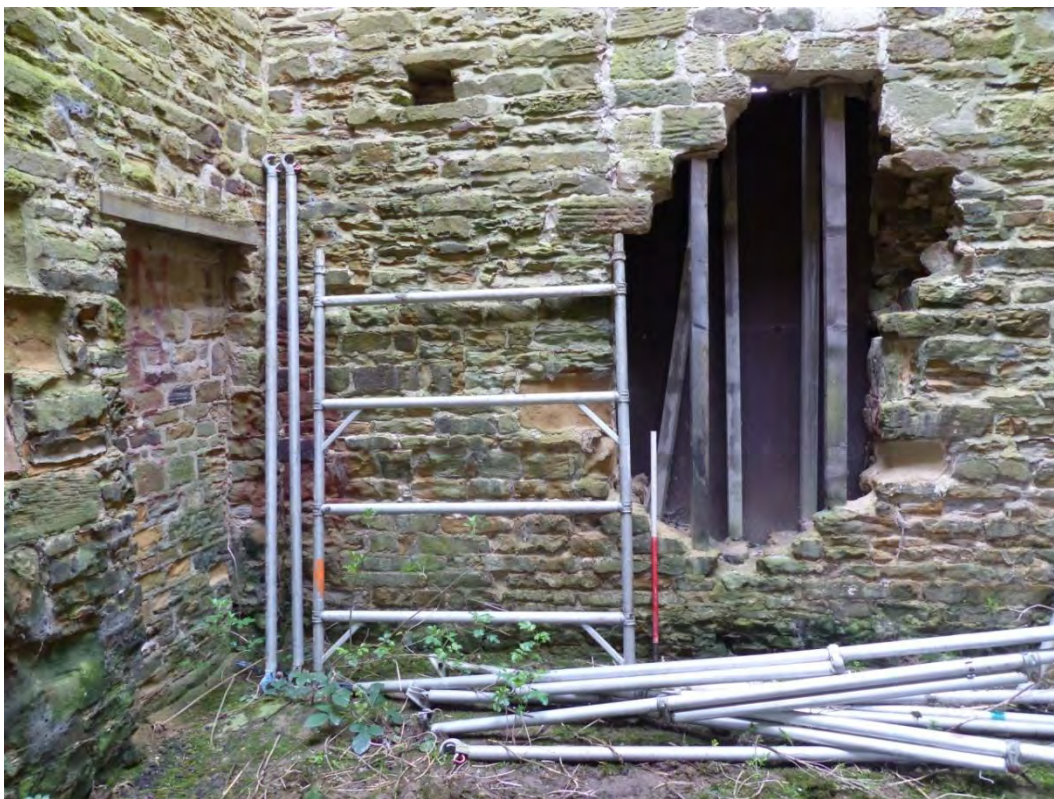
Plate 31: South-west corner of interior main building, looking west
