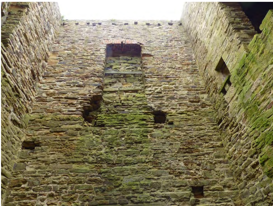
Plate 25: Upper portion of south wall interior, looking south
