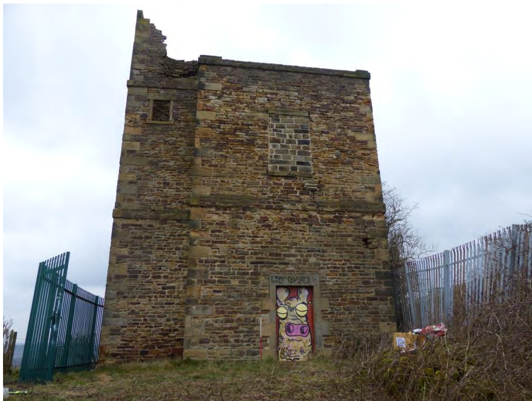
Plate 5: South elevation, looking north
