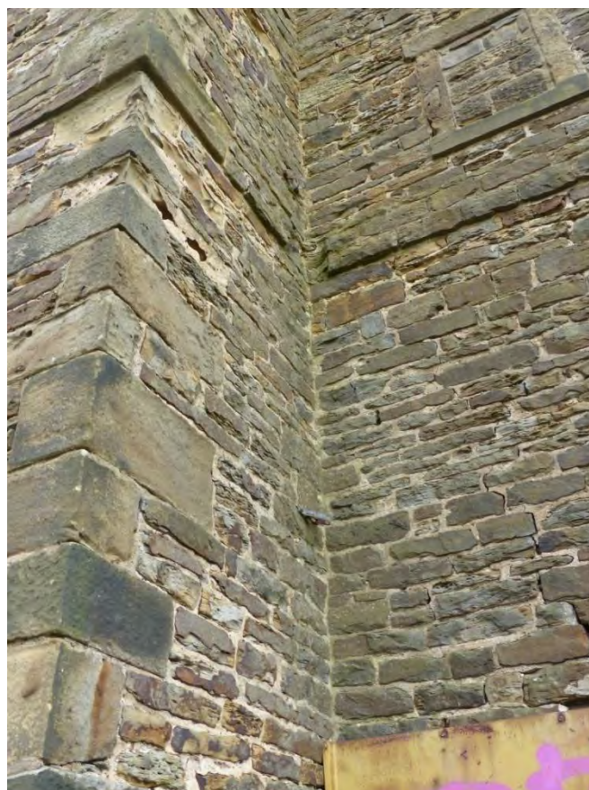
Plate 14: View of disused rainwater brackets to north elevation, looking south-east
