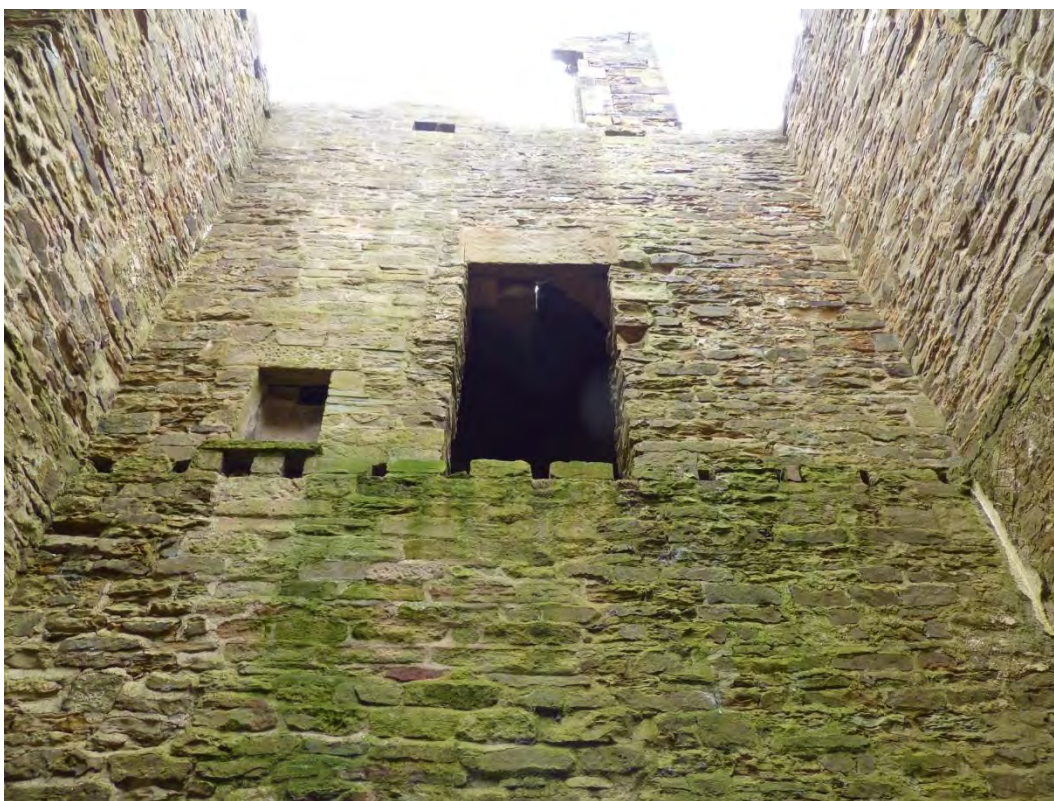
Plate 34: Upper portion of the west interior wall, looking west
