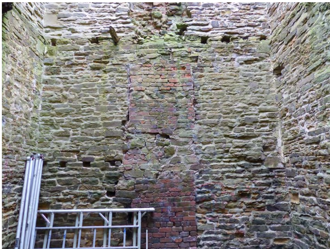
Plate 27: Middle portion of east wall interior, looking east
