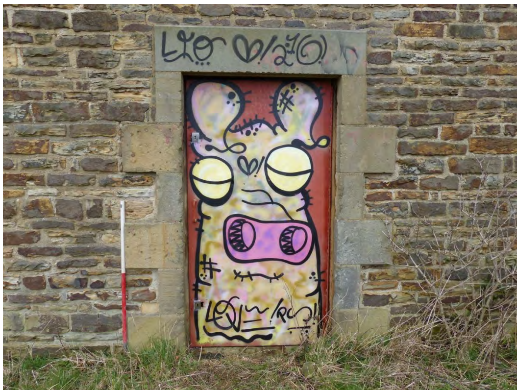
Plate 6: Detail of door on south elevation, looking north
