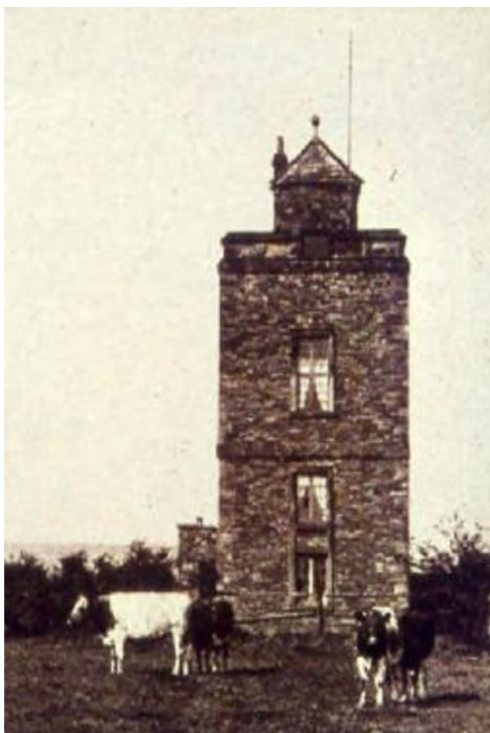
Plate 4: Late 19 th -century photograph of the east elevation, looking west
