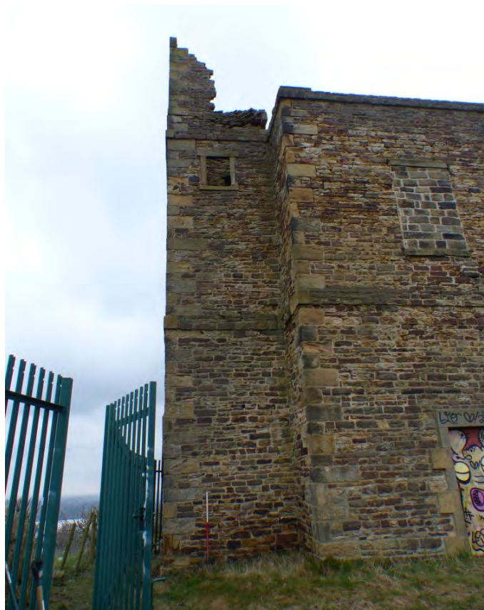
Plate 9: View of south elevation of the stair turret, looking north
