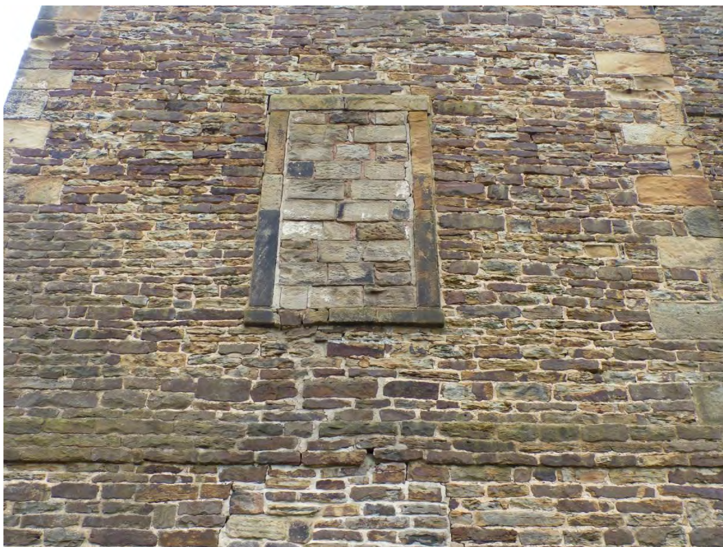
Plate 16: Detail view of blocked window opening to north elevation, looking south
