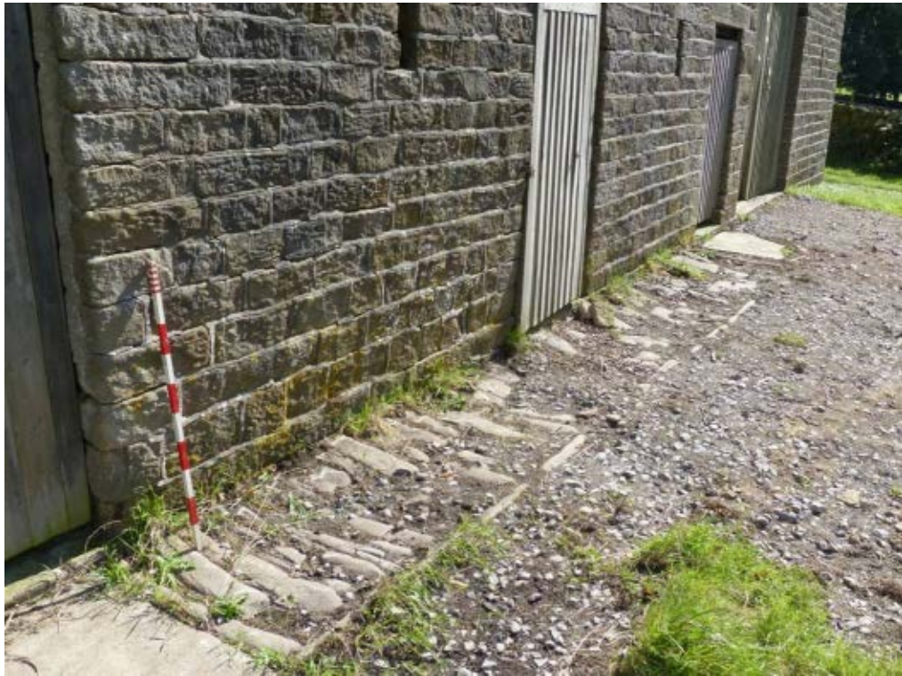
Plate 5: Central Paving setts in front of cow house entrance, facing south-east
