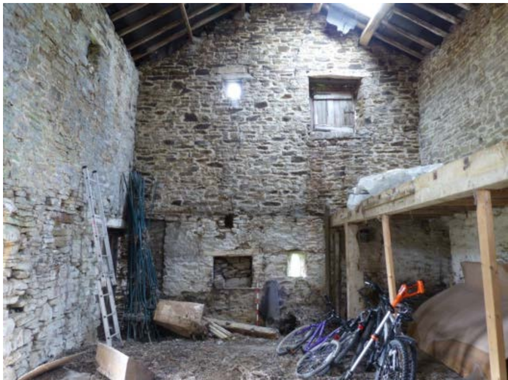
Plate 18: Interior of cow house, a blocked muck hole can be seen as well as the forking hole above, looking north
