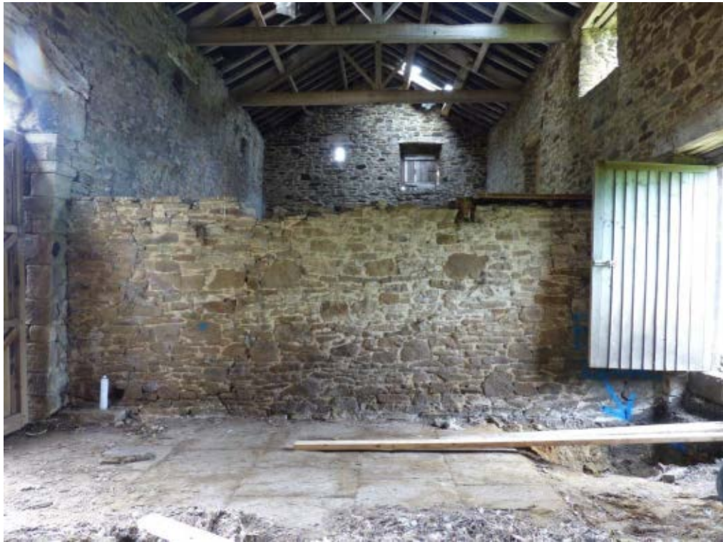
Plate 13: Flagstone threshing floor between the two barn doors, looking north
