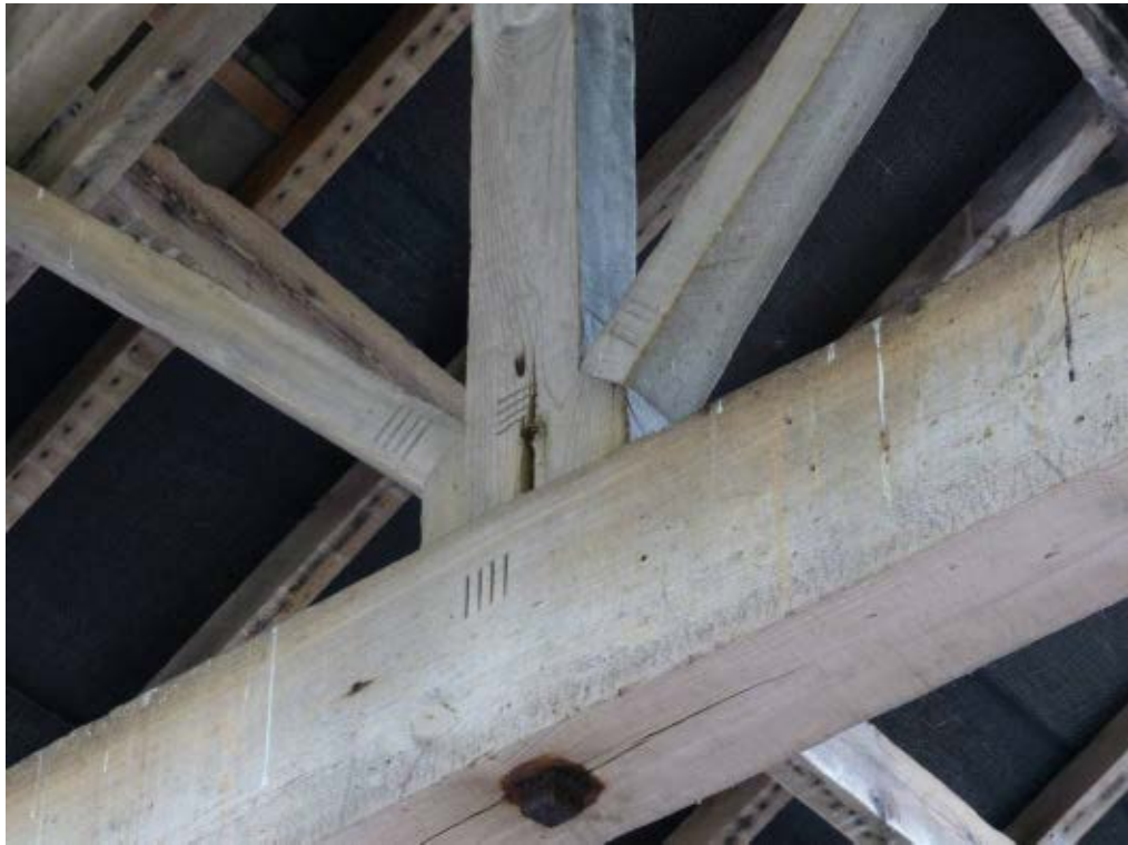
Plate 11: Carpenter's marks on truss III, facing north-west
