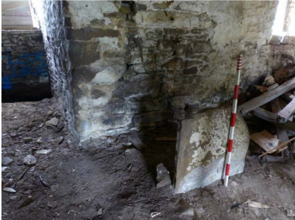
Plate 17: Interior of the cow house, in-situ slab divider, looking south-east
