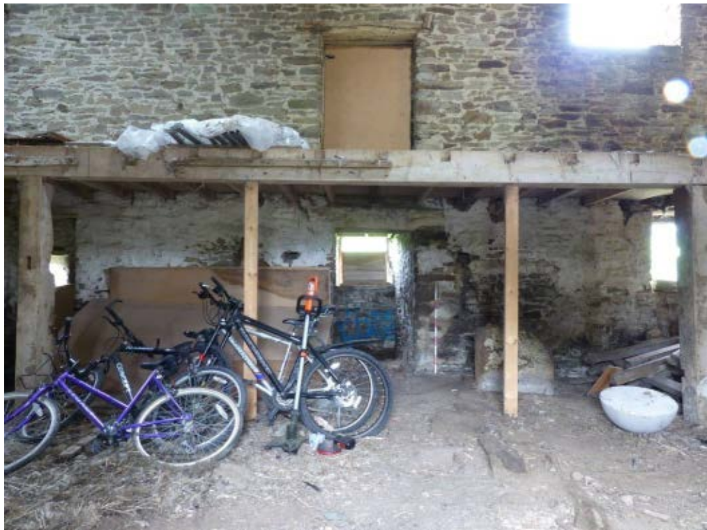
Plate 16: Interior of the cow house, the remains of a stone wall run from the bottom right of the photo, past an in-situ slab divider, looking east
