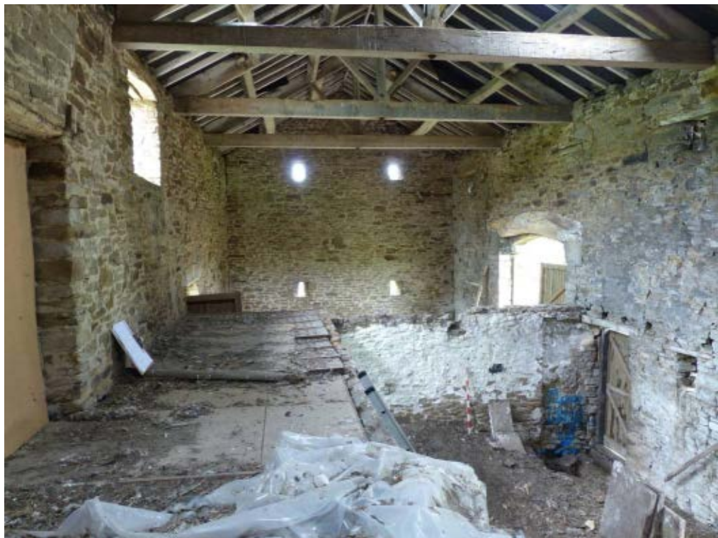
Plate 12: Interior of the barn, facing south
