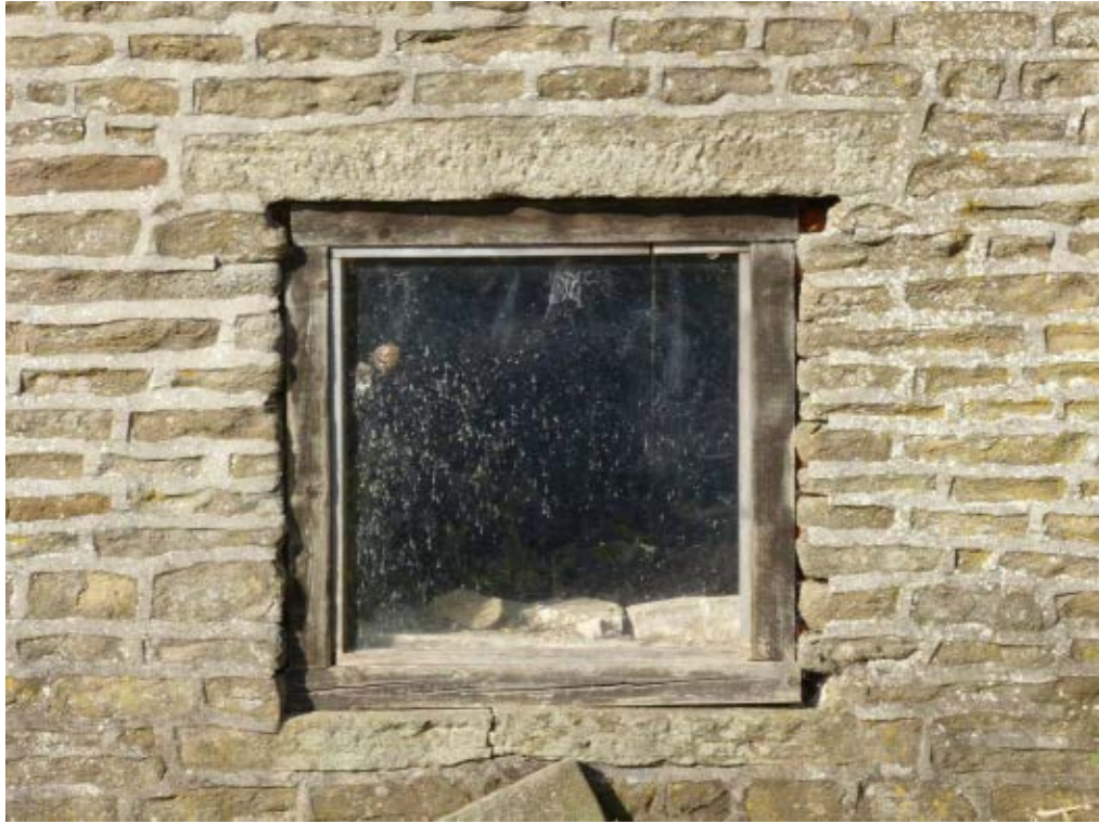
Plate 7: Muck hole in east wall of cow house with later glazing, facing west
