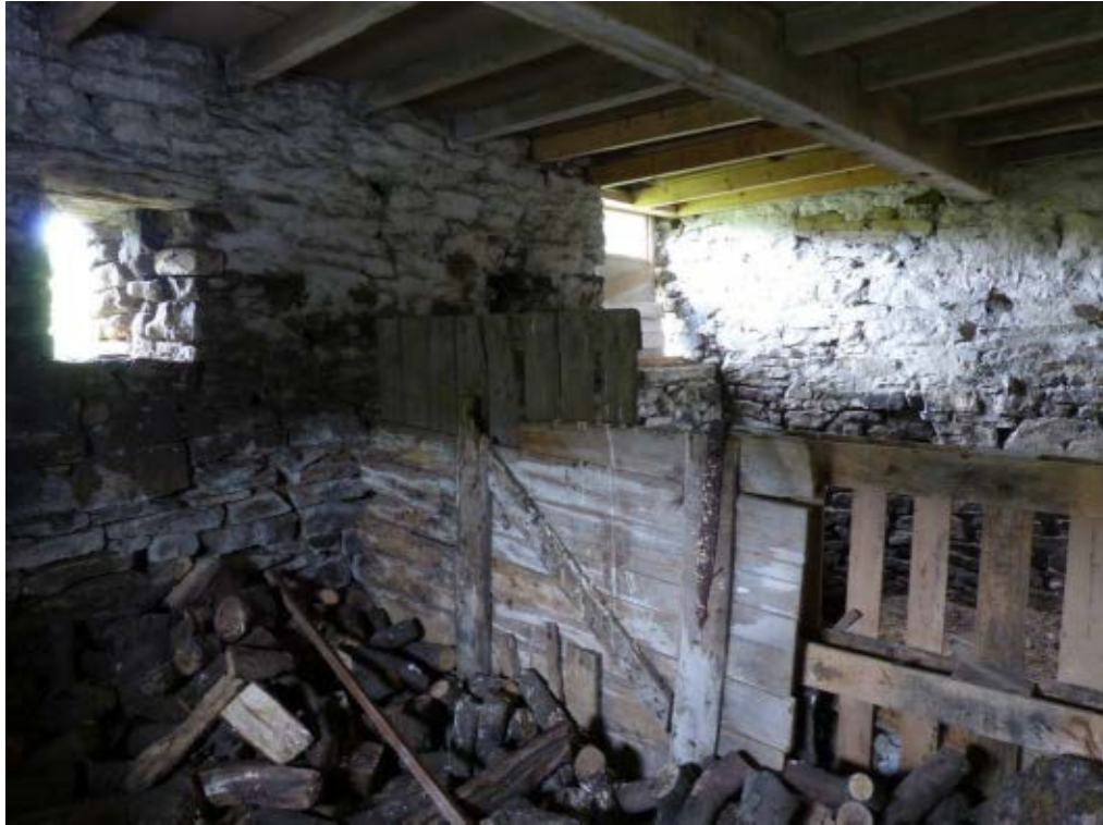
Plate 19: Ground floor of lean-to, facing south-east
