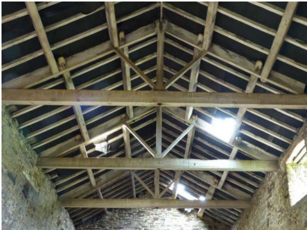
Plate 10: The roof, looking north
