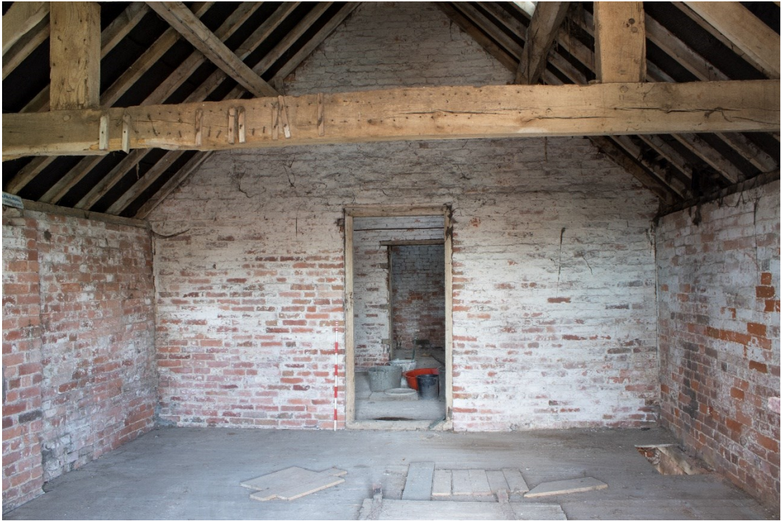
Plate 15: First floor east room, facing west (1840_046.TIF)
