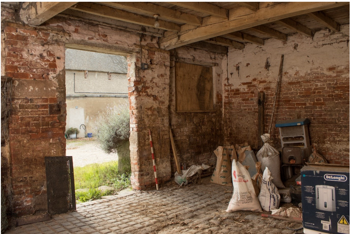
Plate 10: Ground floor east room in main range, facing south-west (1840_027.TIF)
