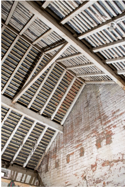
Plate 19: Roof in west range east room, facing north-east (1840_040.TIF)
