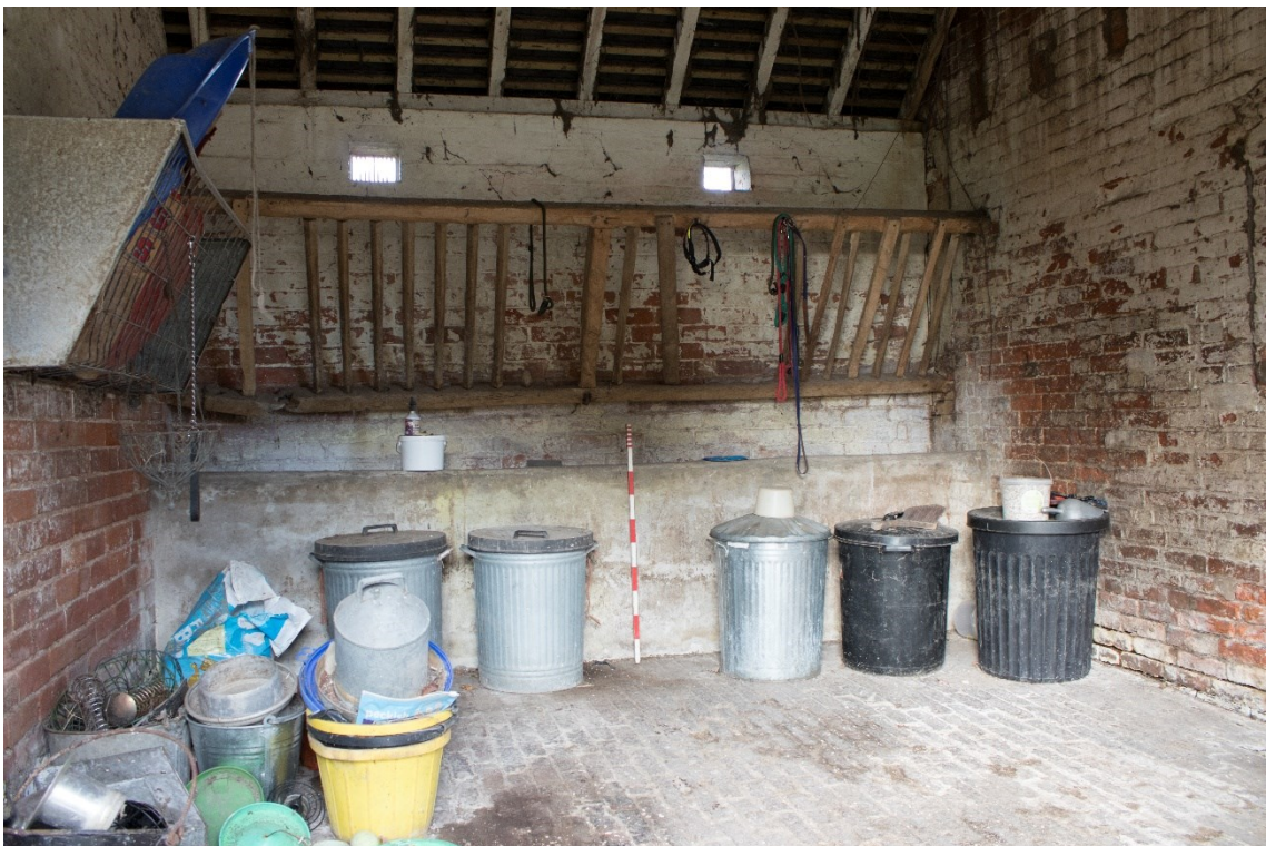
Plate 18: West range east room, facing north (1840_039.TIF)
