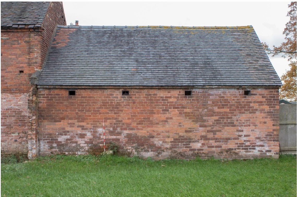
Plate 6: North elevation of the west range (1840_032.TIF)
