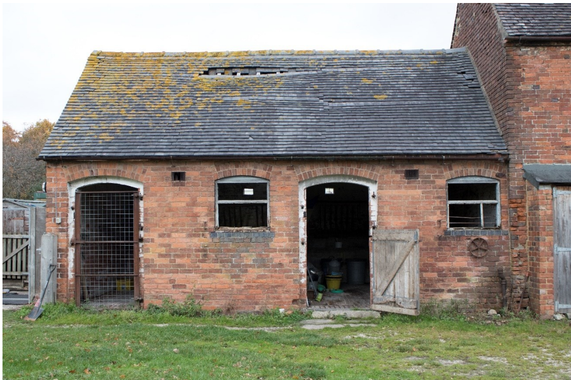
Plate 4: South elevation of the west range (1840_007.TIF)
