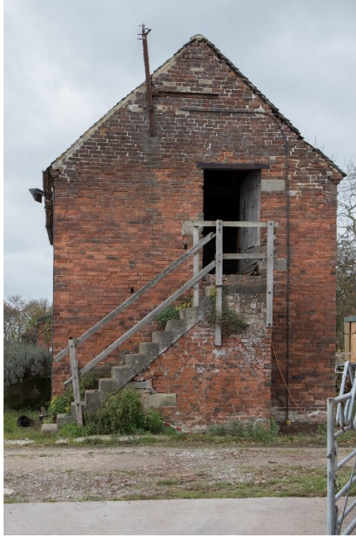
Plate 7: East elevation of the barn (1840_020.TIF)
