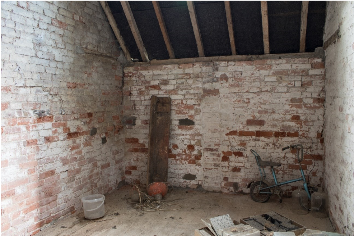
Plate 17: Straight joint in first floor west room, facing north (1840_055.TIF)
