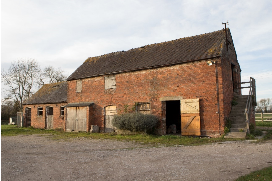
Plate 1: South elevation of the barn (1840_061.TIF)
