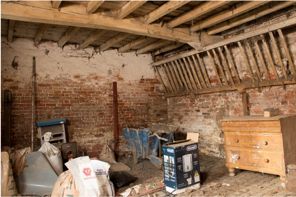
Plate 9: Ground floor east room in main range, facing north-west (1840_027.TIF)
