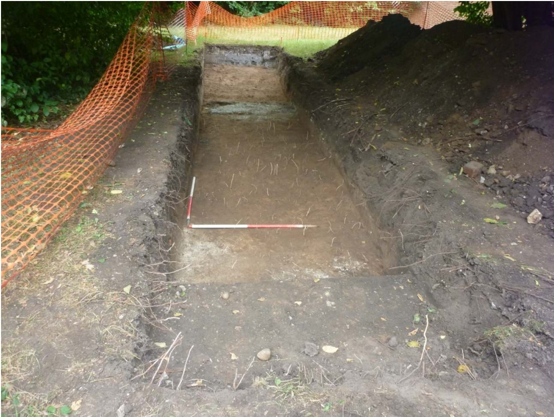
Plate 9: Trench 2, looking south-east. Scale 1m
