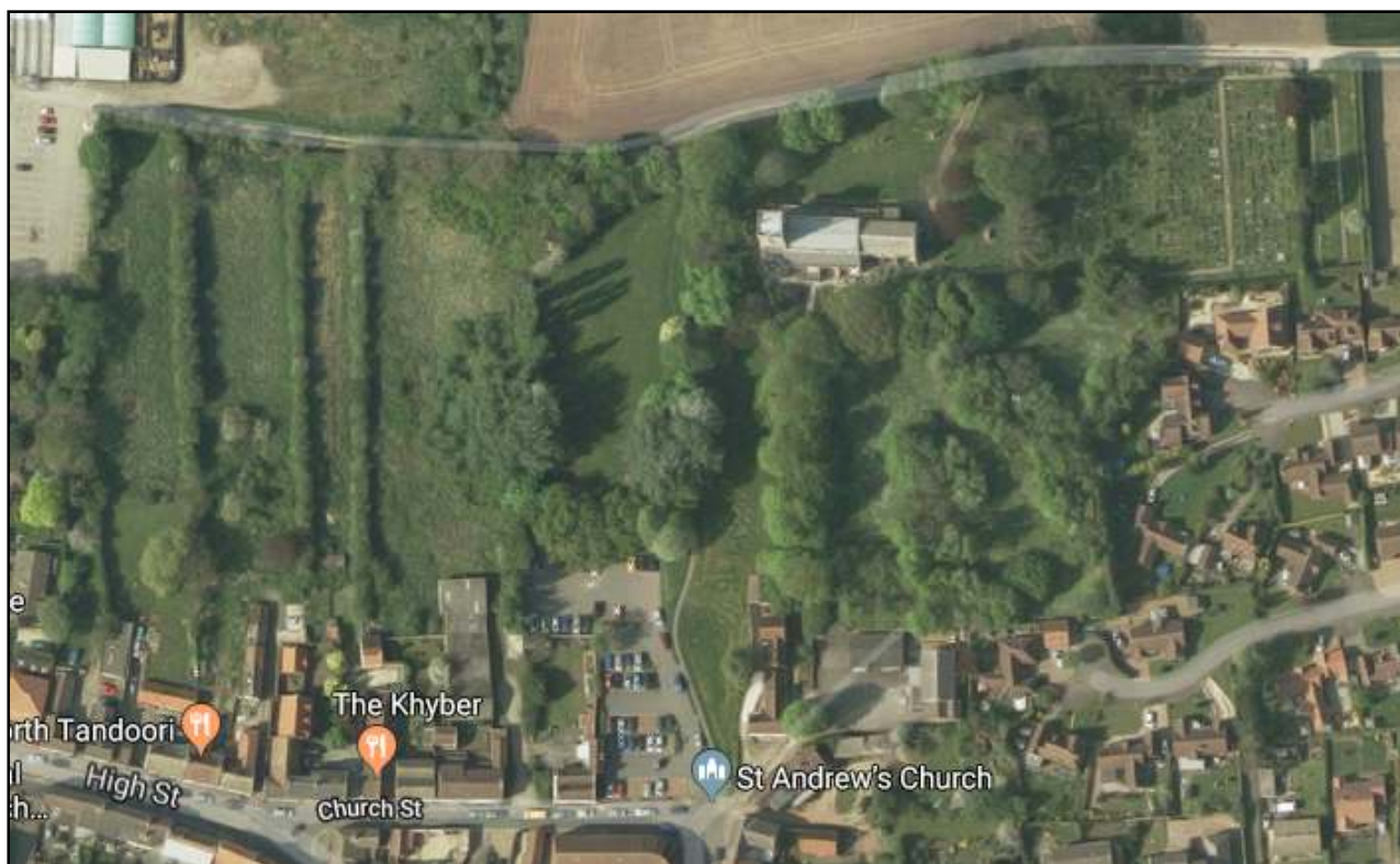
Figure 1: Google map image of the fields to the front of St Andrews Church and the burgage plots to the west (Not to scale.)
