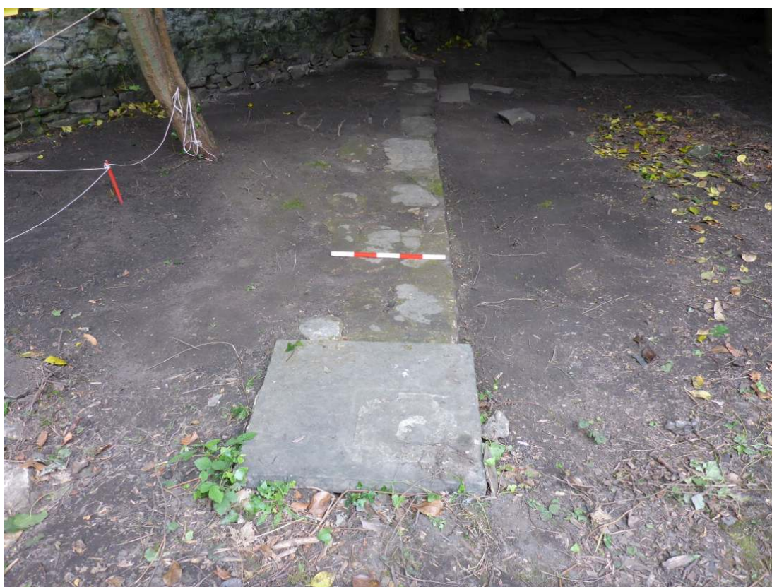
Plate 11: Eastern part of the pergola base (113) and surviving slab, viewed facing northeast
