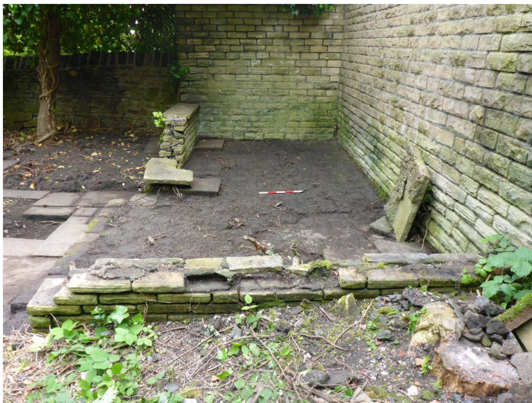
Plate 8: South-facing view of the loggia showing walls 107, slabs 108 and bedding layer 109
