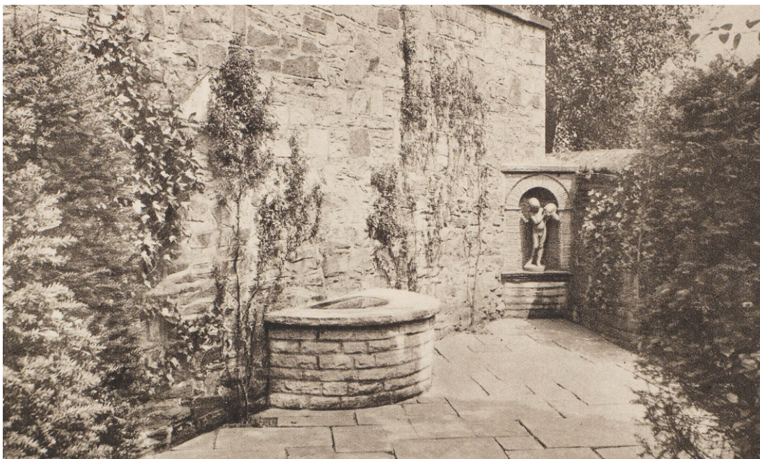
Plate 3: Detail of the dipping well and statue niche, 1931, viewed facing east
