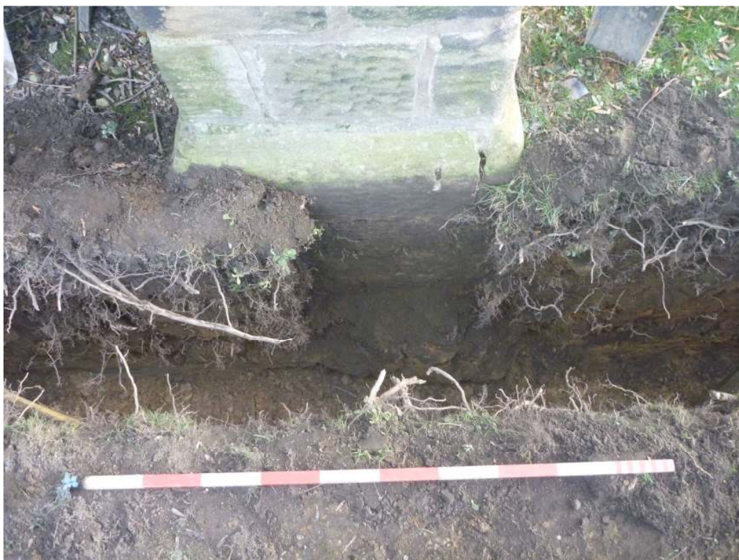
Plate 5: Structure 113 beneath south corner of the church tower, viewed facing northwest
