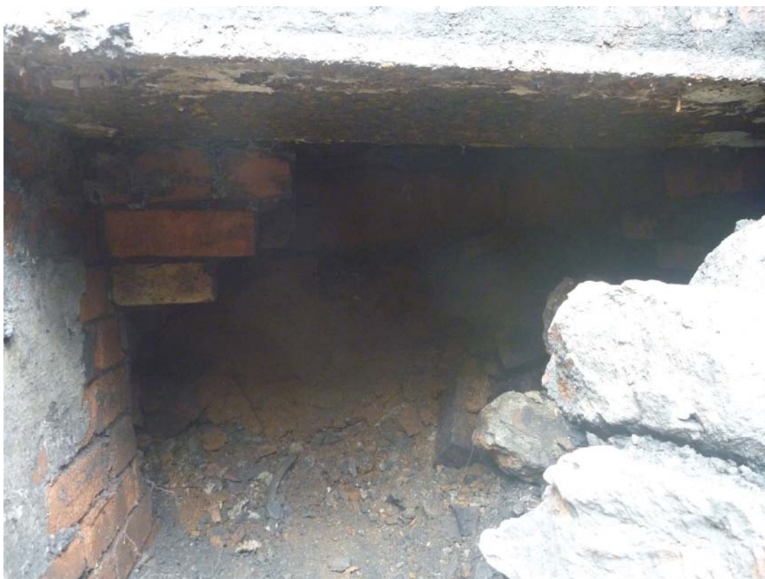
Plate 6: Detail of interior of southern stoking hole, wall 126, showing stepped bricks and infill
