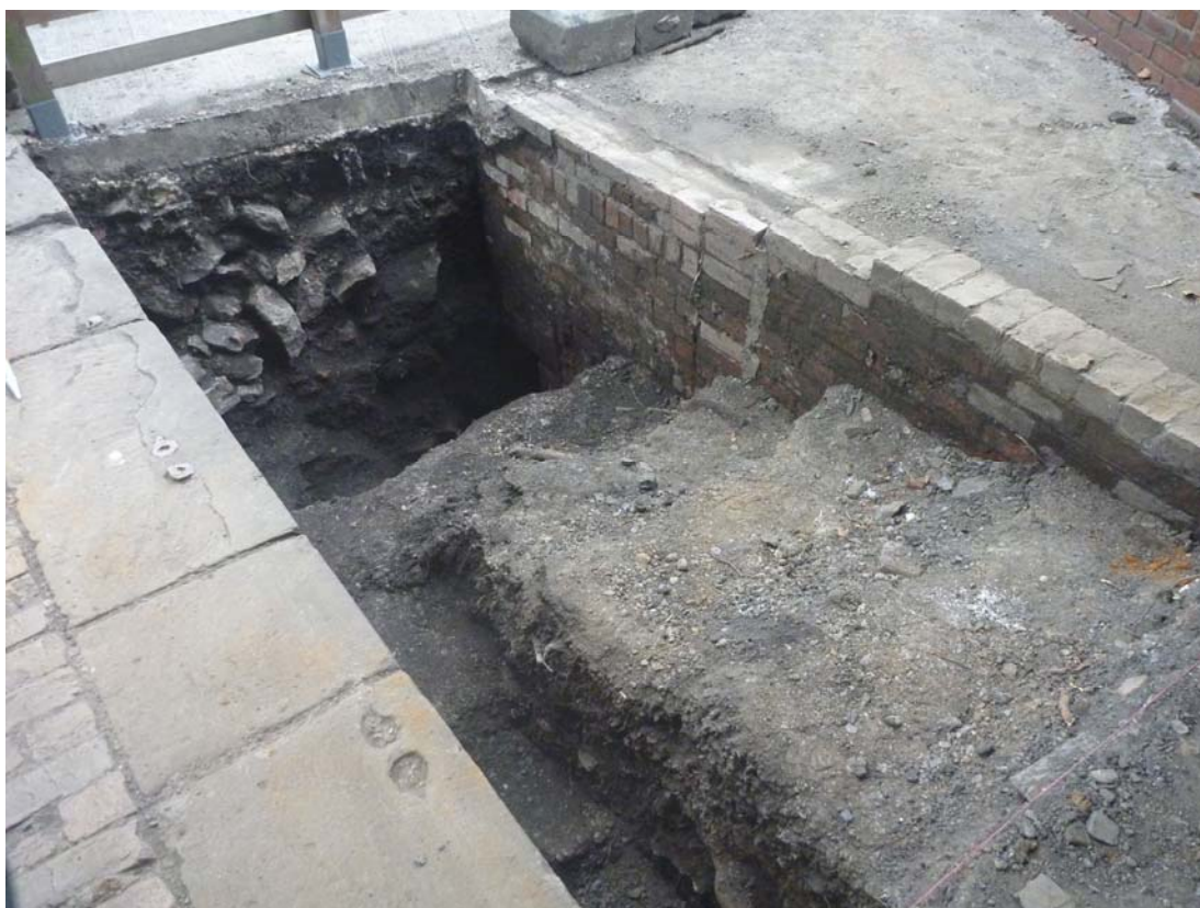
Plate 7: Trench 1, showing western wall 112/127/128, viewed facing southwest
