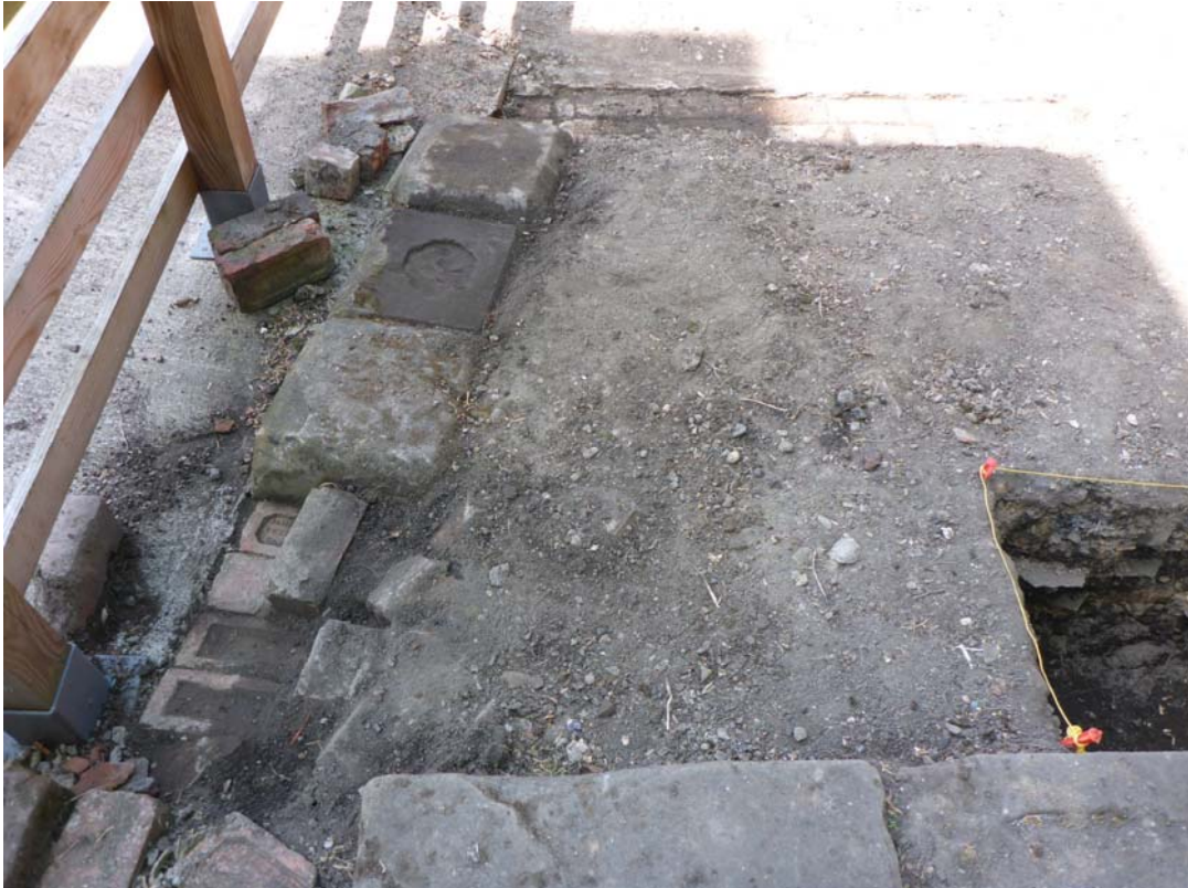
Plate 4: Possible re-used padstones (structure 113), viewed facing west
