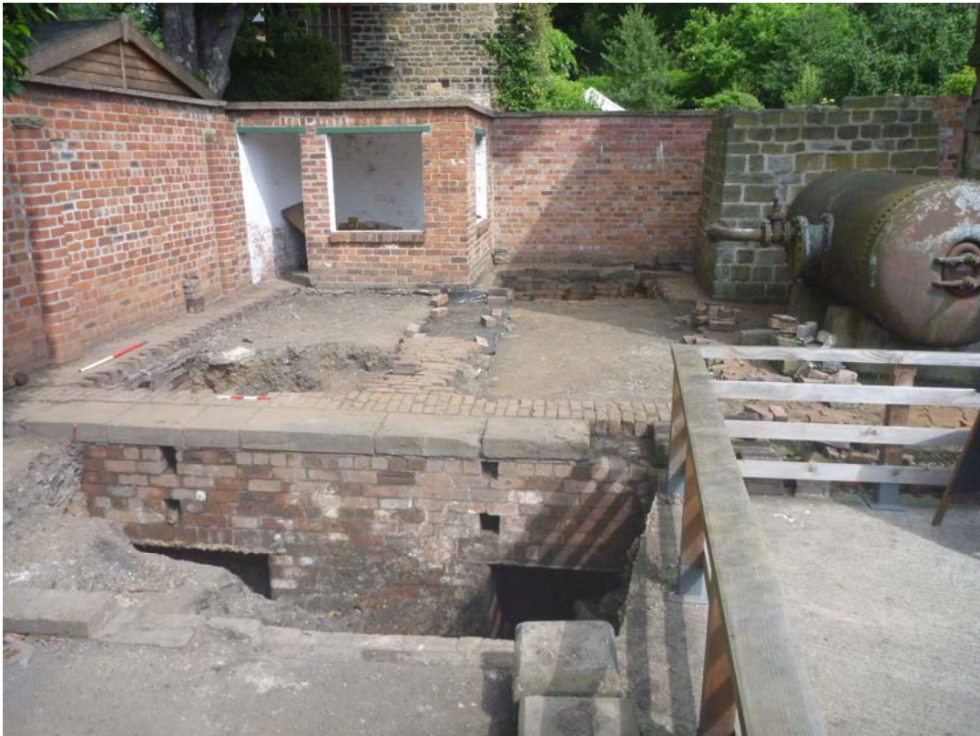
Plate 3: View east across site, Trench 1 in foreground
