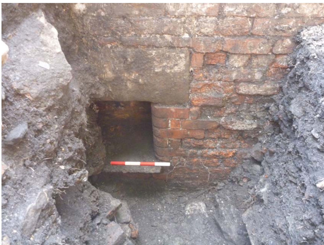
Plate 8: Detail of coal chute in wall 128, viewed facing west (scale in 10cm increments)
