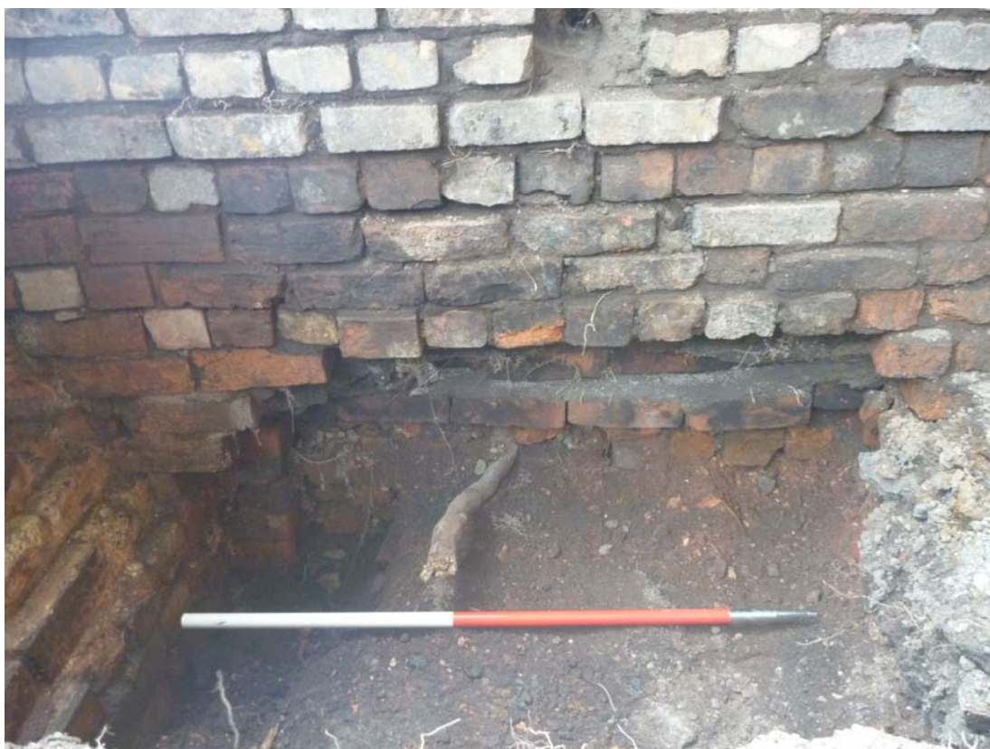
Plate 10: Detail of top of stoking hole in wall 123, viewed facing west
