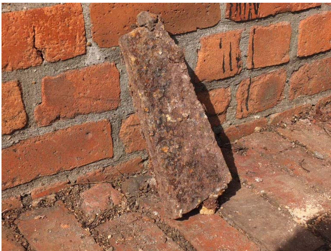
Plate 9: Possible fragment of cast iron lintel from context 102
