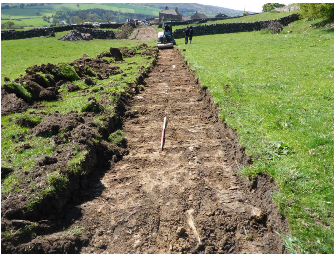
Plate 2: Stripping of half of the easement in Field 4, viewed facing west
