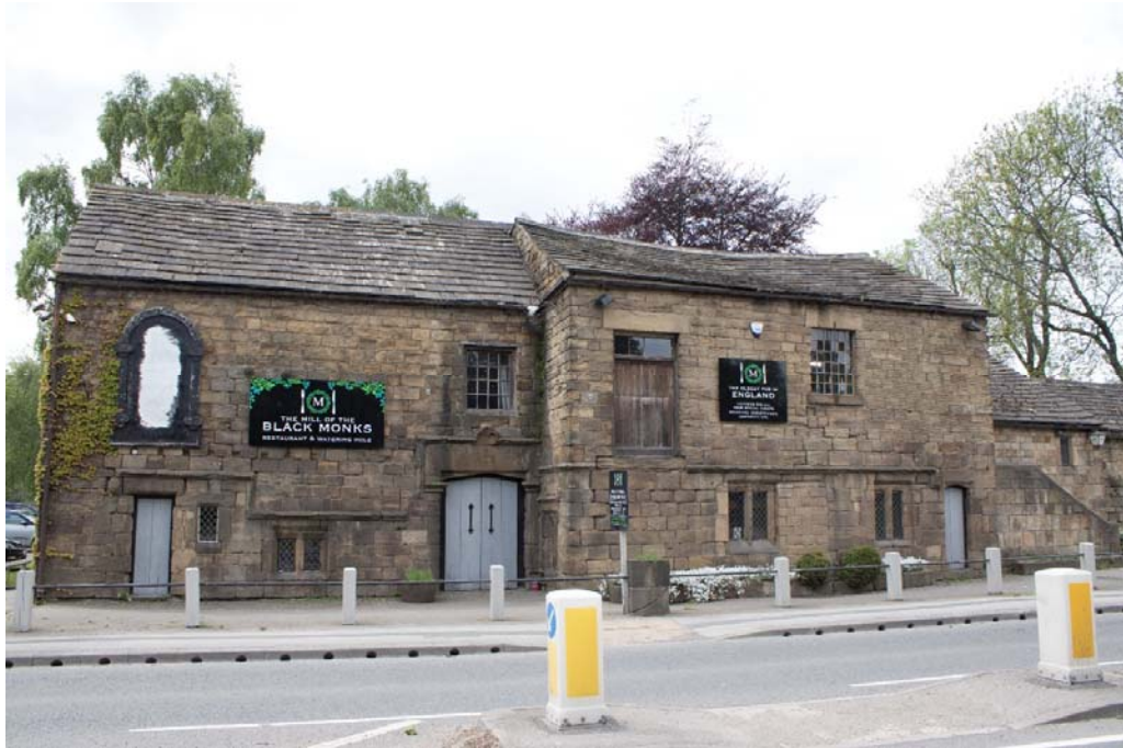
Plate 1: East elevation of the Mill of the Black Monks
