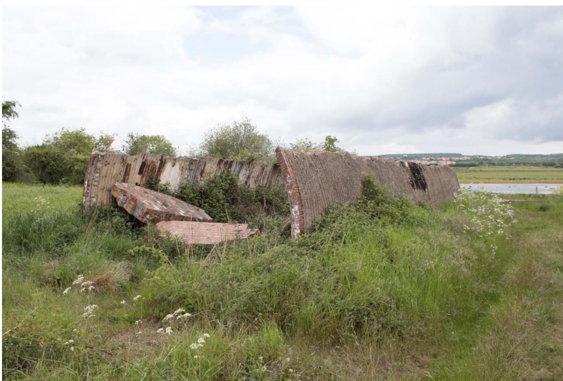
Plate 6: Nissen hut at the north of the site, facing north
