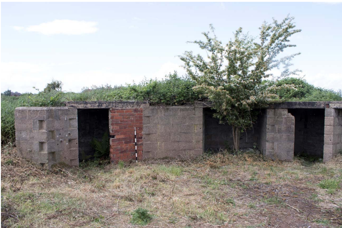
Plate 4: Interior of gun emplacement B, facing north-west
